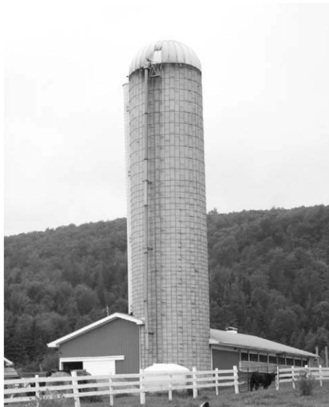
FIGURE 8.5 Typical grain silo for storing cattle feed. (Source: Photograph by the author.)
