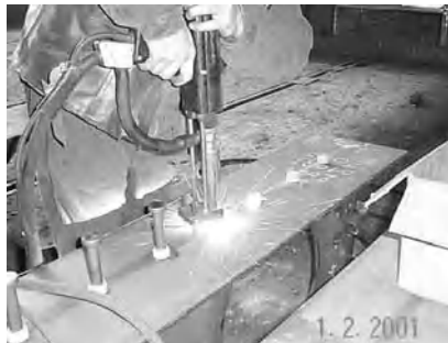
Figure 10.5. Stud welding: welding of connectors – photograph from Baudin-Châteauneuf
