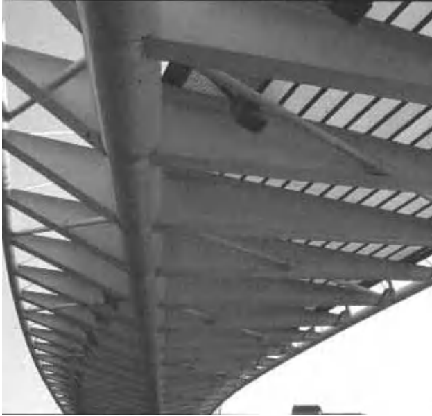
Figure 10.1. Footbridge in Bilbao – Santiago Calatrava Architect – photograph from CTICM
