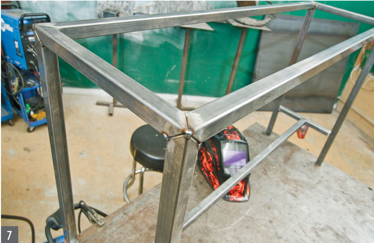
Tack the entire piece together before welding.
