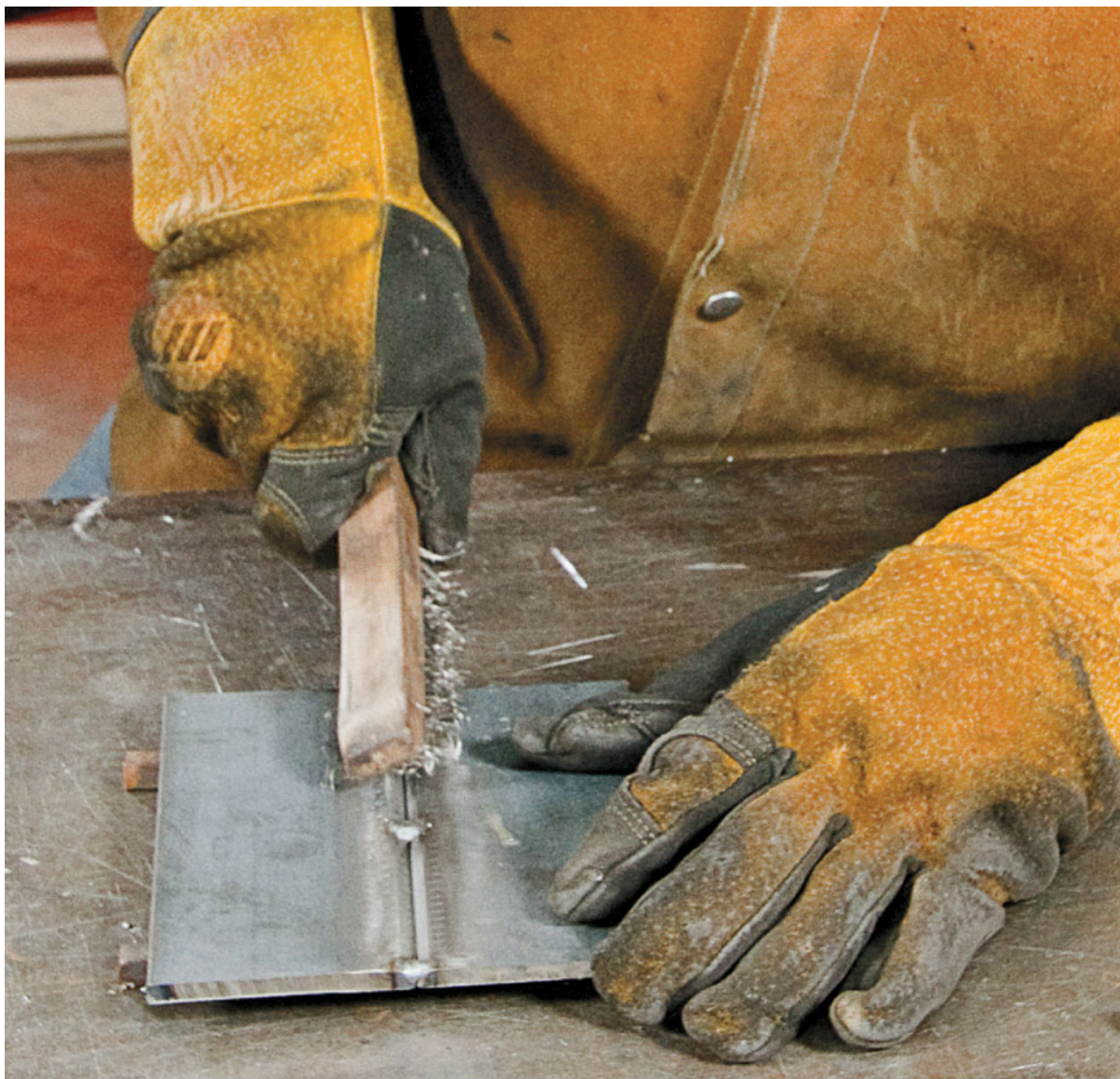
Clean the metal after each weld and series of tacks.
