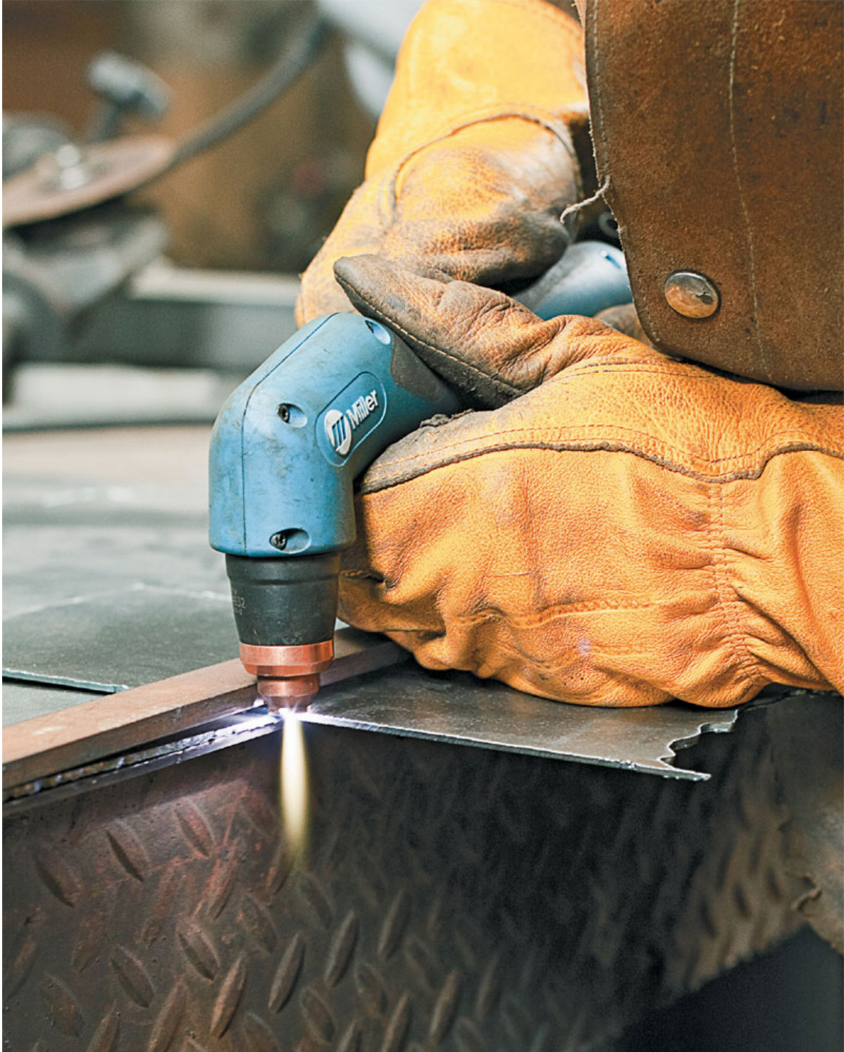
Note how I am cutting with a guide for a straight cut and am using a drag shield (the detachable tip on the plasma gun) in order to make contact with the base metal and my guide.
