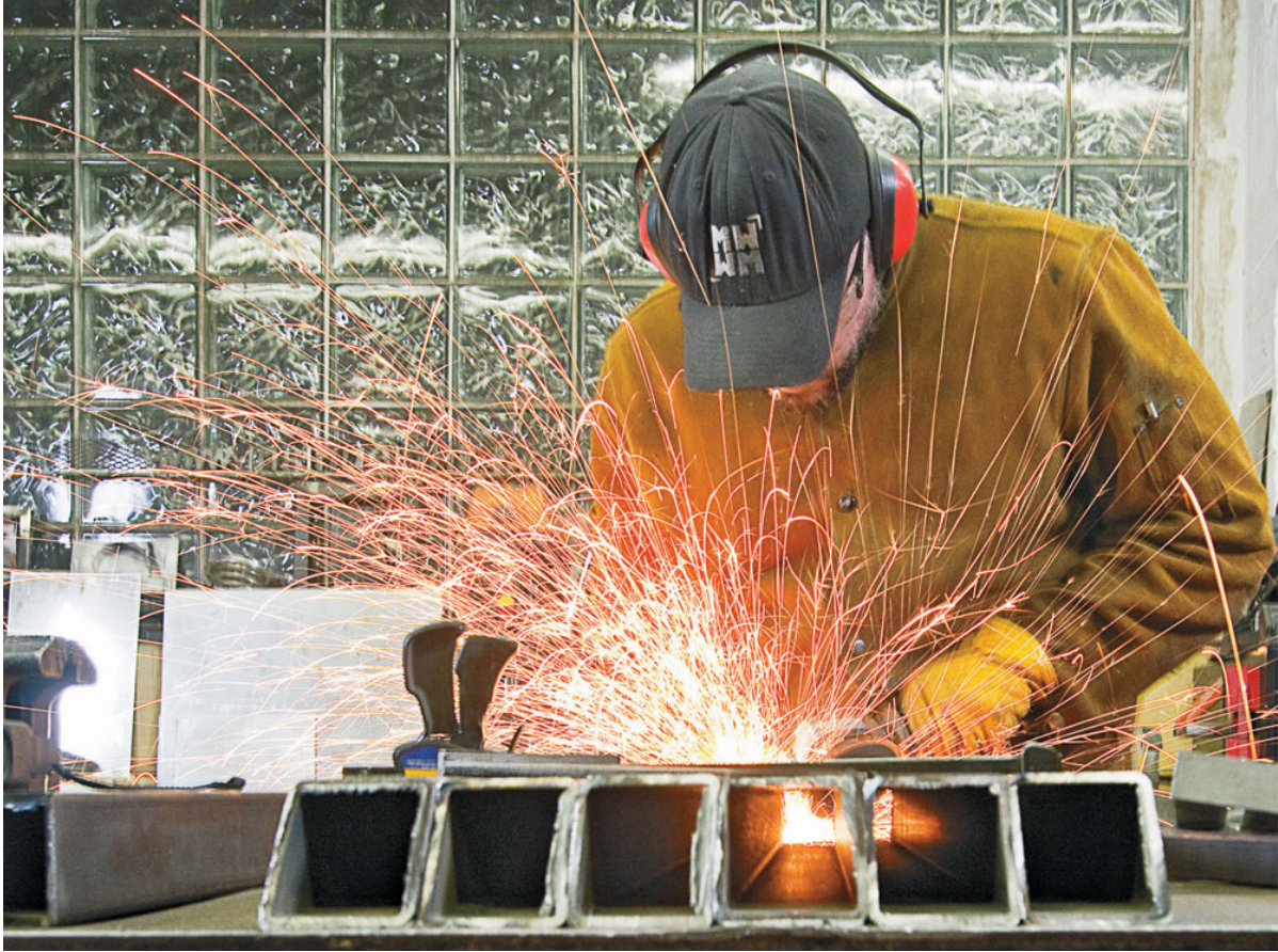
It may be necessary to use a grinder to even out some cuts that may be a little off before you can prep the steel for welding.
