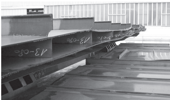
23.1 Typical arc welded deck panels for a passenger ship; note the distortions.
