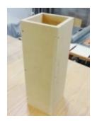
Step 2: The form's base was made using pieces of framing lumber that was 3 1/2" wide. These pieces needed a bevel cut so they would angle upward to the top of the form tube.
