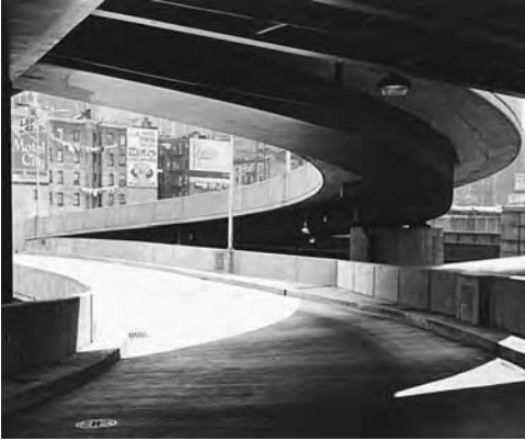
Fig. 14 Smooth, clean lines, without outside stiffeners carry a ramp on a sharp radius curve.
