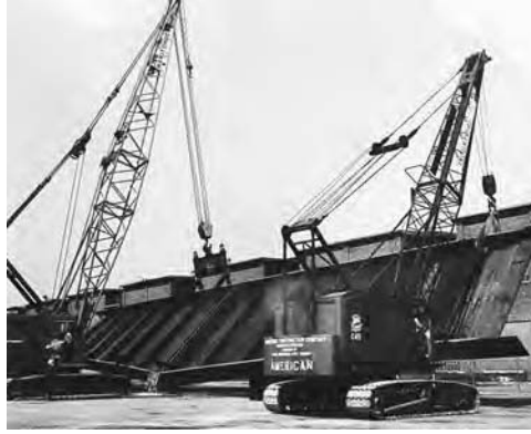
Fig. 15 Giant bridge girders fabricated by Allied Structural Steel for the Mississippi River crossing between Dresbach, Minnesota, and Onalaska, Wisconsin.
