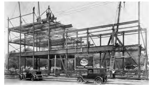
Fig. 7 This building was erected in 1928 using arc welding and bare-wire electrodes.
