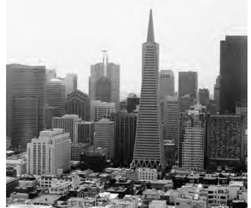
Fig. 16 San Francisco skyline showing a building with welded steel frames.
