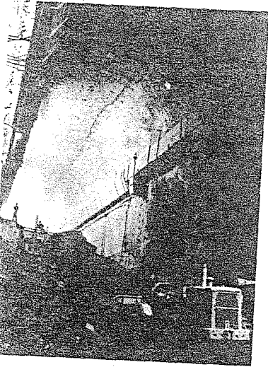
Figure 168 : Temporary construction entry mounted on anchored crane rails used to gain access to the roof of upper sidewalls of the cavern for initial rockbolt tensioning and shotcrete application.
