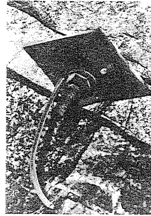
Installation of a rockbolt washer across the "sawtooth" profile of a blocky rock face makes subsequent sealing of the hole difficult.
