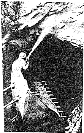
Success of a shotcrete operation depends very heavily upon skill of the nozzleman.
