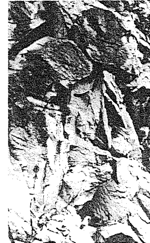
The sad remains of what could have been a perfectly safe and stable rock face.
