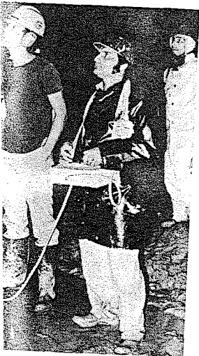
Figure 182 : Remote control box for shotcrete placement using a robot machine. The nozzle position is controlled by means of the two small "joysticks" on the control box.
