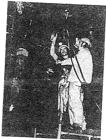
Figure 153 : Grouting a stressed 20m long high tensile steel cable in a stope back at the New Broken Hill Consolidated Ltd. mine.
