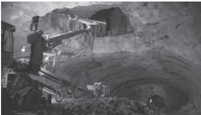
Figure 13. There is often little rock cover between new and existing tunnels.
