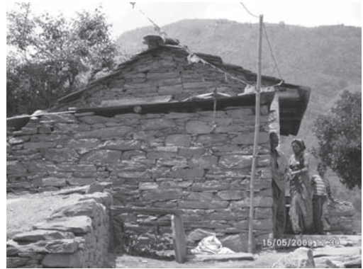
Figure 1. A house built using stone blocks & clay in study area.
