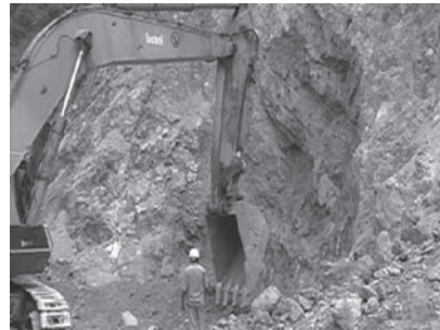
Figure 7. Tunnel portal excavation by excavator.
