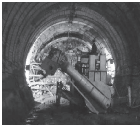
Figure 5. Casagrande PG 175 drilling rig at work.
