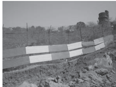
Figure 1. Barricade for preventing flyrock for railway track & traction.
