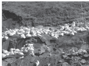
Figure 2. Arrangement of muffling for control of flyrock.
