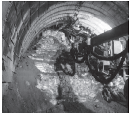
Figure 3. Forepoling with 36 mm steel rod using Boomer.
