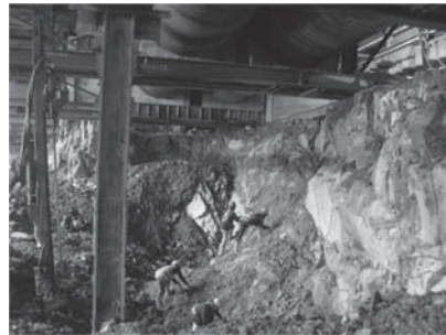
Figure 12. The twin water pipes just above the blasting area.
