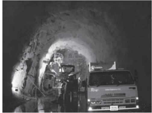
Figure 4. UG Bulk charging unit of Orica Mining Services at the face.
