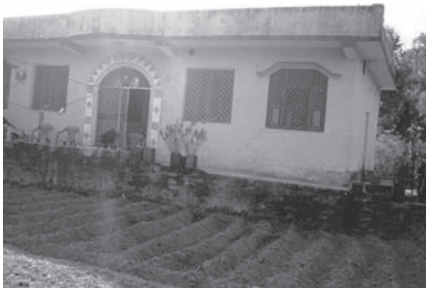
Figure 2. A house surrounded by the cultivation land without appropriate foundation works.
