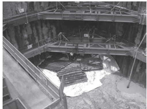
Figure 7. Overburden, geotextile and rubber mats as additional measures for fly rock prevention.
