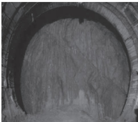
Figure 6. Full face of modified horse shoe shape.
