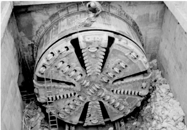
Figure 6.2 Shield machine receiving.
