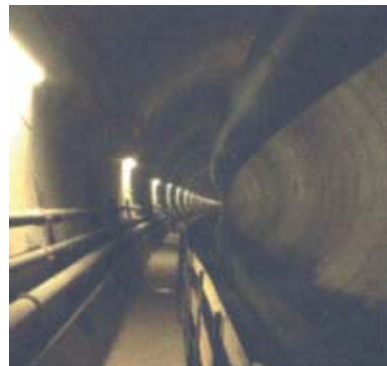
Figure ap.7.10.4 A picture of the tunnel.
