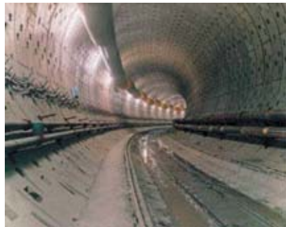
Figure ap.7.7.2 The excavated tunnel.
