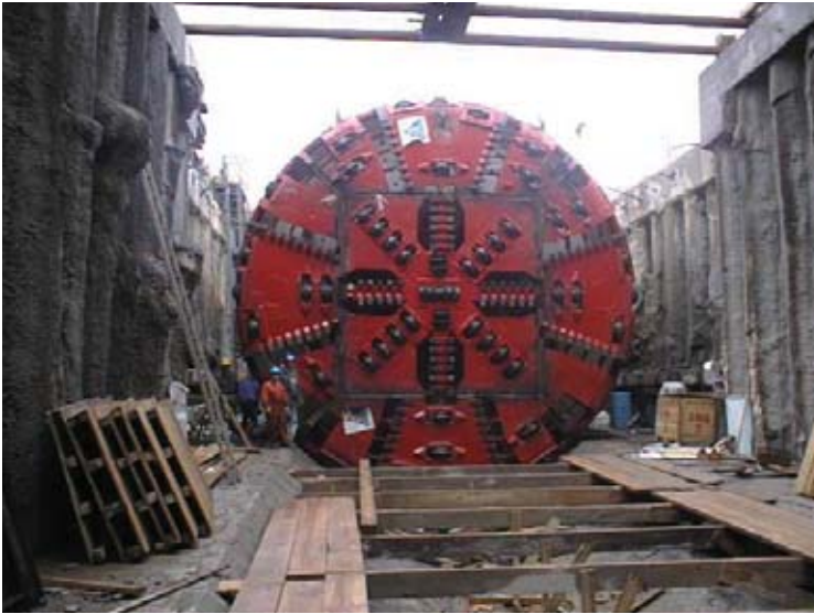
Figure 8.21 The cutterhead of the first Herrenknecht TBM in Porto.
