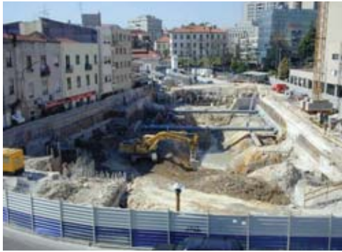
Figure 8.19 An example of open excavation for station construction.
