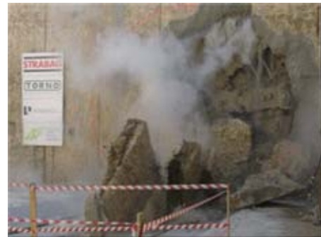
Figure ap.7.12.1 The TBM for excavating the Castellanza tunnel.
