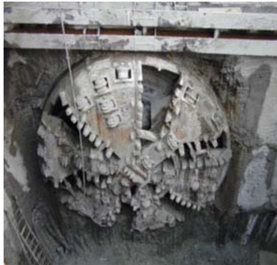
Figure ap.7.8.5 The TBM cutterhead.
