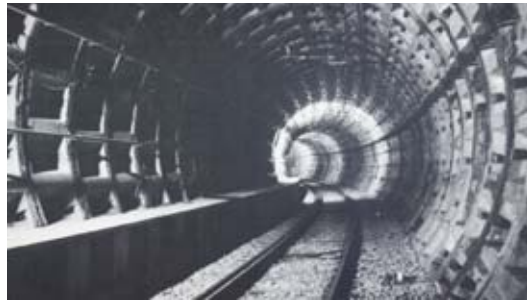
Figure ap.7.1.3 A picture of the tunnel.
