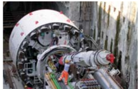
Figure ap.7.11.1 The TBM for excavating the Naples Line I.
