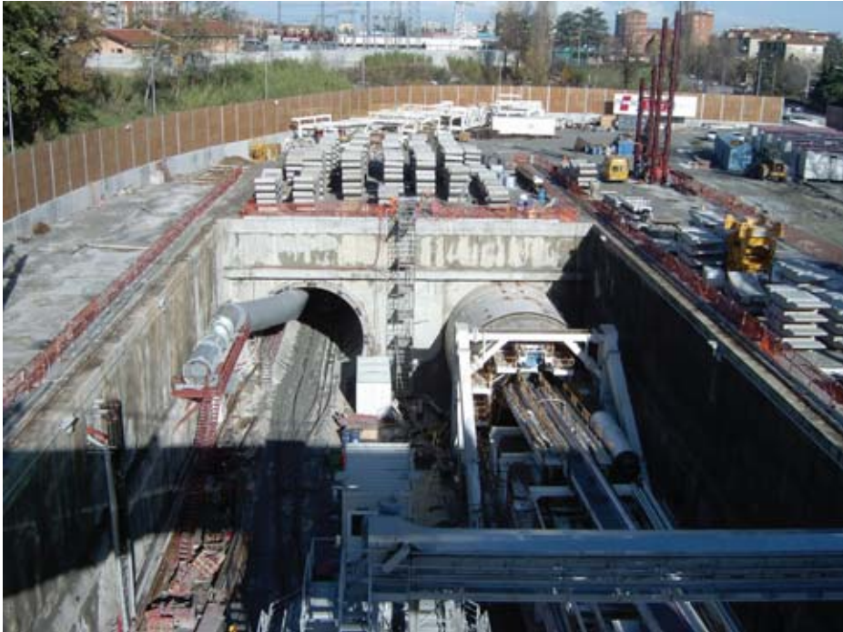
Figure 8.55 The second Lovat TBM ready to start.
