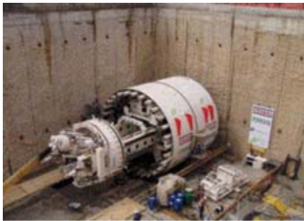
Figure ap.7.12.6 The TBM into the launching shaft.
