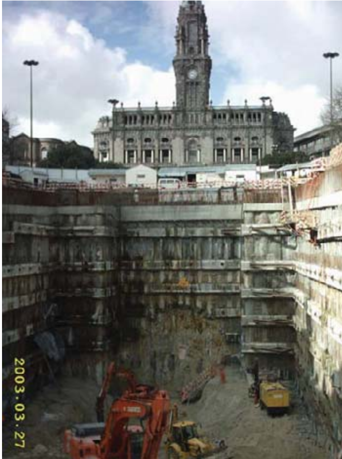
Figure 8.17 View of the Aliados station before TBM breakthrough.
