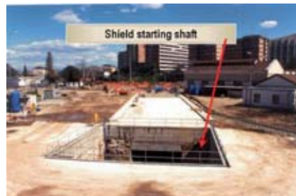
Figure ap.7.10.7 “Quattro Venti” job site area and shaft.
