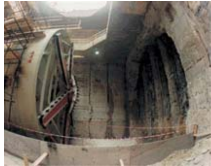
Figure ap.7.7.1 The TBM approaching the tunnel.
