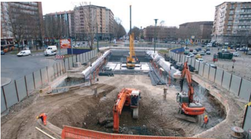
Figure 8.31 Excavation of a station from the surface.
