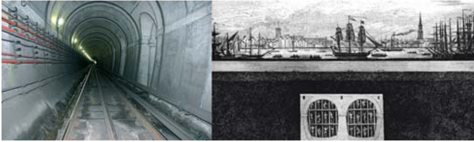
Figure 1.5 Brunel's shield in action on the left under the Thames (Mathewson et al., 2006) which is today still part of the "East London Metro Line" (on the right).
