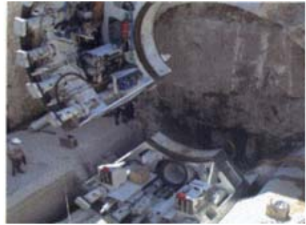
Figure ap.7.10.5 Picture during assembling operation.
