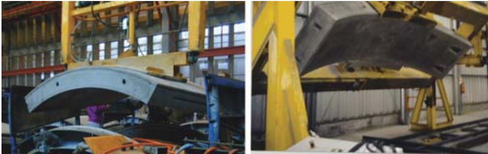
Figure 5.79 Segment extraction from mould and rotation.
