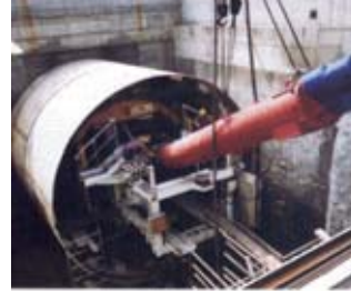
Figure ap.7.6.3 TBM assembling in Milan job site.
