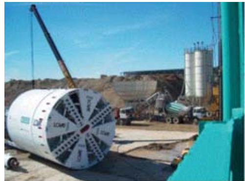
Figure ap.7.9.1 The TBM for excavating the Line 1 extension tunnel.
