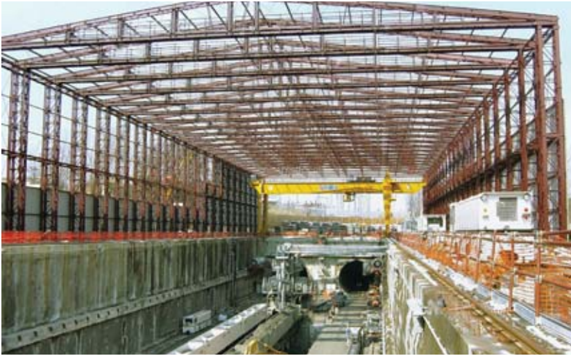
Figure 8.54 Overview of the South Portal of the Tunnels.
