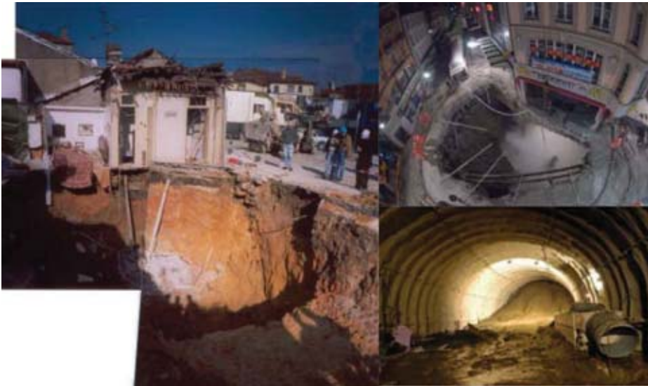
Figure 6.1 Some pictures of collapse consequences.
