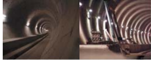
Figure ap.7.12.3 The excavated tunnel.
