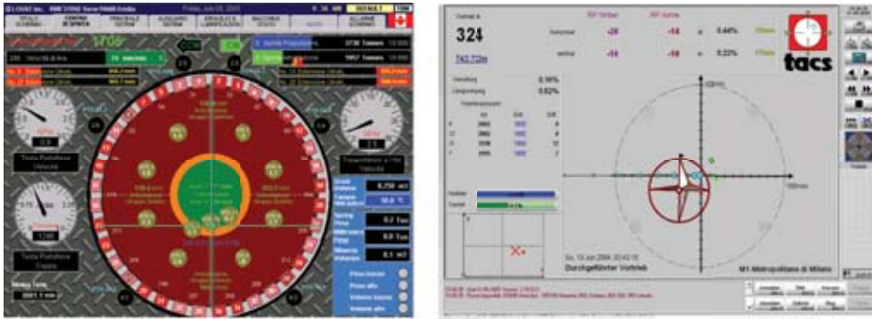
Figure 4.14 An example of a control panel (left) and a guidance screen (right) in an EPBS machine.
