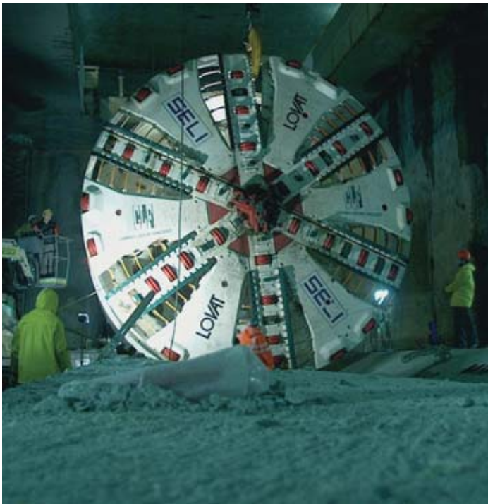
Figure 7.3 Winter assembly of a TBM at the bottom of a shaft.
