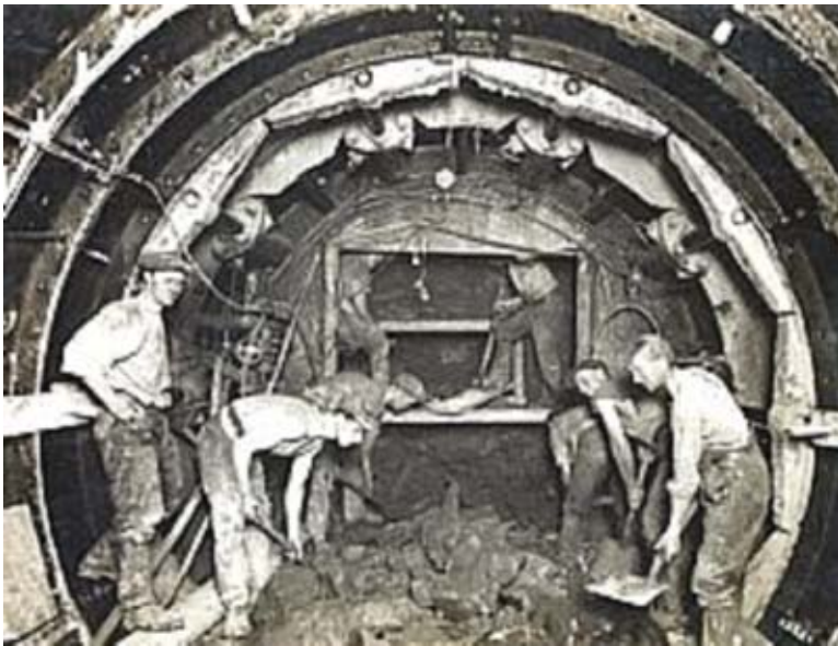
Figure 1.7 A picture of the “Greathead's shield”, taken in the 1900s, used for tunnel excavation since late 1800s, illustrating the circular shape and the metallic rings lining the excavation walls.
