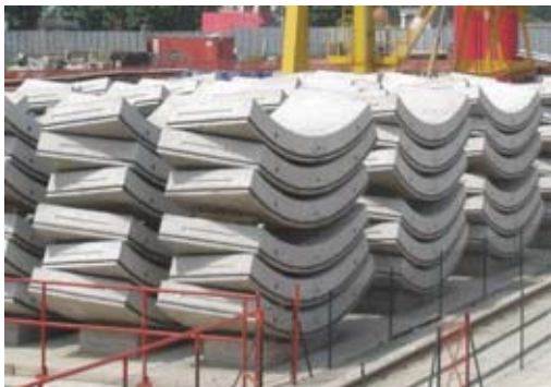
Figure ap.7.13.3 Segment stored in Metro of Brescia site.
