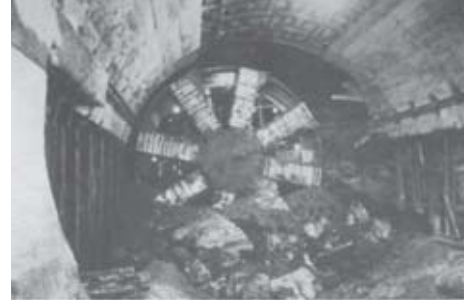
Figure ap.7.1.1 The TBM excavating the Line A tunnel.
