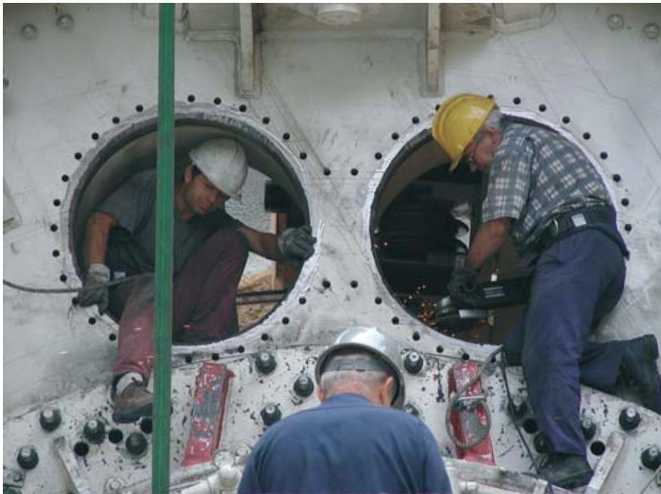
Figure 7.6 Assembling air locks.
