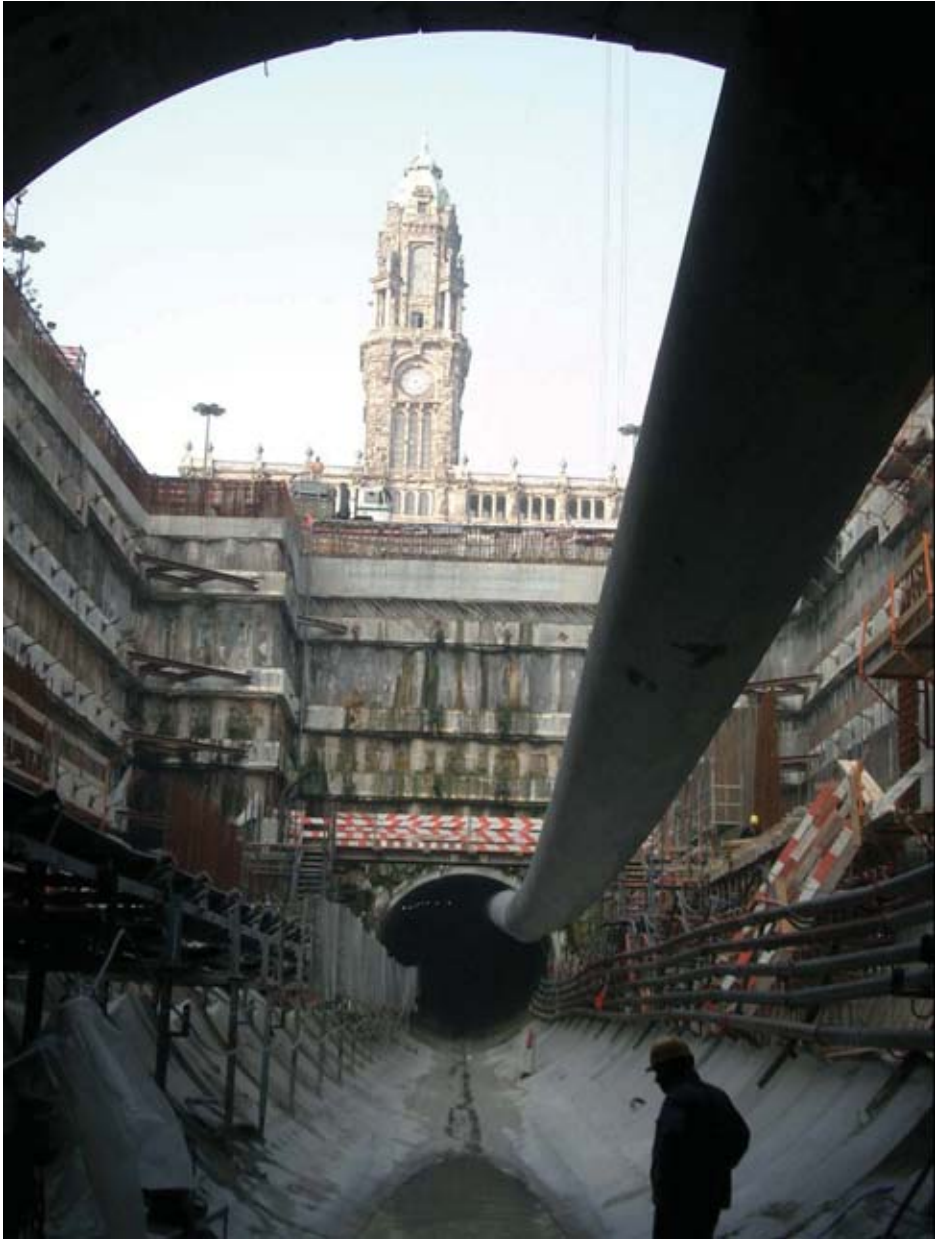
Figure an.6.4 Aliados Station in the Porto Metro Line C.
