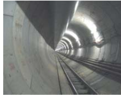
Figure ap.7.11.3 The excavated tunnel.
