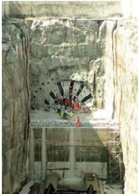
Figure 8.48 One of the breakthroughs during tunnelling in the SMART Project.
