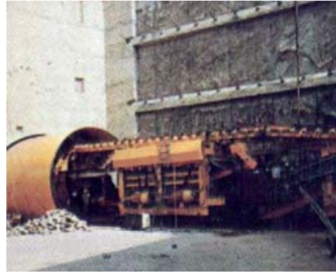
Figure ap.7.2.1 The TBM for excavating the Line B tunnel.
