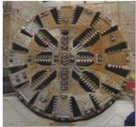
Figure ap.7.13.1 The TBM for excavating the Metro of Brescia tunnel.
