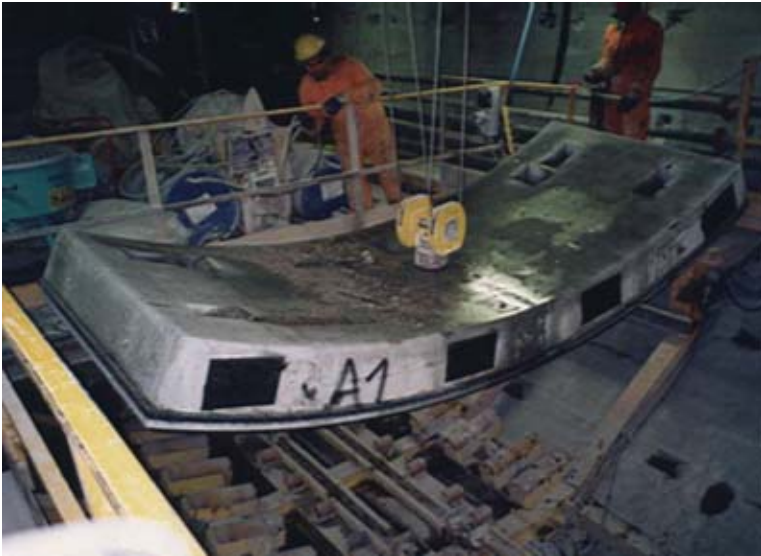
Figure 5.52 A segment with load distributing pads.
