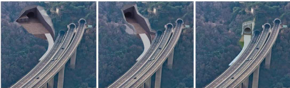
Figure 5.1 Rendering examples of different hypotheses of Delle Grazie Tunnel portal of the Gronda Project (Italy). The pictures show the different tunnel portal impacts and excavation at different stages of the project development (from left to right). The design choices were focused to minimize the visual impact of the portal on the hill slope, to reduce the extent of the side roadways (Francesconi & Degni, 2019).
