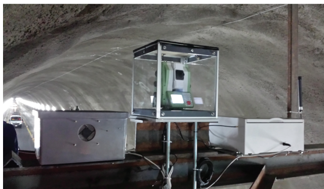
Figure 12.4 Topographic monitoring via automatic total station. (Courtesy of Leica Geosystems.)
