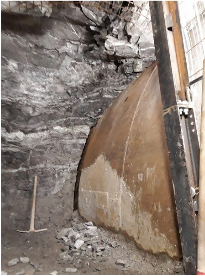
Figure 3.4 Overbreak controlled by the orientation of the discontinuities. (Courtesy of E.M. Pizzarotti.)
