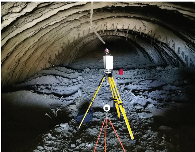
Figure 11.2 Laser scanner monitoring. (Courtesy of Anas S.p.A.)
