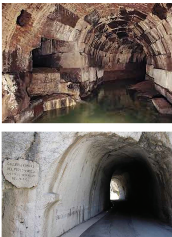
Figure 1.1 Cloaca Maxima (Rome) (above), a 600-metre-long tunnel constructed in Rome between 400 B.C. and 578 B.C. with the purpose of draining the wet areas north of the Palatine Hill, and the Furlo Tunnel, still in use, opened by Emperor Vespasiano in A.D. 76 (below).
