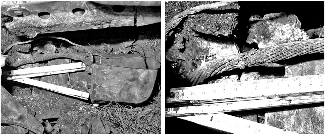
Figure 3.10 Photographs of the traces of electrical sparking observed in the circuitry of HGV 1
