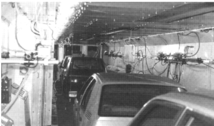
Figure 12.6 Inner view of the full-scale double-deck shuttle wagon mock-up used to investigate fire safety concepts and installations for the Channel Tunnel
