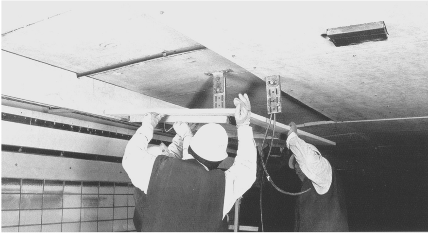
Figure 7.10 The Promatect tunnel-lining system (Photograph courtesy of Promat International Ltd – Tunnel Fire Safety)
