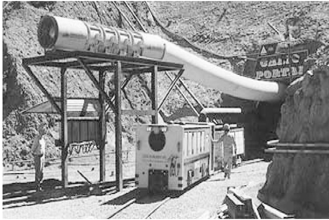
Figure 4.11 Diesel locomotive with ventilation arrangement at the portal of a tunnel – a track system layout (courtesy of GIA Industri AB)
