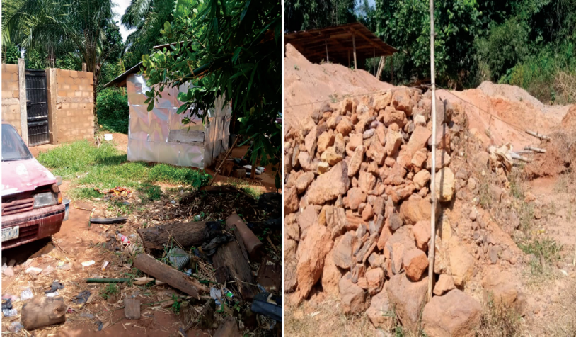
Plate 3.4 Parts of the Ezekoro forest where buildings construction is taking place.
