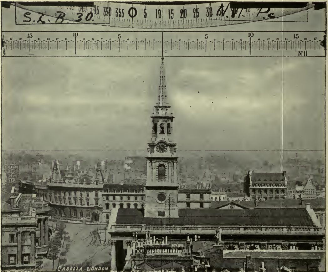
FIG. 64B.—Picture from Bridges-Lee Photo-theodolite.
