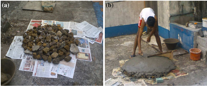
Fig. 4.8 Making of parabolic dome. a Rubble works. b Laying cement on rubbles
