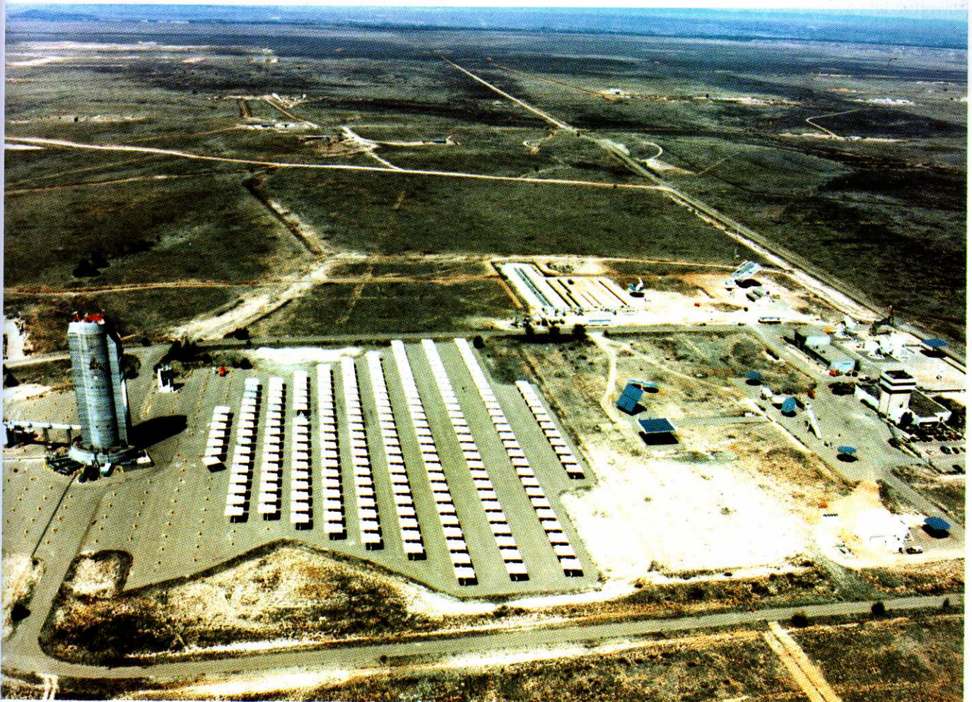
Figure 5-1. The 5.5-MW t central receiver test facility (CRTF) at SNL in Albuquerque, New Mexico, USA (Source: SNL)
