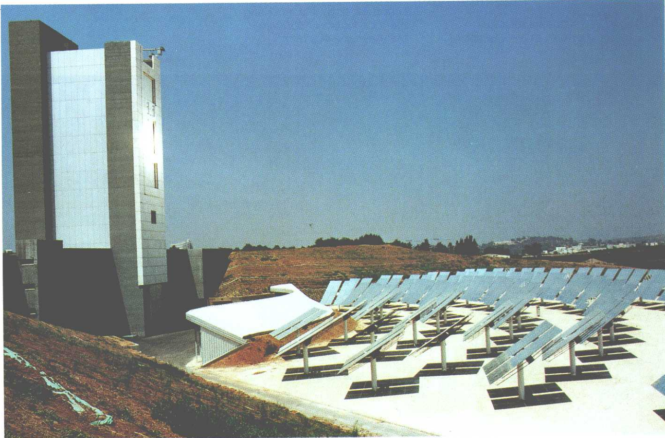
Figure 5-13. The 3-MW t central receiver research facility of the Weizmann Institute of Science in Rehovot, Israel (Source: WIS)
