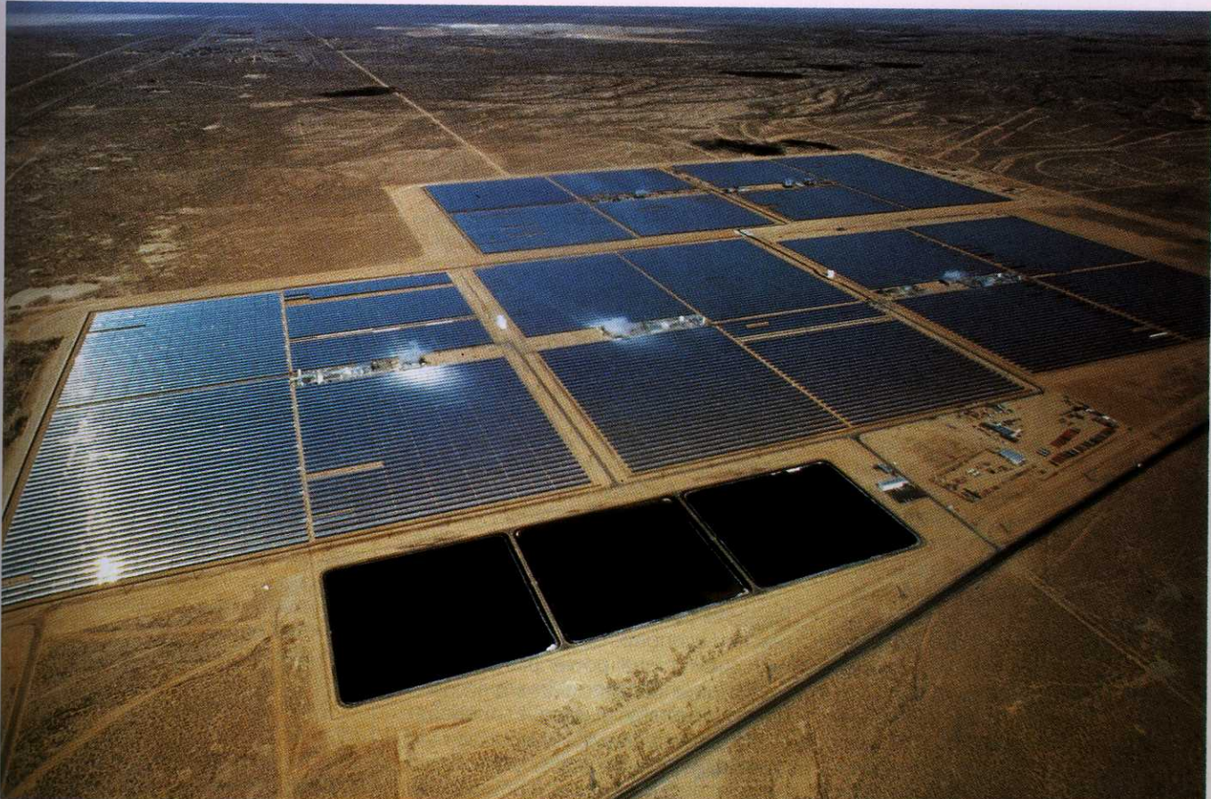
Figure 2-12. Five 30-MW e parabolic trough power plants, SEGS III-VII, at Kramer Junction in California, USA (Source: Flagsol)
