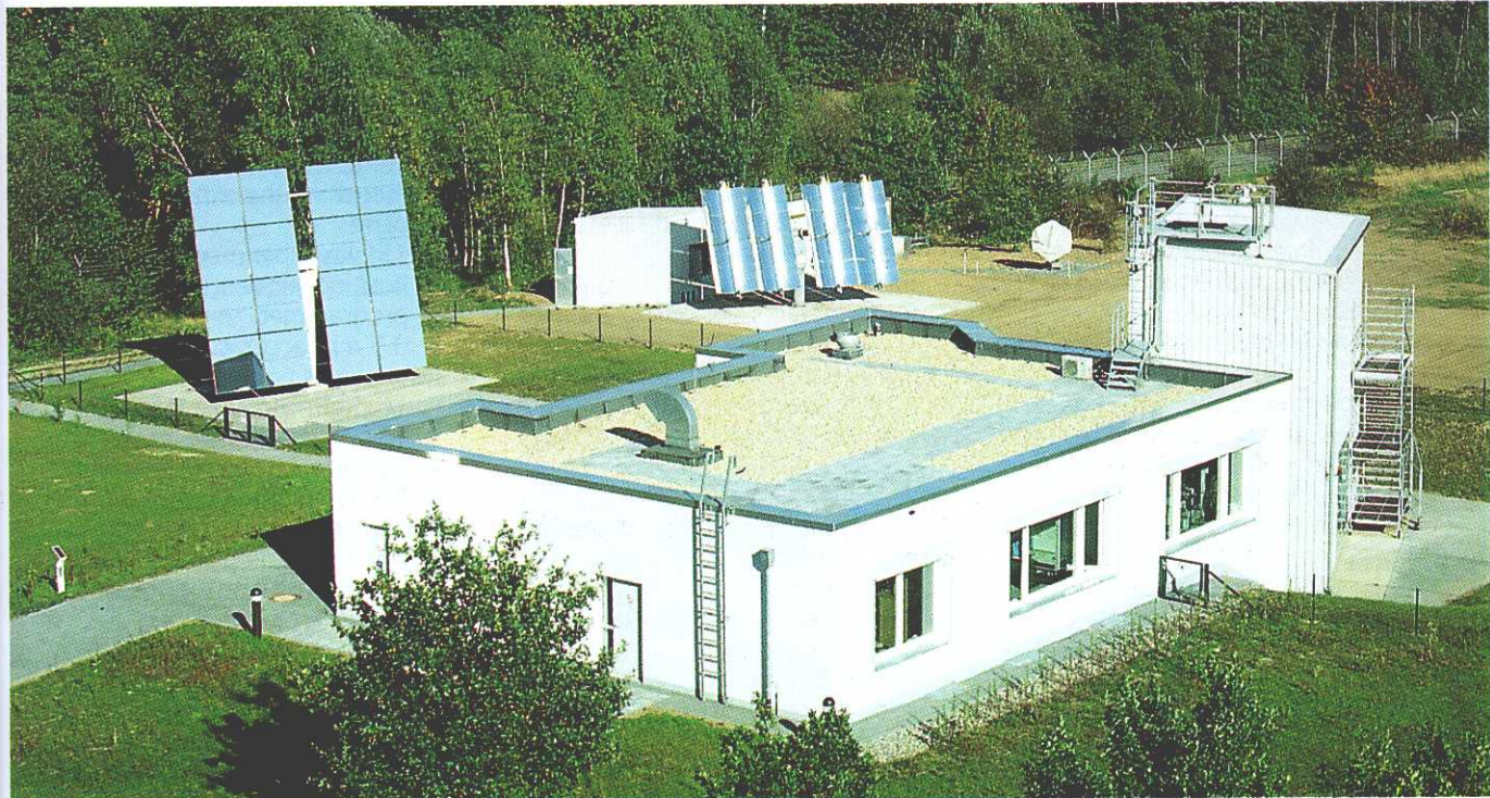
Figure 5-9. The high-flux solar furnace of DLR in Köln*
