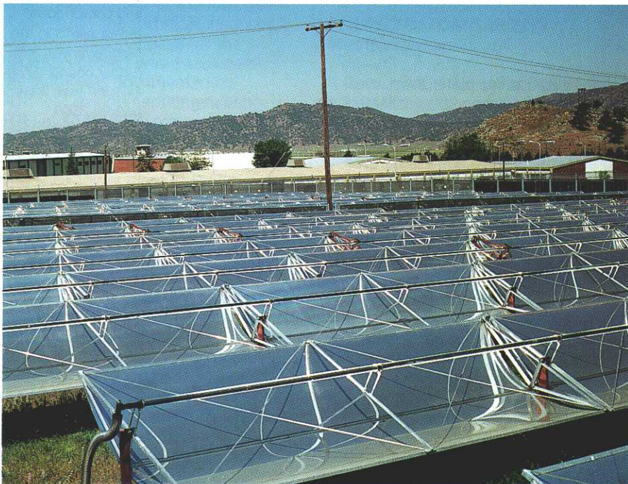
Figure 2-29. System supplying process hot water to the California Correctional Institution in Tehachapi, California, USA (Source: IST/INREL)
