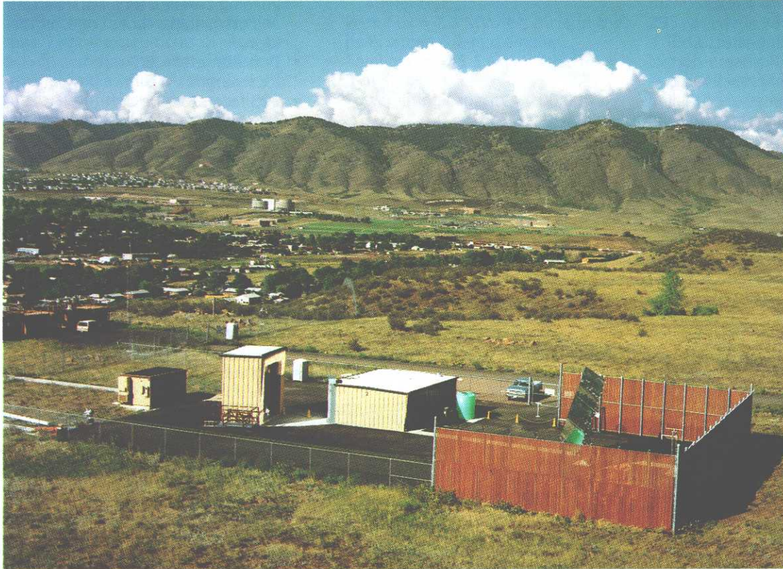
Figure 5-4. The 10-kW high-flux solar furnace (HFSF) at NREL in Golden, Colorado, USA (Source: NREL)
