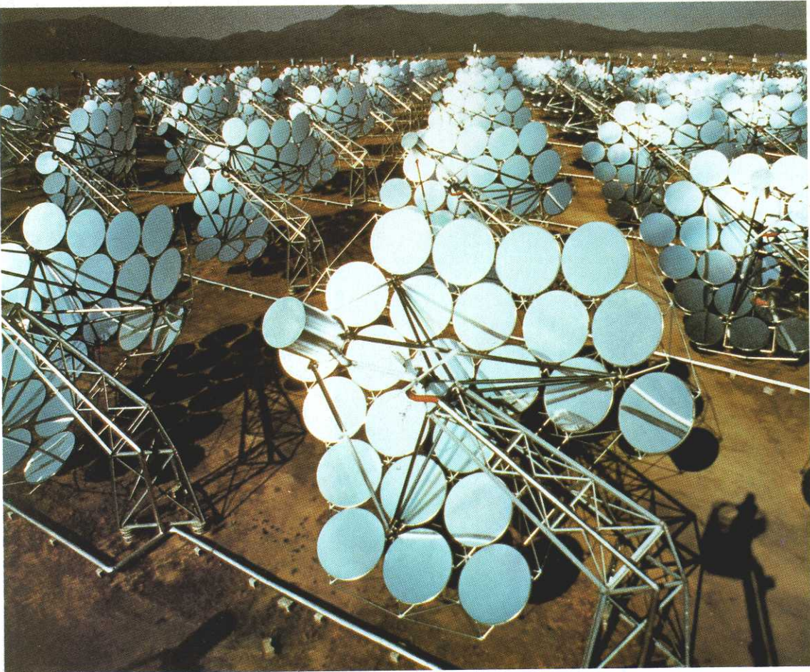
Figure 2-22. Solar One plant at Warner Springs, California, with total power of 4.9 MW e , using 700 LaJet model LEC 460 multifaceted, stretched-membrane dish collectors (9.5-m diameter) (Source: NREL)
