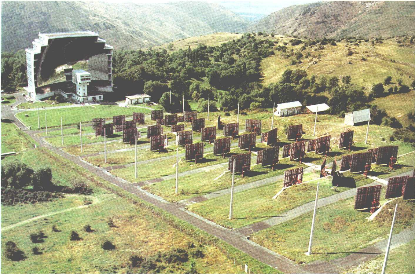
Figure 5-12. The 1-MW high-flux solar furnace at Odeillo, France (Source: CNRS)
