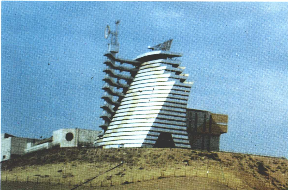
Figure 5-16. The 1 MW high-flux solar furnace of the Uzbek Academy of Sciences in Parkent, Uzbekistan (Source: DLR)
