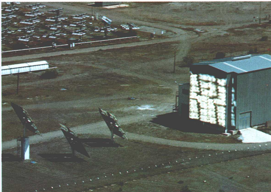
Figure 5-7. The 60-kW PSA high-flux solar furnace, primary concentrator, and focal experimental zone in Almeria, Spain (Source: CIEMAT)
