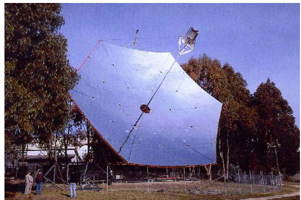
FIGURE 13 The world’s largest 400 m 2 solar dish system. Source: Australian National University.
