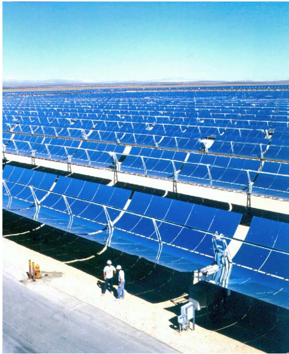
FIGURE 9 View of SEGS trough-based solar thermal power plant in southern California. Source: Kramer Junction Operating Company.
