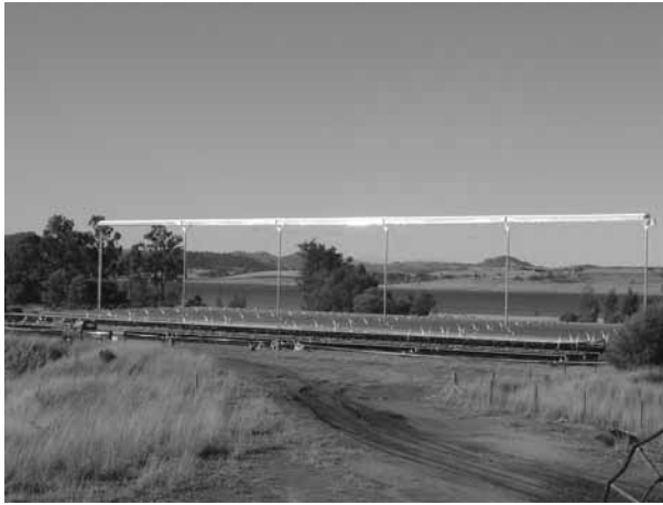
6.13 Stage 1 of the Liddell array in 2004 soon after initial operation (copyright Areva Solar, used with permission).
