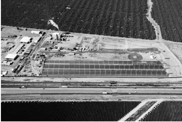
6.16 The three-line Kimberlina array in Bakersfield, California, in late 2008 of LFR technology (copyright Areva Solar, used with permission).
