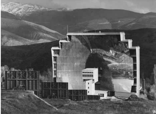
8.2 The French 1 MW solar furnace at Odello employing a field of 63 heliostats each 45 m 2 in area. The working area is in the focal building just in front of the large parabolic mirror.
