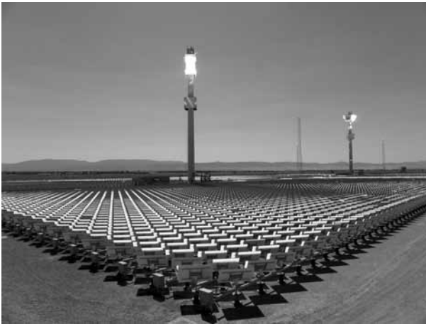
8.7 Two 10 MW th modules of the eSolar (USA) Sierra Sun Tower facility. The receiver in the foreground utilizes four flat panels in an external square configuration, while the background tower carries a north-facing and a south-facing cavity receiver. A total of 24,000 heliostats, each 1.14 m 2 , are factory mounted on support structures (eSolar, with permission).
