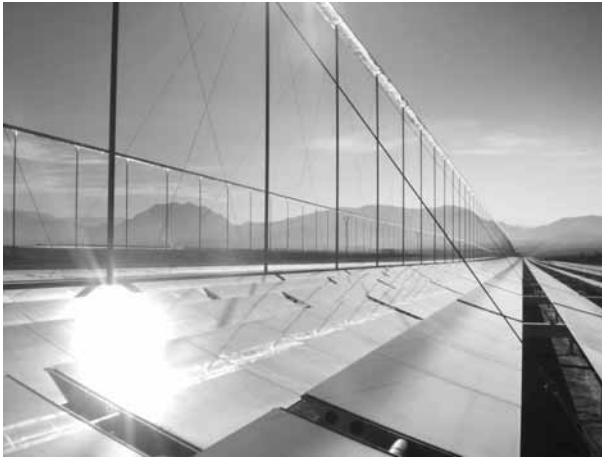
6.26 PE-1 1.4 MW powerplant (courtesy Novatec Solar GmbH).
