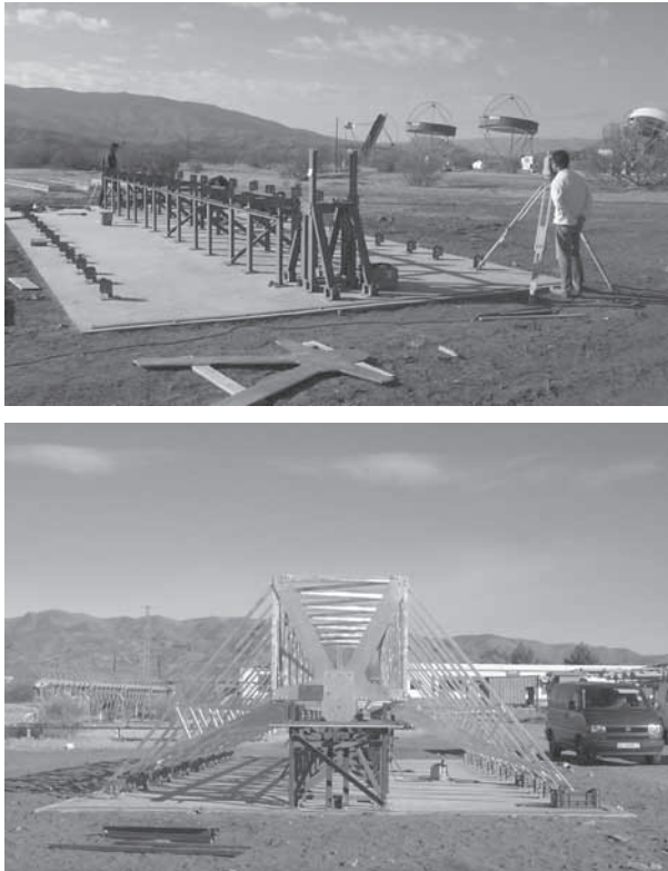
7.6 Check out of the assembly jig for EuroTrough collectors (top) and a parabolic-trough module assembled in the jig (bottom).
