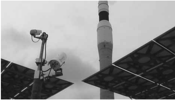
8.8 Torresol's Gemasolar 19.9 MW e commercial molten-salt facility with heliostats and a local BCS station in the foreground and tower/receiver in back, probably in preheat configuration. The active receiver is the central 20% of the white area with the bottom 40% comprising the BCS target (K. Younglove, with permission).
