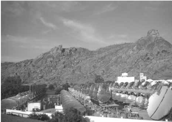
19.4 Sheffler Dishes: solar steam cooking system at Brahma Kumaris, Rajasthan, India (source: Brahma Kumaris, 2007).
