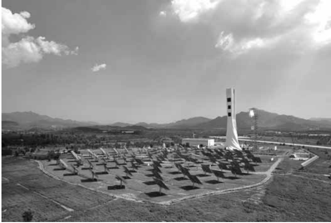
8.5 Photo of the 7.5 MW th experimental/pilot plant of the Chinese Academy of Science near Beijing, China. The illuminated initial cavity receiver/tower stands behind the new tower which has several test apertures (Zhifeng Wang, with permission).
