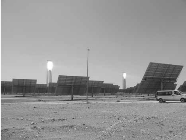
8.6 The two commercial Abengoa (Spain) saturated steam systems, PS10 and PS20 (in back), with 120 m 2 heliostats in foreground.
