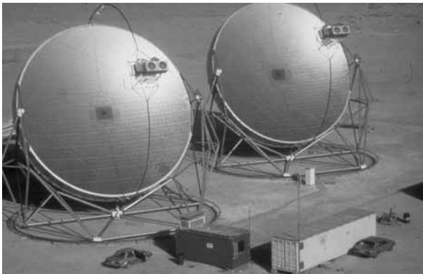
9.4 17 m metal membrane concentrator built by sbp.
