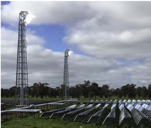
Figure 7.15 1.2\text{-MW}_{\text{th}} sodium receiver at Vast Solar's Jemalong Solar Thermal Station, Forbes, Australia.
