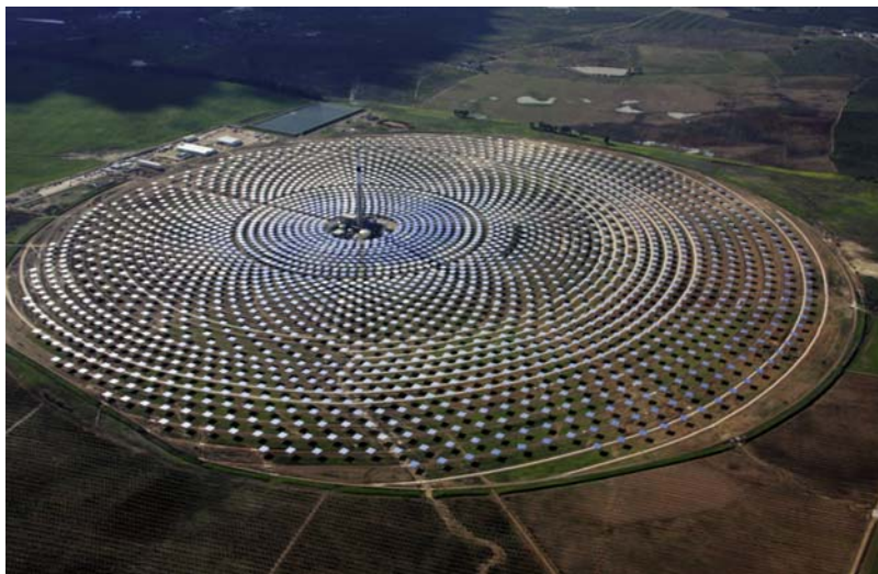
Figure 15.3 Gemasolar plant: 19 MWe, 15 h of storage (Seville, Spain), with operating temperatures going up to 565^{\circ}\text{C} on the molten salt receiver loop ( 540^{\circ}\text{C}/110 bar for the steam produced). Source: SENER/Torresol Energy.
