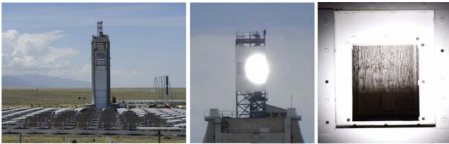
Figure 6.3 On-sun testing of a falling particle receiver at the National Solar Thermal Test Facility at Sandia National Laboratories, Albuquerque, NM.
