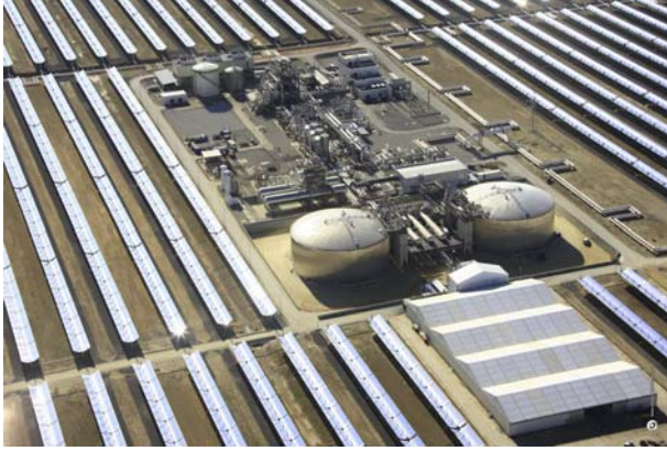
Figure 1.2 Solar field of SENERtrough® cylindrical-parabolic collectors. Arcosol and Termesol thermosolar plants, owned by Torresol Energy. (Source: SENER/Torresol Energy).
