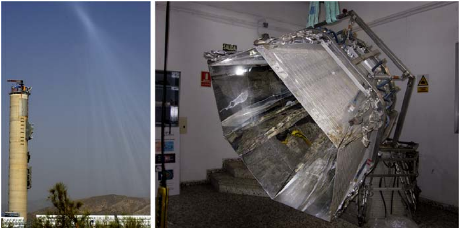
Figure 2.5 CESA-1 tower (left) and REFOS secondary concentrator unit composed of three secondary concentrators (right) at PSA.
