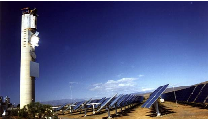
Figure 14.6 CESA-1 tower plant (Copyright by PSA).
