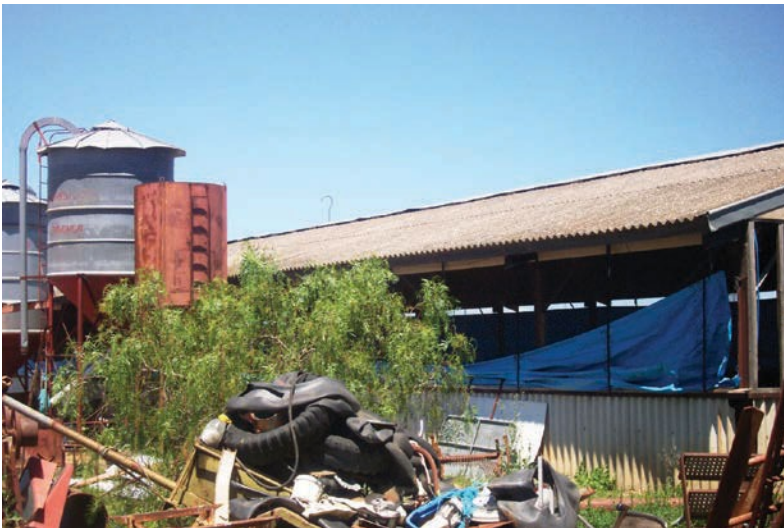
Fig. 1.7i. Older-style buildings with waste materials around the site.
