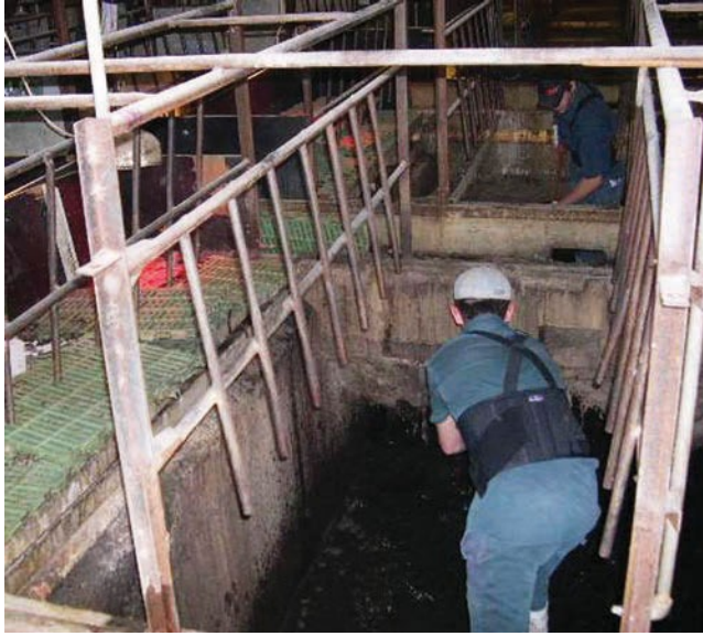
Fig. 7.5ii. Old sheds with workers in full manure pits.
