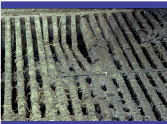
Fig 2.21 – Damaged slats are likely to cause injury. (Courtesy of D. Chennells.)
