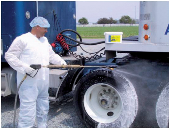
Fig 2.10 – External cleaning and disinfection are important to reduce contamination by faecal material. (From Pritchard et al. (2005), with permission.)
