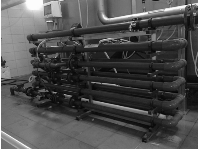
Figure 7.8 Example of pipe flocculator.
