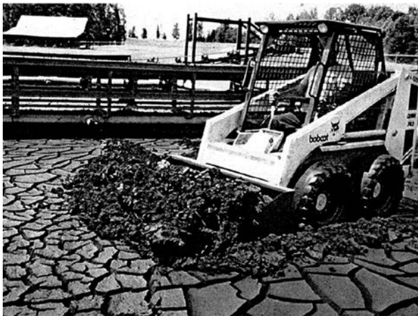
Figure B.9 Removal of cake from drying bed.
