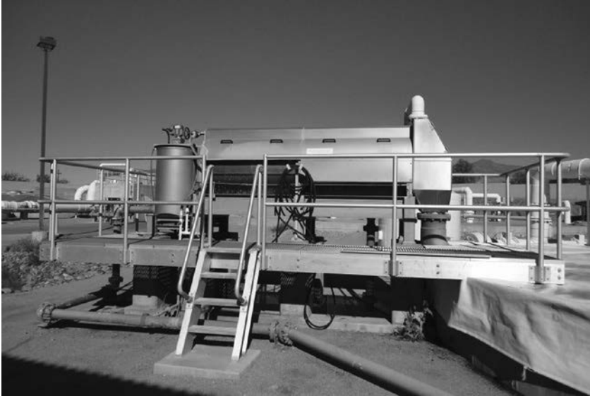
Figure B.19 Rotating drum thickener (Courtesy Parkson: www.parkson.com ).
