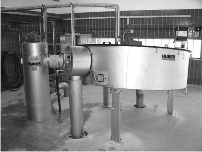
Figure B.20 Disc thickener (Courtesy Huber technology: www.huber.de ).
