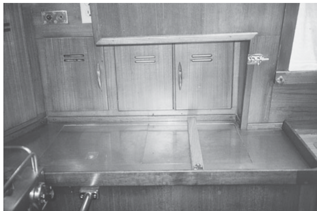
Figure 4-34. A wooden batten anchored in the fiddle and closed with a barrel bolt secures this fridge hatch.
