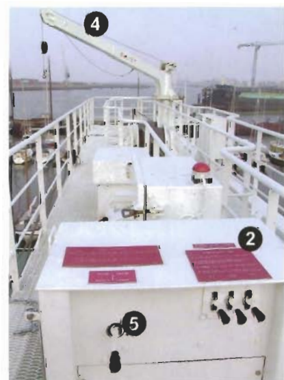
Top of the hatch crane
