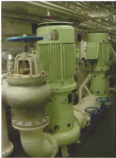
Cooling-water pumps
