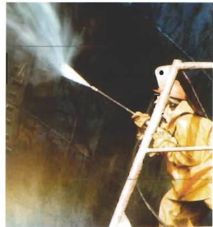
Hydro-jetting of the skin
