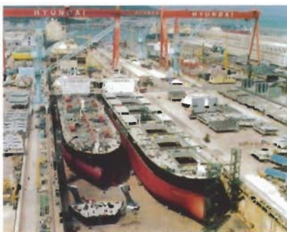
Construction in an excavated dock
