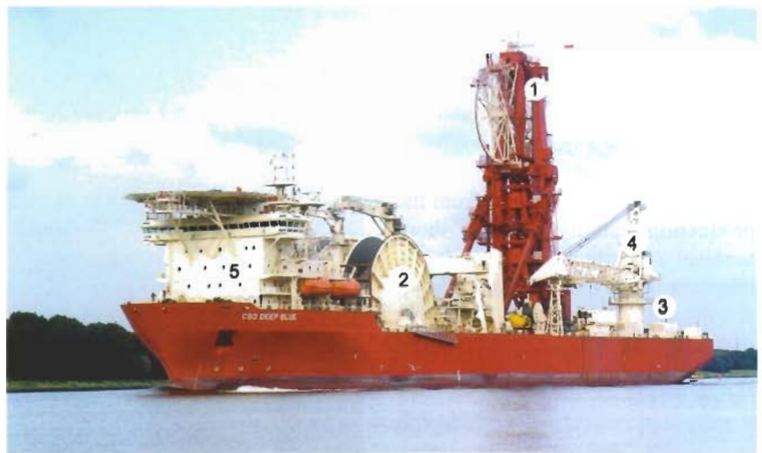
Combined Reel-Lay and J-Lay pipelaying vessel
