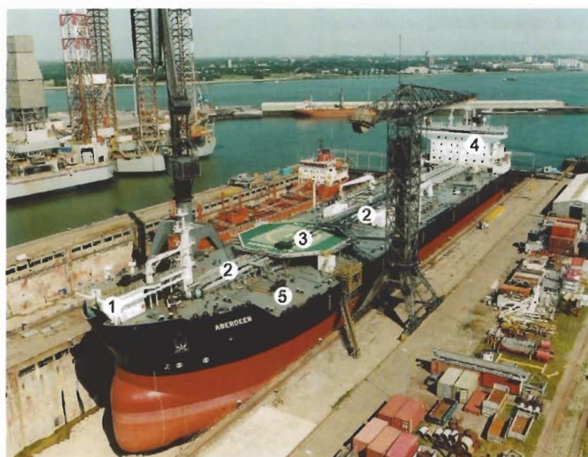
Shuttle tanker in dry dock
