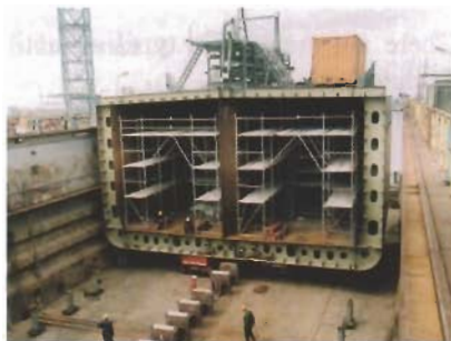
Tanker being built in a dry-dock
