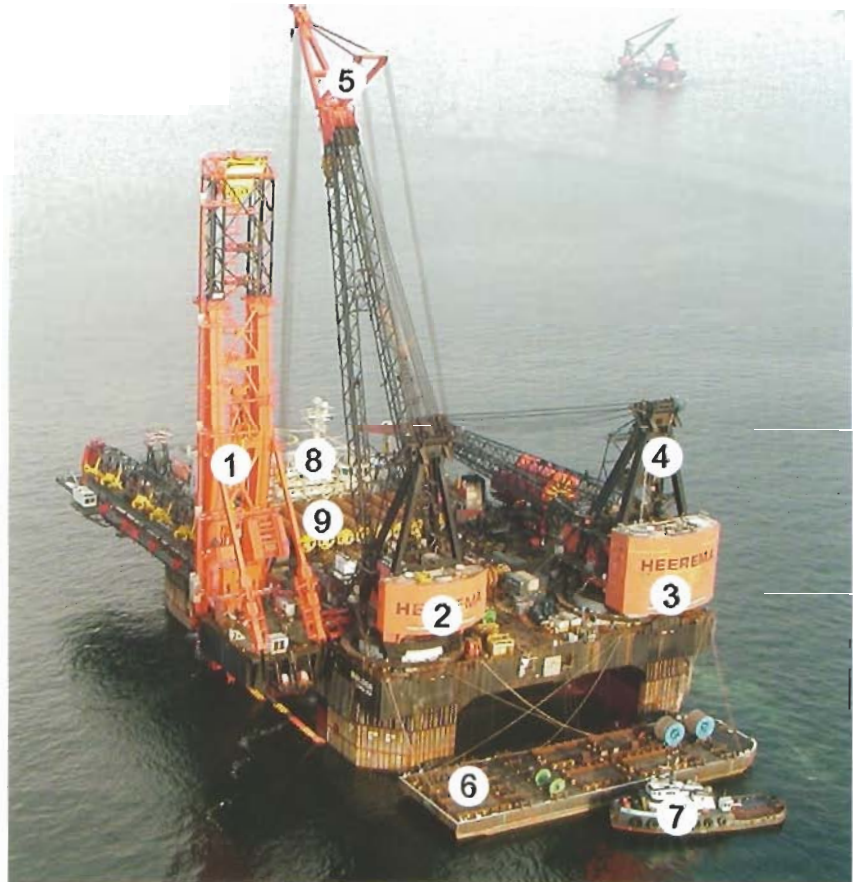
Dual purpose semi-submersible crane vessel for heavy lifting/installation and (J-lay) pipe laying
