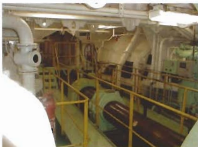
Shafting looking aft
