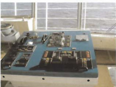
Bridge wing console.
