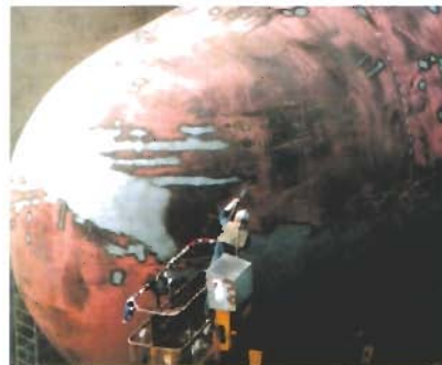
The old paint-layer is removed by gritblasting
