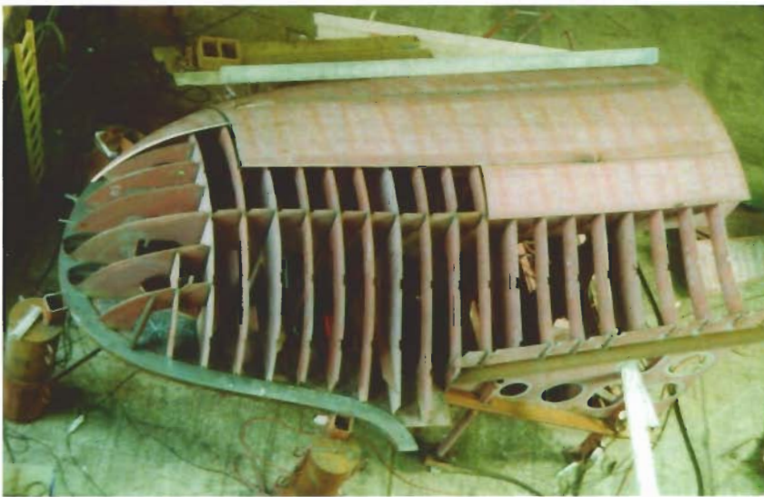
Fitting of the shell plating
