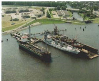
Repair-department of a dockyard with two floating docks
