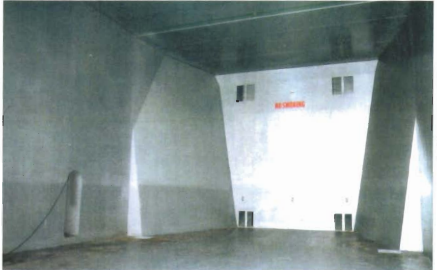
Hold seen in the forward direction (multi-purpose ship)
