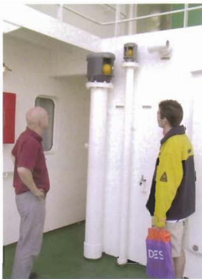
Raised tank vents
