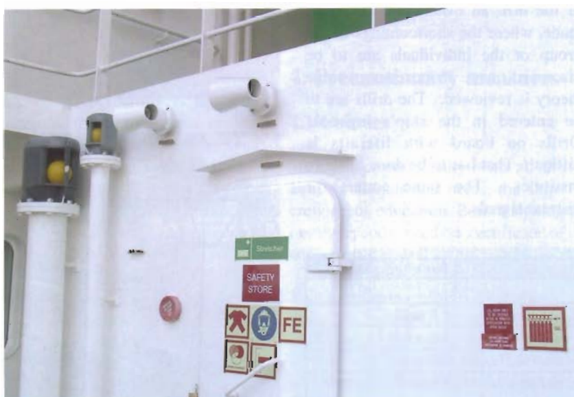
Entrance door with name and technical marking
