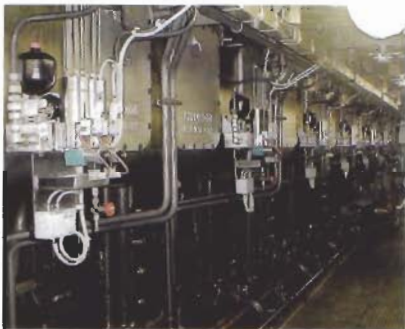
Cylinder lubricators
