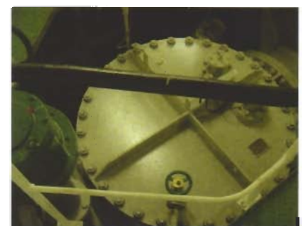
Water inlet filter
