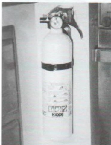
Multi-purpose Dry Chemical A,B,C is a universal extinguisher which can be used on all fires.
