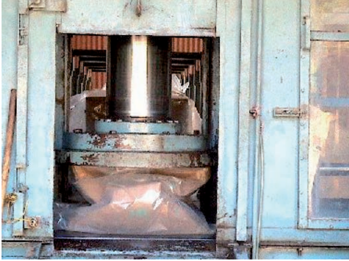
FIG. V-4. HEPA filter compaction stage.
