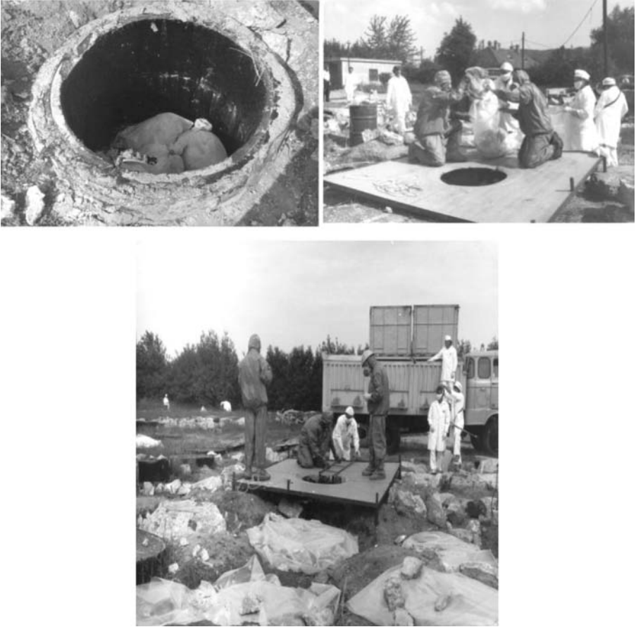
FIG. IV-1. Remediation of the Solymár repository.
