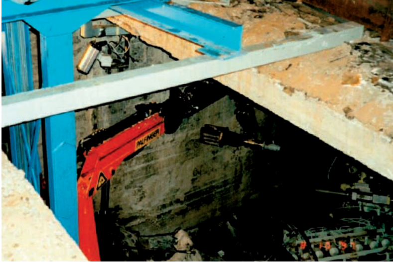
FIG. 7. Removal of waste from a vault with a custom designed manipulator.
