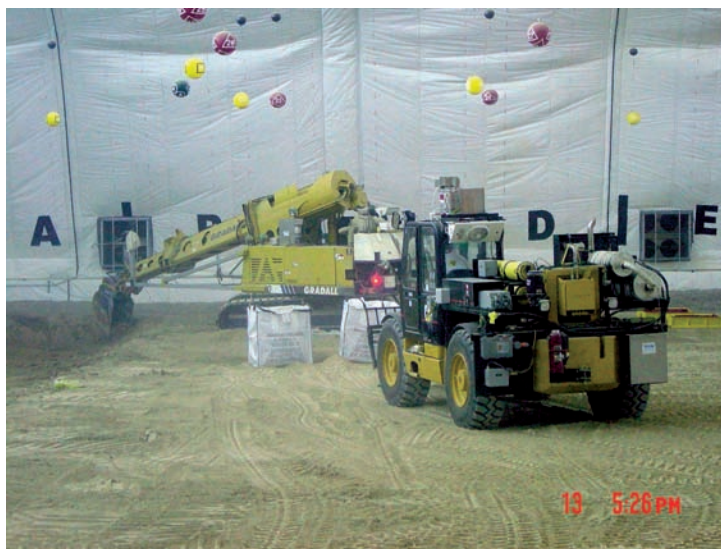
FIG. 6. Remote controlled digger.
