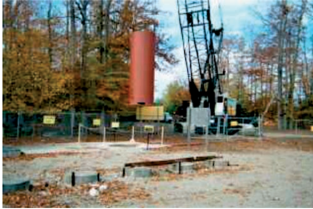
FIG. I-2. Lifting of an encapsulated tile hole.
