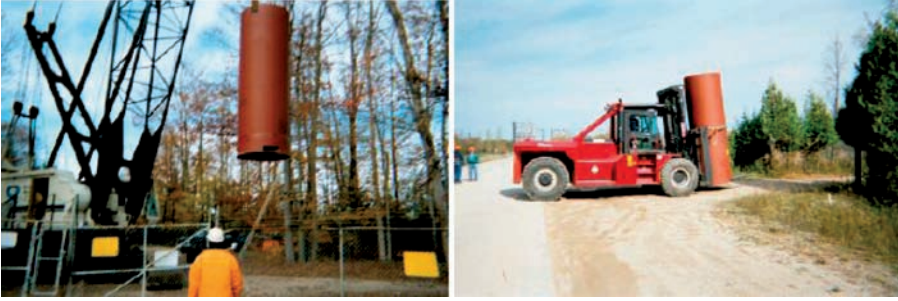
FIG. 8. Lifting a 25 t encapsulated ILW container with a conventional crane and forklift truck.
