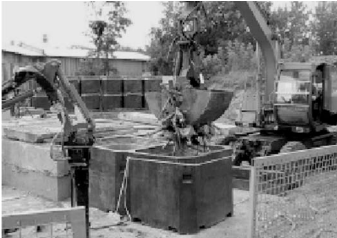
FIG. VI-5. Waste extraction with an excavator clamshell bucket.
