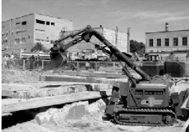
FIG. VI-6. Radioactive waste extraction with robotics equipment.
