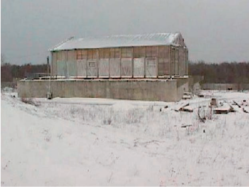
FIG. II-2. Lightweight building erected on top of the SWS to facilitate retrieval of the waste.
