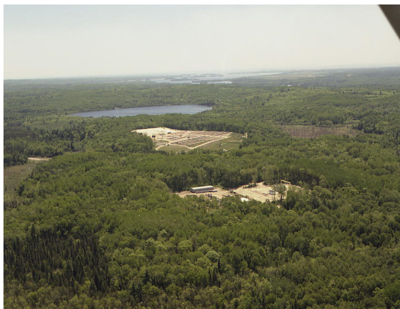
Figure 3: Supervised area looking southeast, showing waste management areas
