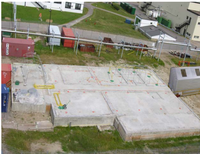
Figure 4: Building 107 north-end concrete floor slab
