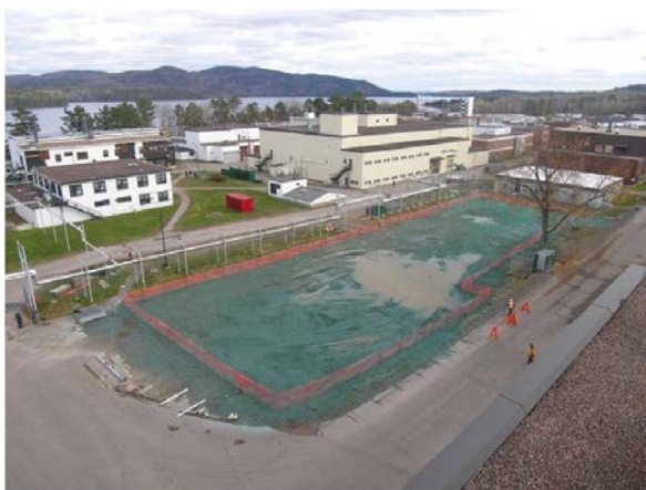
Figure 6: Interim site conditions: Building 107 and concrete slab removed
