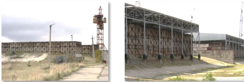
Figure 4.1. SDRW “Pidlisny”: Before and after reparation works
