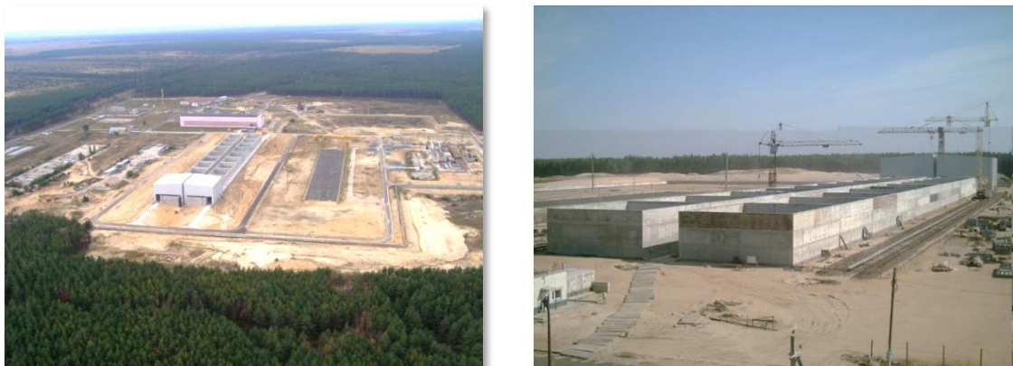
Figure 8.2. The Engineered Near-surface Disposal Facility
