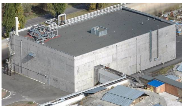
Figure 7.16. Liquid Radioactive Waste Treatment Plant
