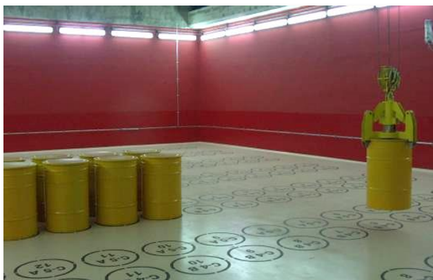
Figure 7.19. LRW curing area
