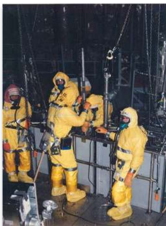
Figure 2.9. Full-scale defuelling work platform
