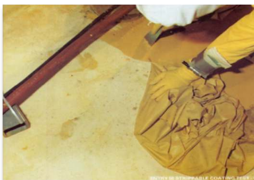
Figure 2.6. Strippable coating for floor decontamination
