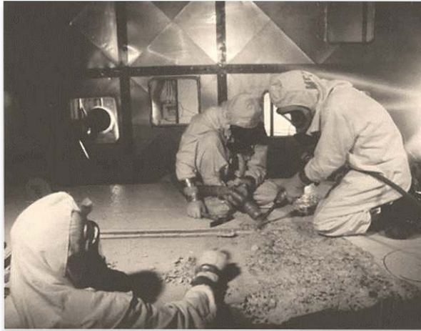
Figure 2.14. Manual debris clean-up operation
