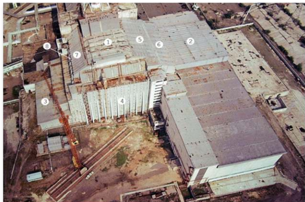
Figure 2.18e. External protective structures of shelter before new confinement installation
