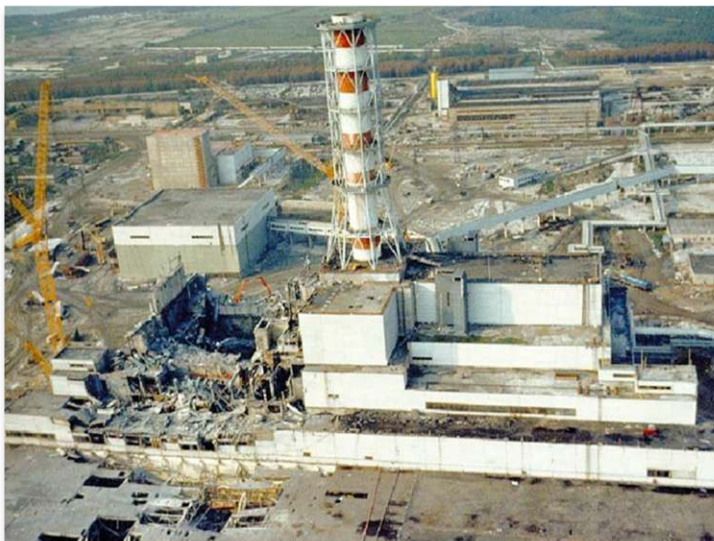
Figure 2.18a. Ruined Unit 4 after graphite fire ended
