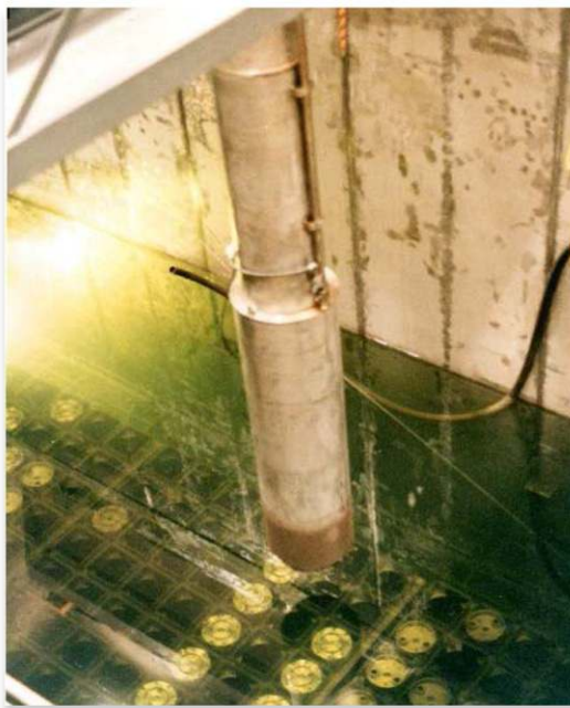
Figure 2.13. Canisters placed in a submerged storage rack in spent fuel pool
