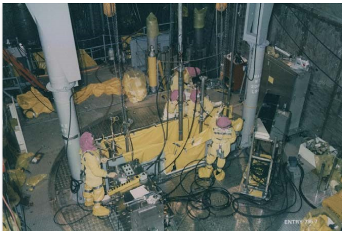
Figure 2.10. Rotating defuelling platform operation
