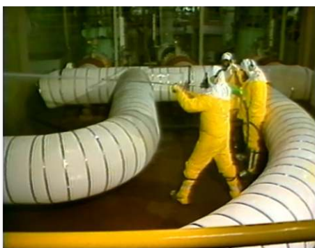
Figure 2.5. High pressure spray decontamination
