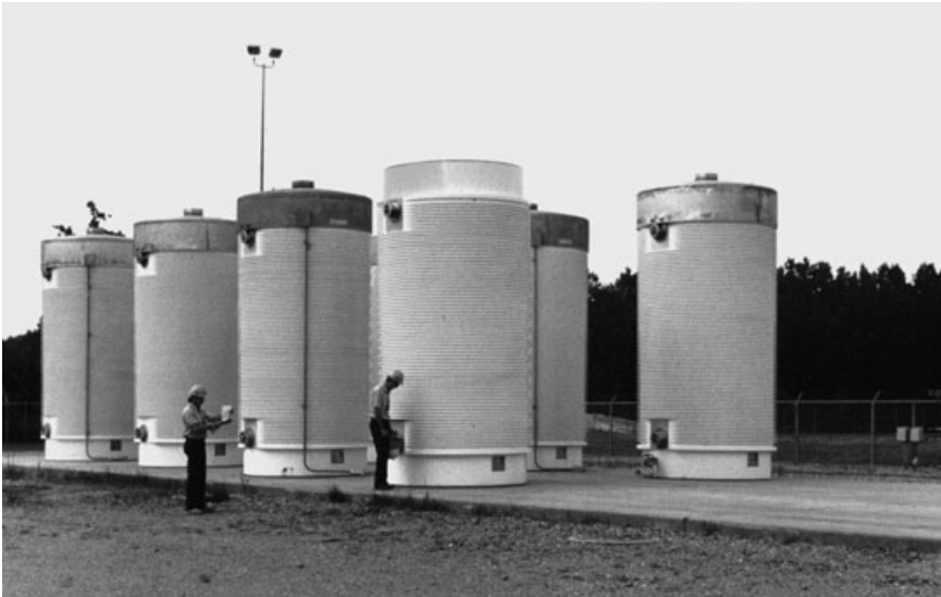
13.6 Dry storage casks facility for spent fuel (source: NRC 2010).
