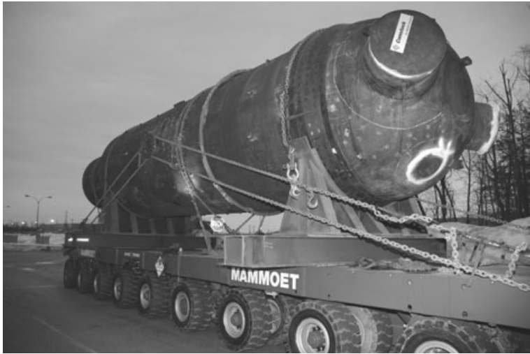
7.1 One-piece removal of steam generator from Bruce NPP, Canada.
