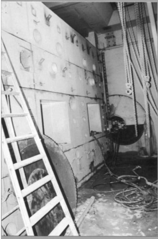
7.5 Use of diamond saw at ORIS decommissioning project (France).
