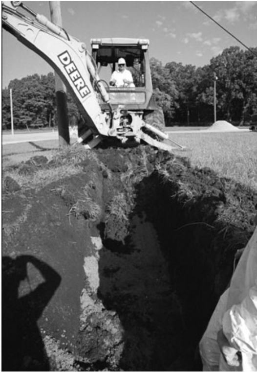
7.2 Removal of underground piping at Argonne National Laboratory, USA.
