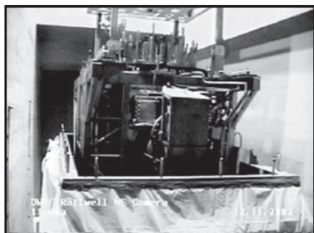
9.7 DWPF Melter One being disposed of after 9 years of operation. The melter was emptied through the emergency bottom drain and lifted out of the melt cell into a waste box for storage and eventual disposal (courtesy of Savannah River Site).
