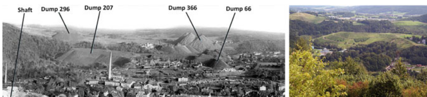
Fig. 5.4 left: dump landscape of the Schneeberg-Oberschlema deposit, 1967; Source Wismut GmbH; right: landscape after remediation. Source Lersow, M., August 2017
