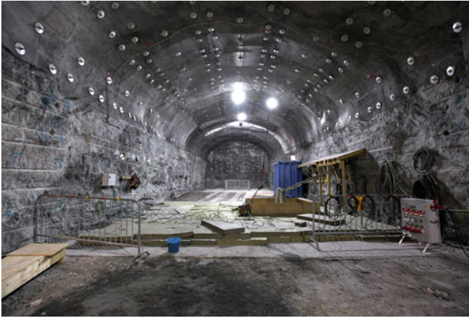
Fig. 8.2 Test gallery (tunnel) in the host rock granite, underground research laboratory (URL) Onkalo/Finland. Source Posiva Oy
