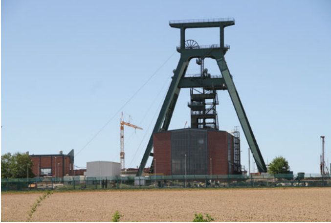
Fig. 6.5 Shaft 1 of Konrad mine in the conversion phase - used for the transportation of personnel and materials
