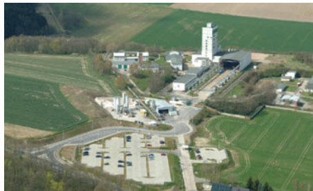
Fig. 6.8 Aerial photograph ERA Morsleben. Source BfS 2009
