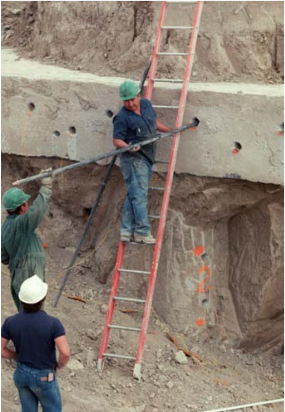
FIG. 20. Initial Engine Test (IET) stack at Idaho National Engineering and Environmental Laboratory (INEEL), USA. Insertion of explosives.
