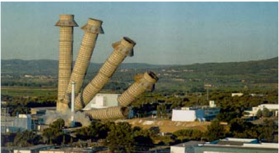
FIG. 22. Time sequence of the stack fall at Marcoule G1, France.
