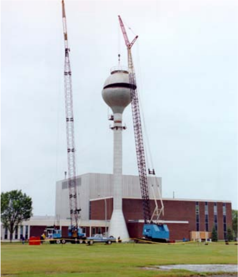
FIG. I.A-2. Removal of the upper half of the water tank.
