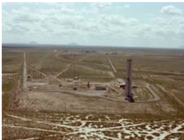
FIG. I.C-1. IET facility with exhaust stack.
