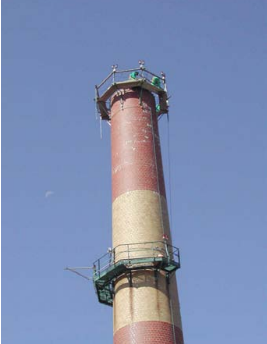
FIG. I.D-5. Bracket and cable scaffold.
