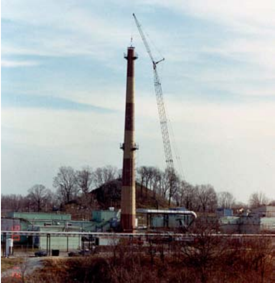
FIG. 1.D-2. Two hundred foot (61 m) crane placing camera platform on stack.
