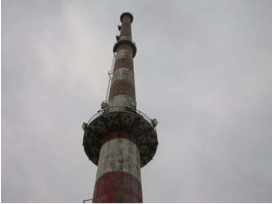
FIG. 9. Stack at Garigliano NPP, Italy.
