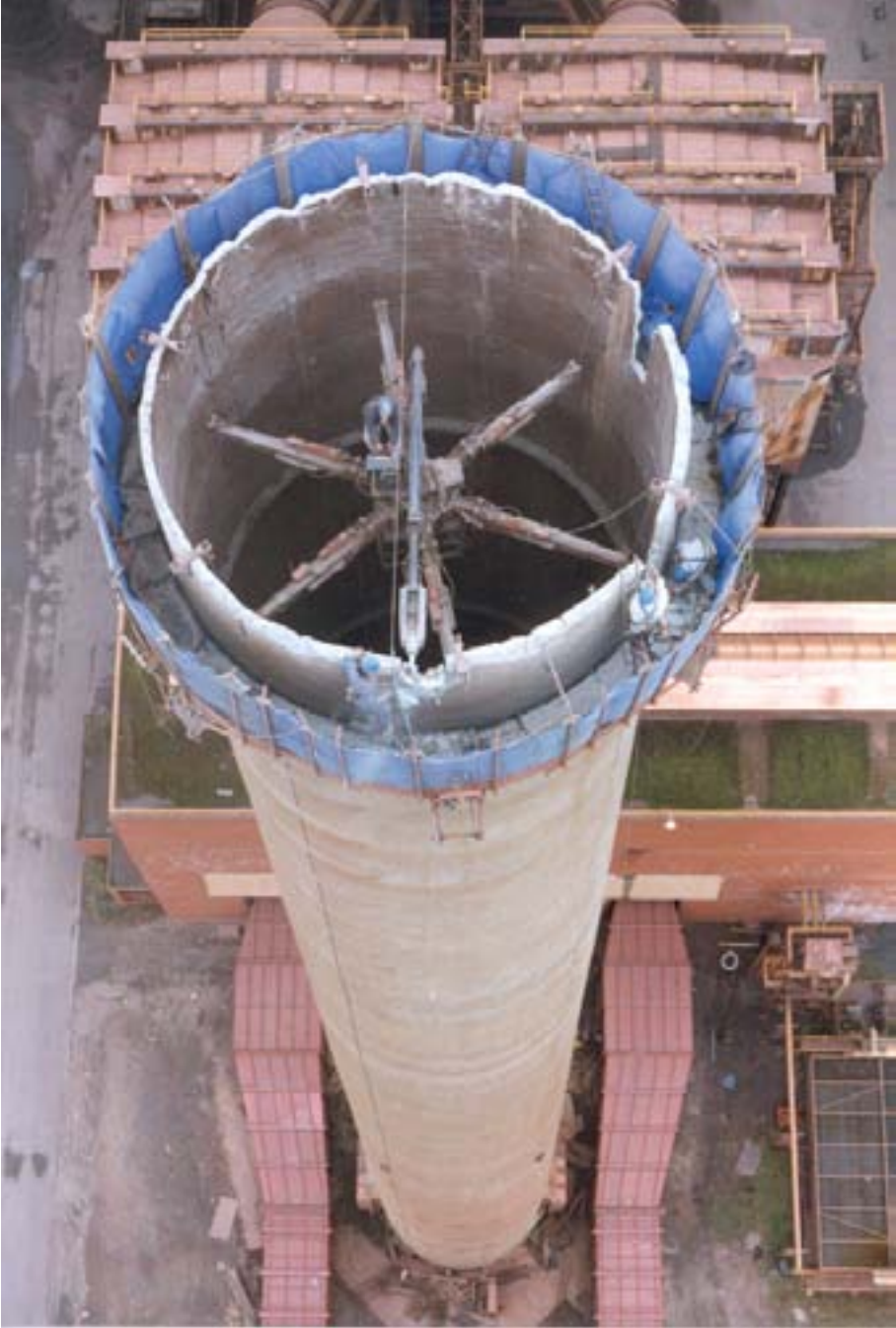
FIG. 3. Brick lined concrete stack at Corus Steelworks, Port Talbot, United Kingdom.
