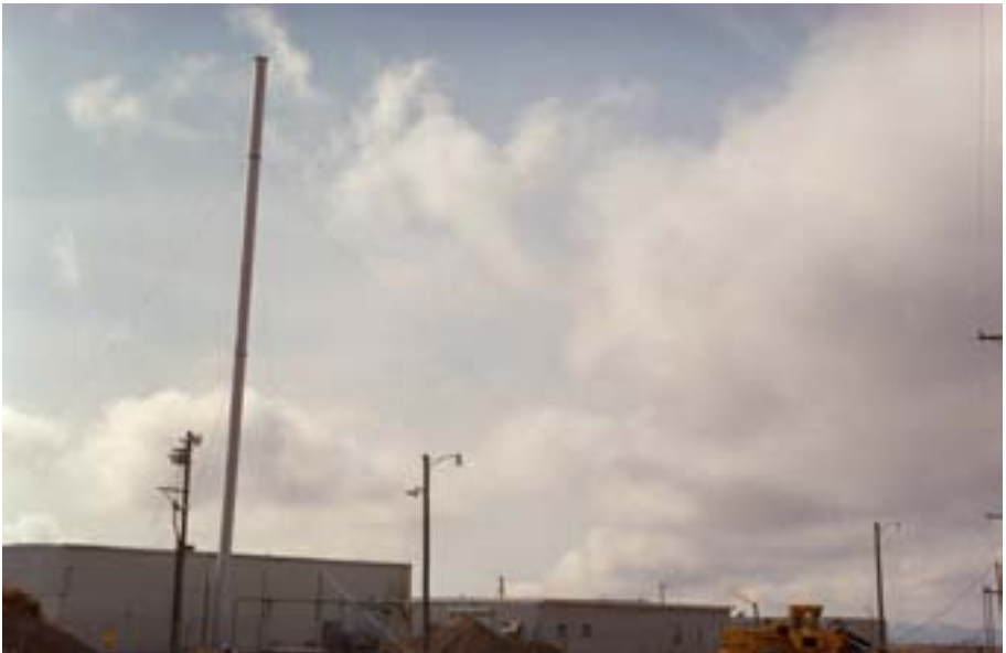
FIG. I.C-5. ARA-715 stack at start of fall.
