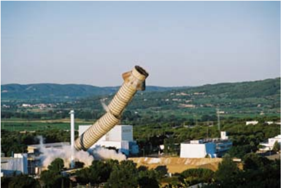
FIG. I.G-8. Felling of the stack.
