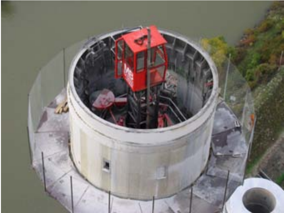
FIG. 16. Gösgen NPP, Switzerland. Climbing saw inserted into the stack.
