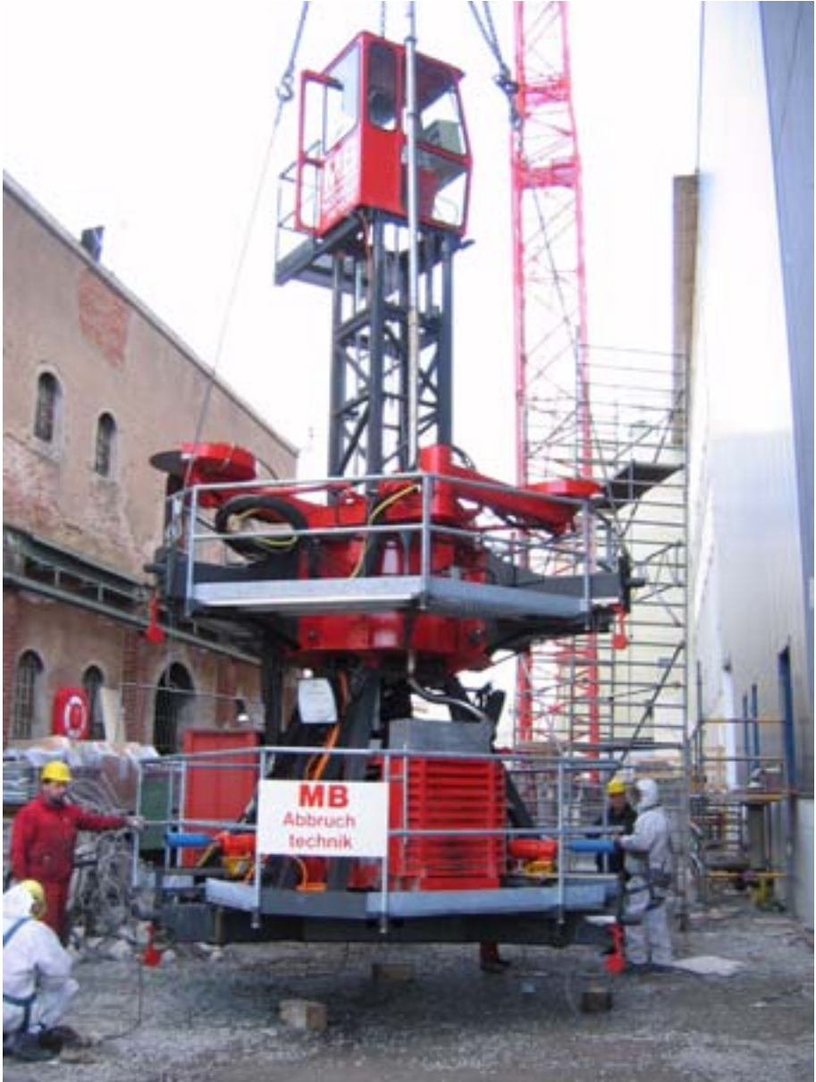
FIG. 1.H-3. View of the climbing sawing machine.
