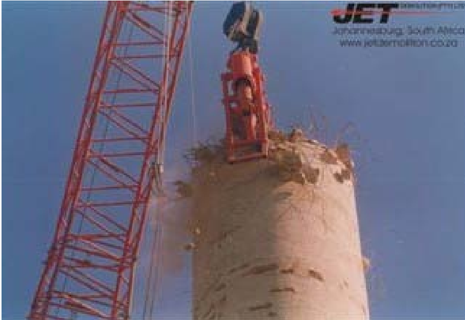
FIG. 19. Top-down breaking of a concrete stack, South Africa.
