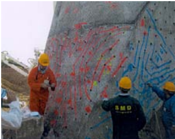
FIG. I.G-5. Drilling of the stack feet before blasting.
