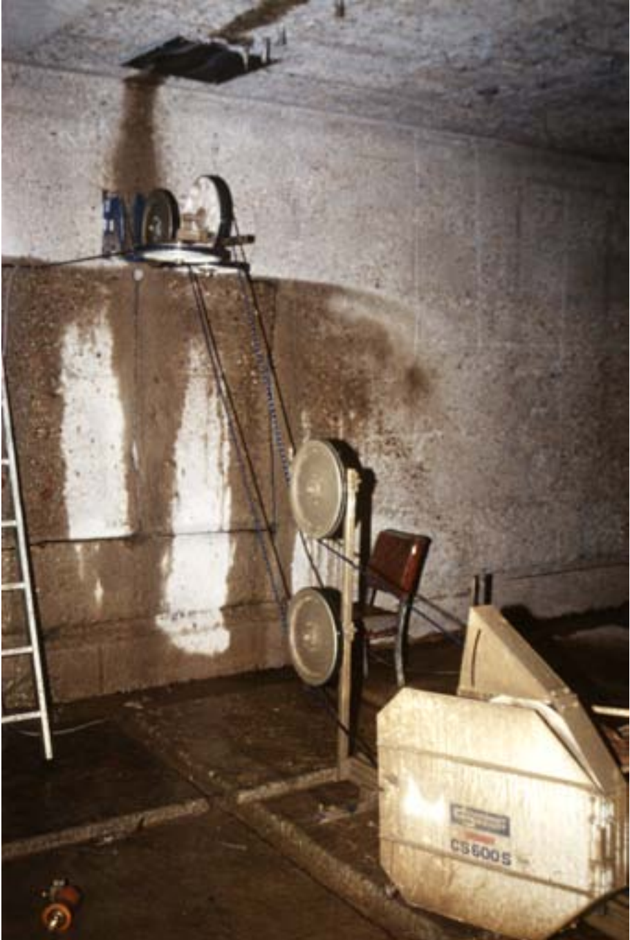
FIG. 12. Creating new cell entrances using a diamond cable cutting machine.
