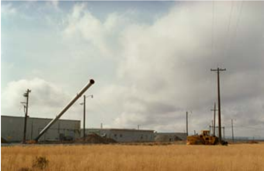
FIG. I.C-6. ARA-715 stack during fall.
