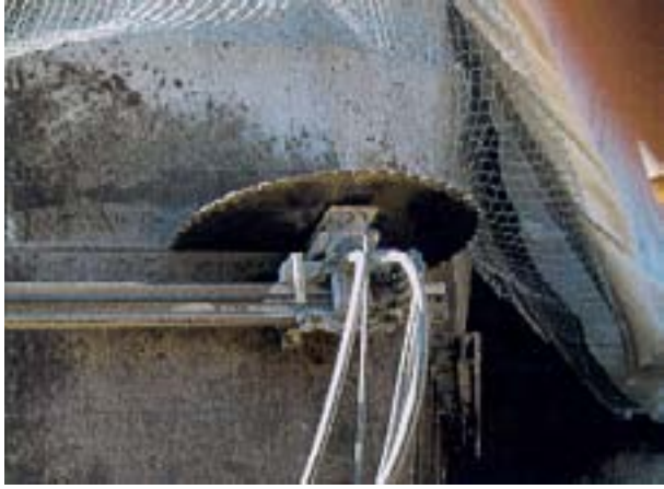
FIG. I.G-7. Sawing of the south foot.
