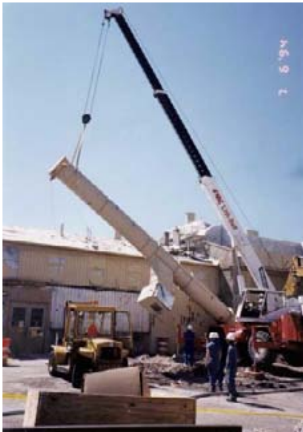
FIG. 23. Exhaust stack intact removal at Los Alamos National Laboratory, USA.
