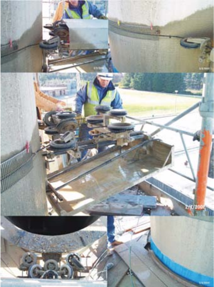
FIG. I.B-6. SGHWR stack decommissioning: wire sawing.
