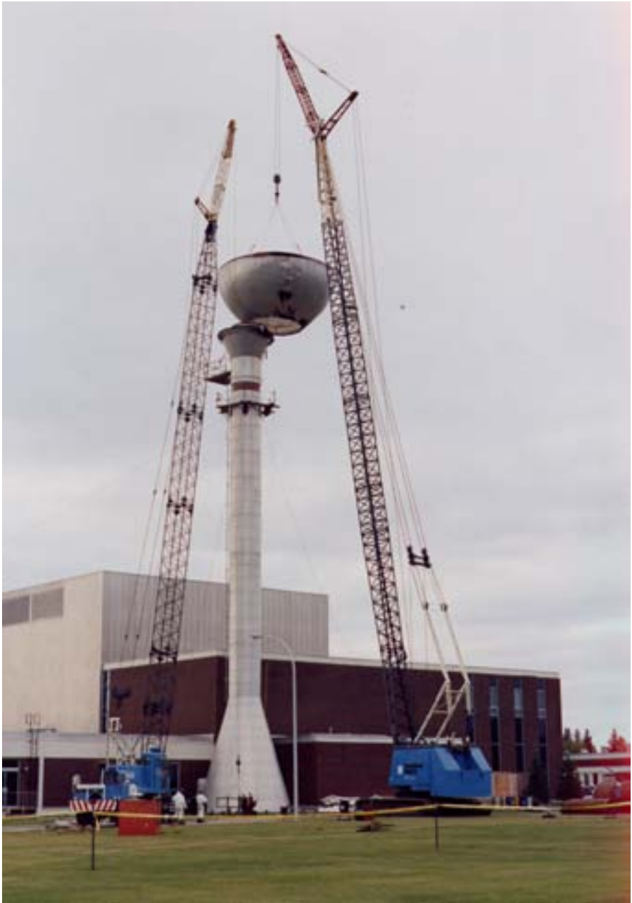
FIG. I.A-3. Removal of the lower half of the water tank.
