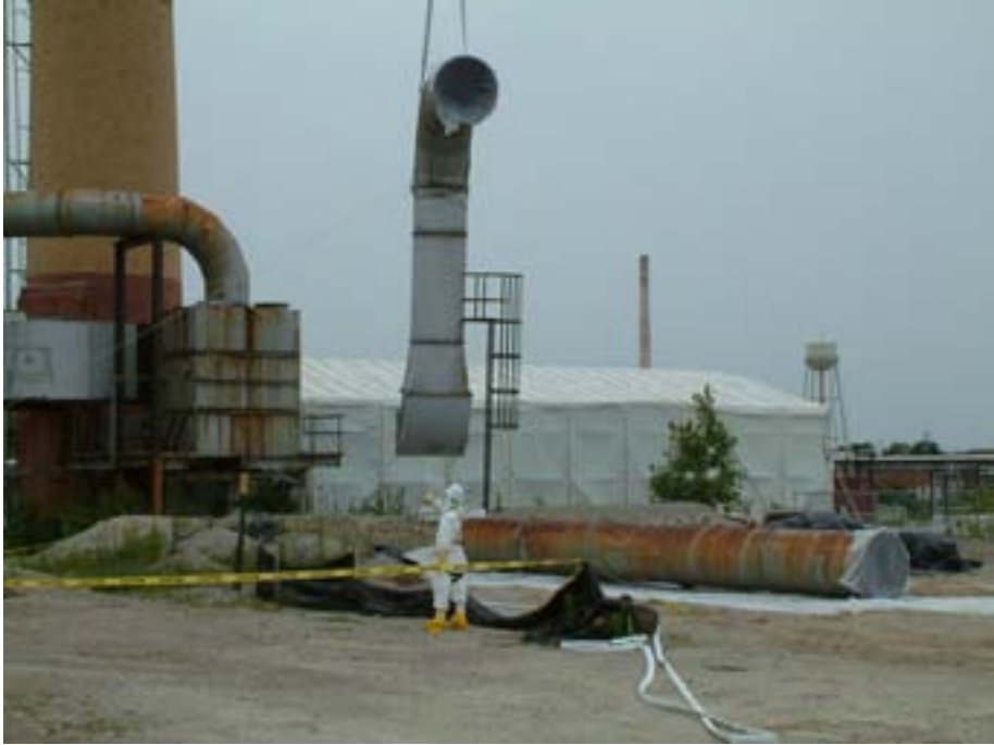
FIG. I.D-4. Lowering 'fogged' exhaust duct.
