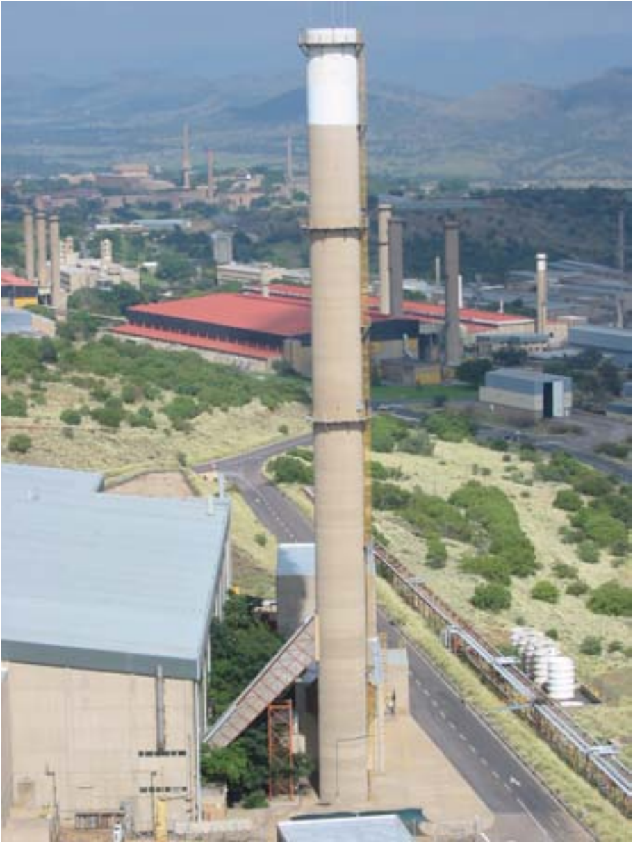
FIG. I.F-1. Stack considered for characterization.
