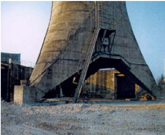
FIG. I.G-3. Demolition of the filling between the stack feet.
