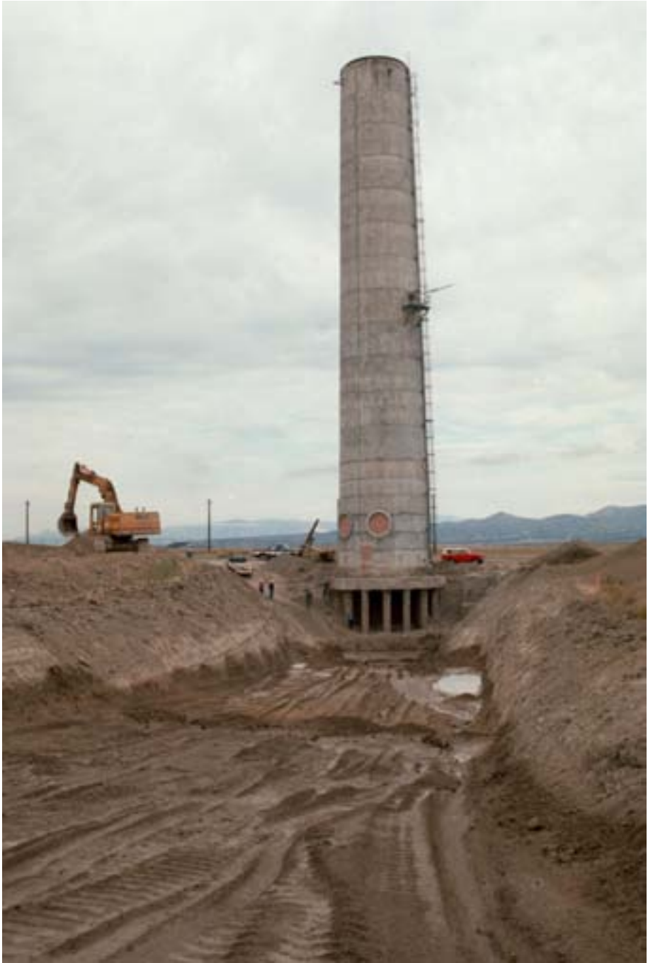
FIG. I.C-2. IET stack, exposed foundation and trench.
