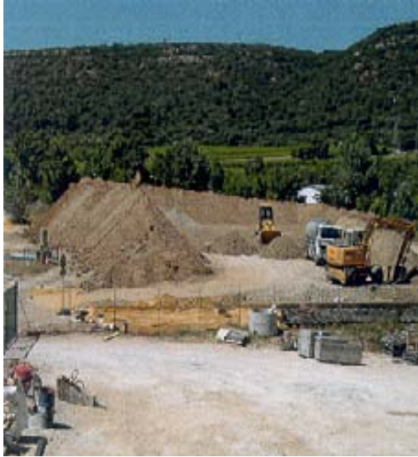
FIG. I.G-6. Construction of the mattress (shock absorber).
