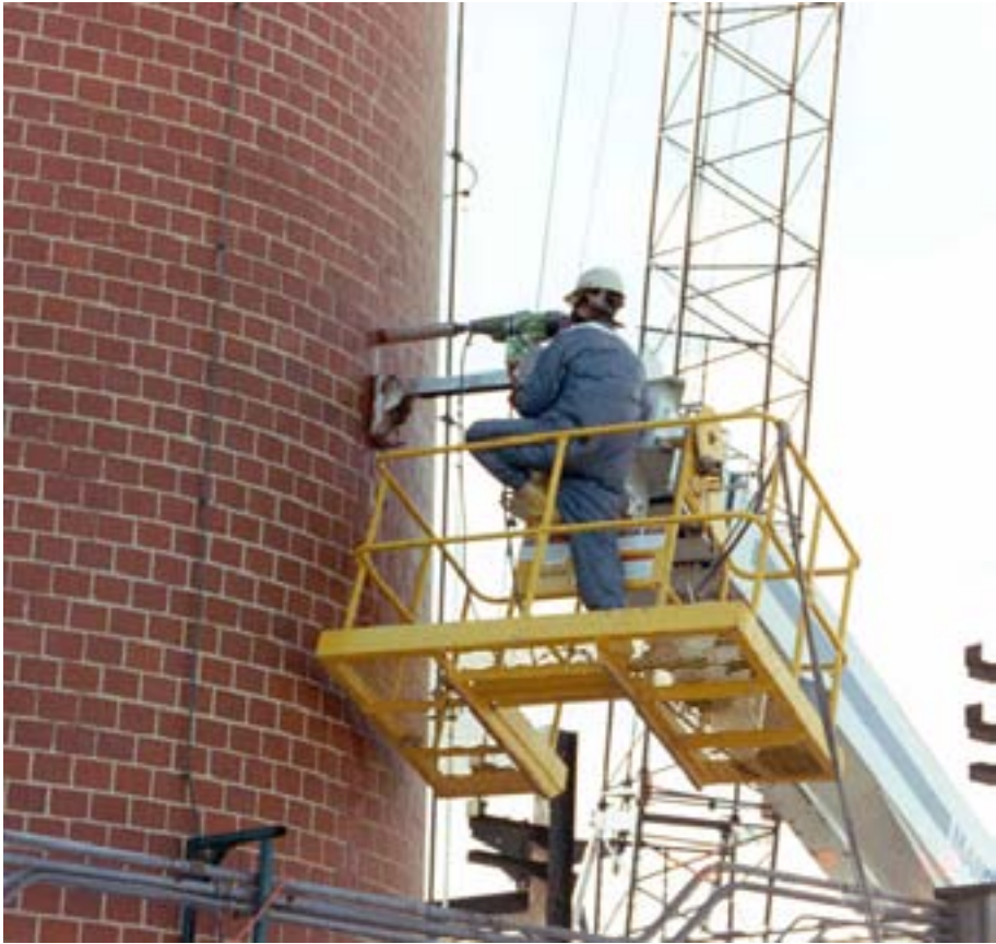
FIG. 6. Mound facility, USA. Stack core drilling at 20 ft (6 m) level opposite ventilation entry port.
