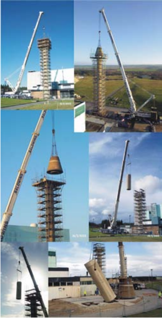
FIG. I.B-5. SGHWR stack decommissioning: lifting operations.
