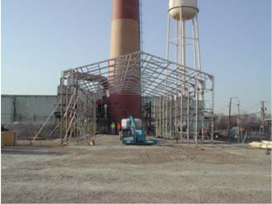
FIG. I.D-3. Fabrication of airlock.
