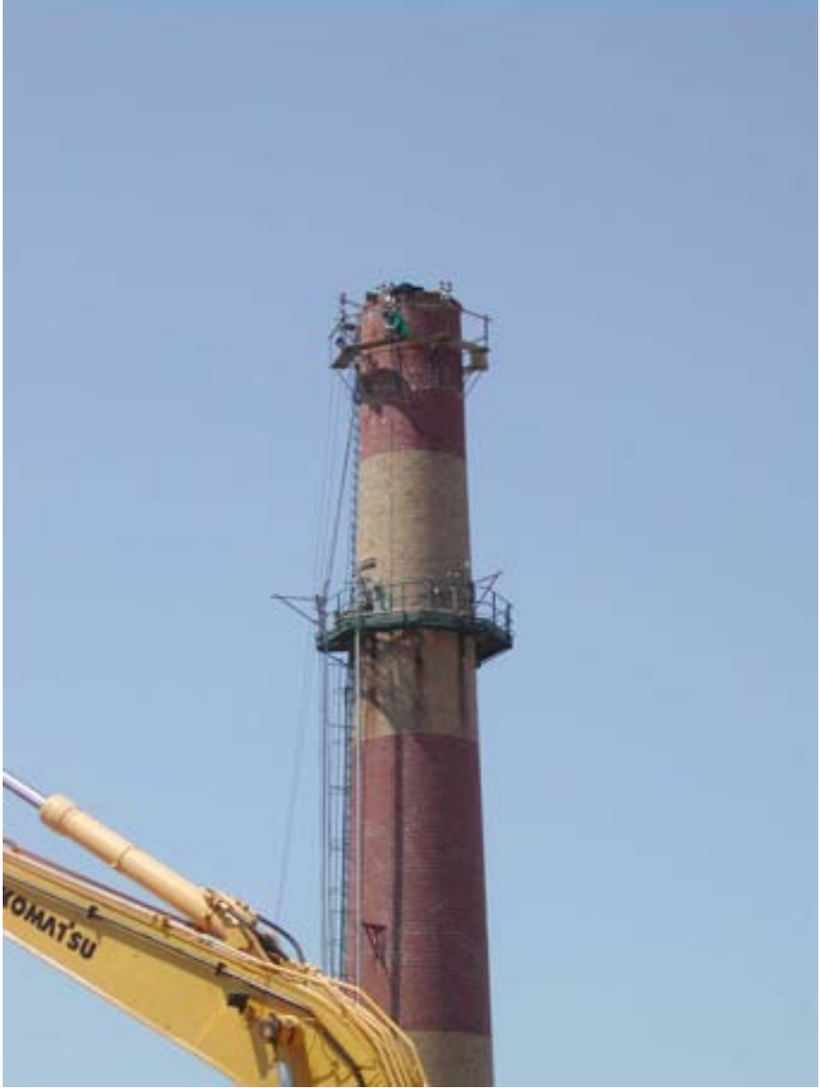
FIG. 18. Mound facility, USA. Top-down breaking of a brick stack.
