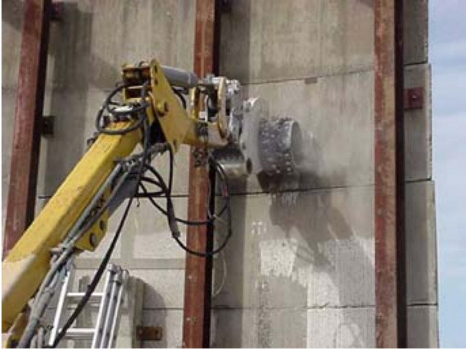
FIG. 7. Windscale Pile, United Kingdom. Adapted asphalt shaver.
