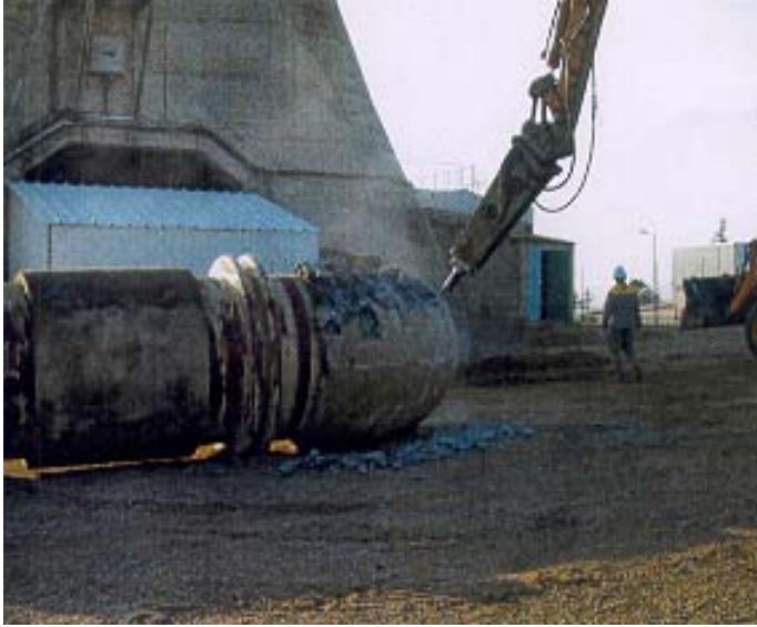
FIG. I.G-2. Removal of the ventilation piping.
