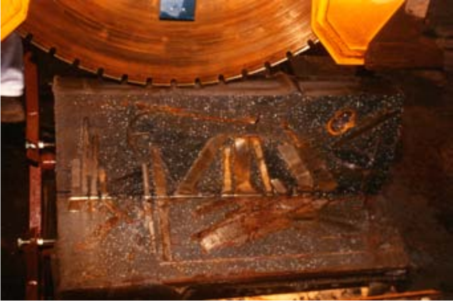
FIG. 13. Concrete cutting using a diamond tipped blade saw.
