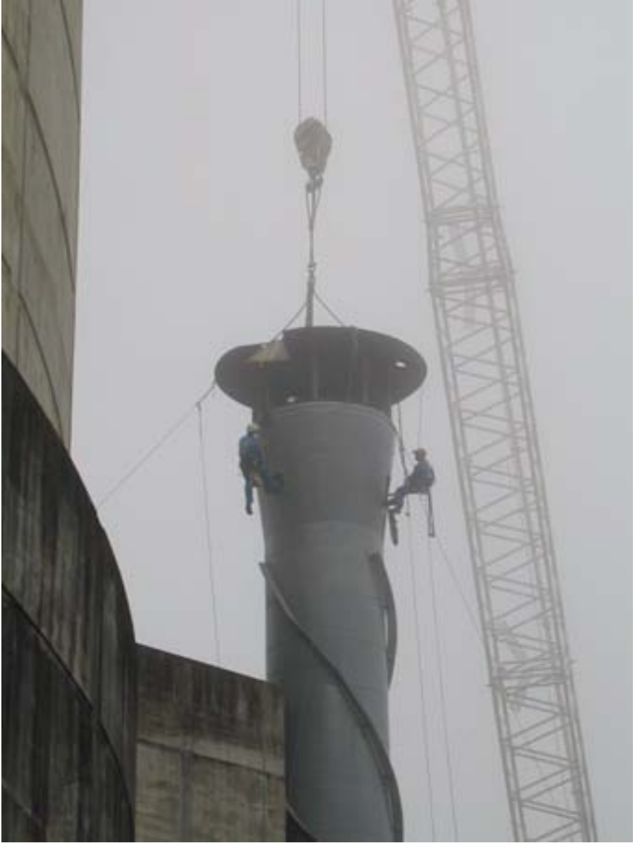
FIG. 15. Stack at Creys-Malville, France. Preparation for segmenting.
