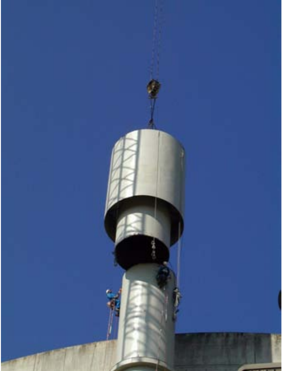
FIG. 14. Creys-Malville, France. Removal of stack segments.
