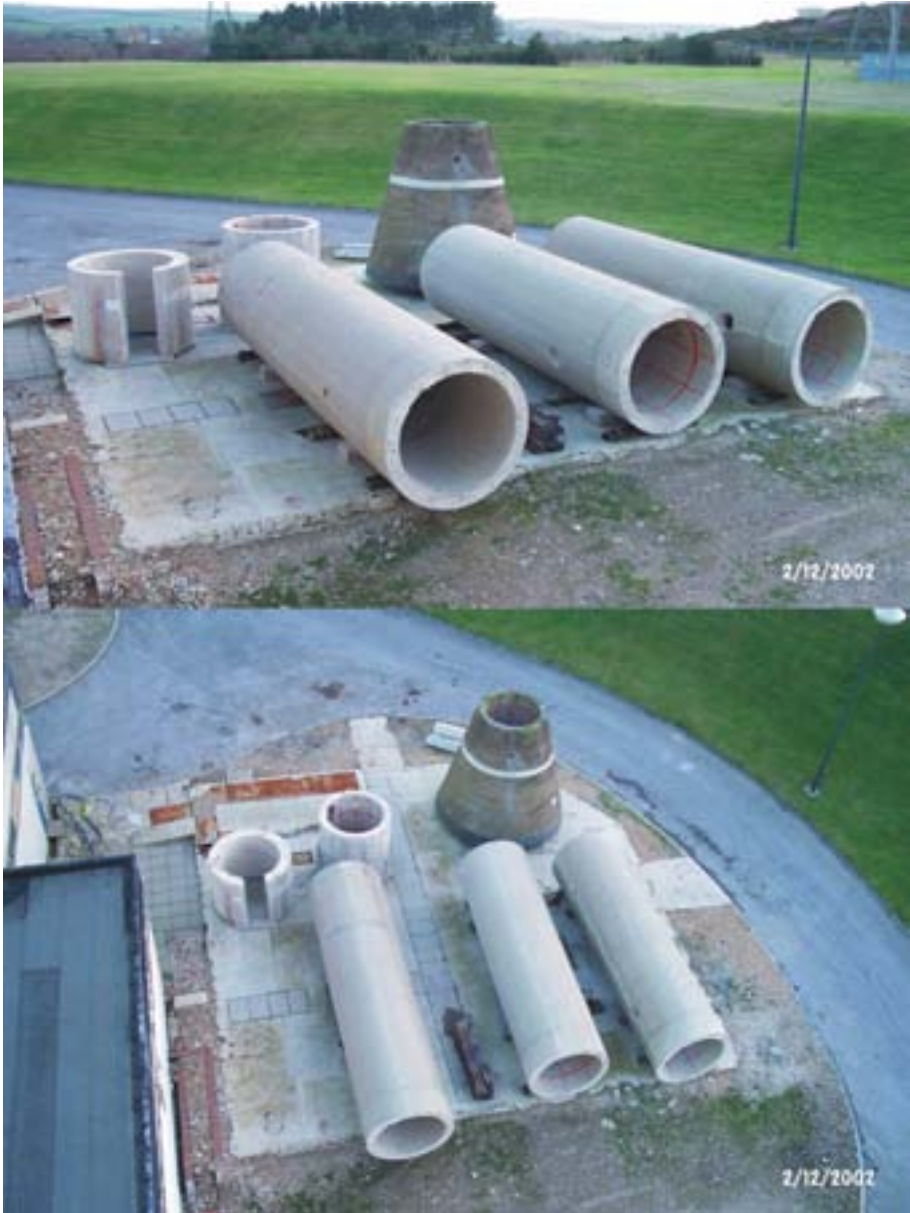
FIG. I.B-7. Views of decontaminated SGHWR stack sections after decommissioning.
