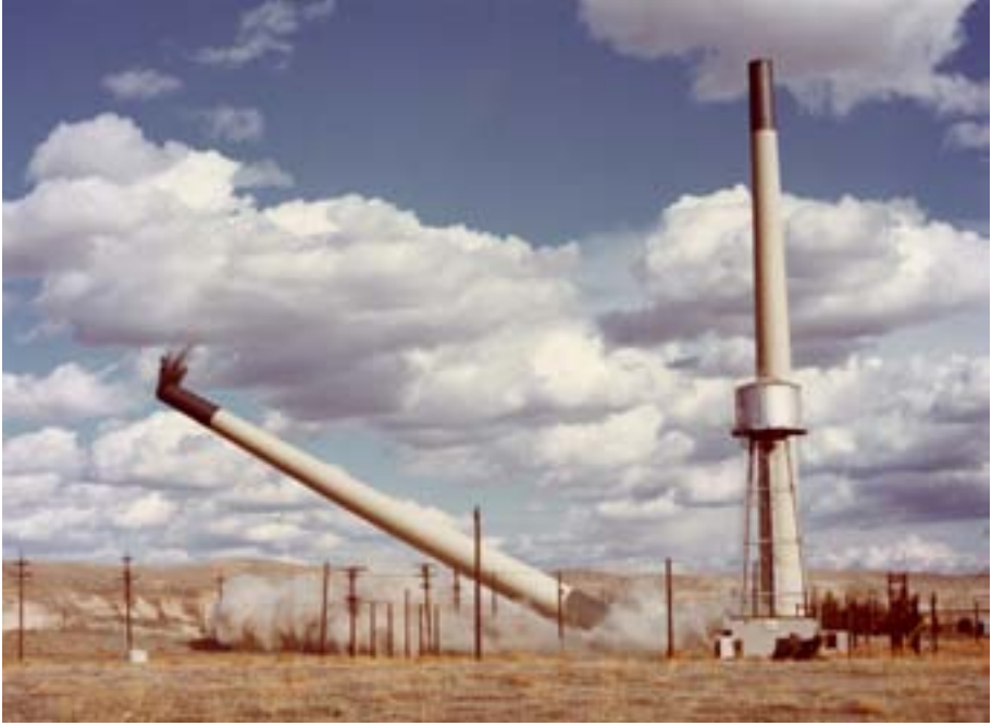
FIG. 21. Felling of the 110-F stack at Hanford, USA, using explosives.
