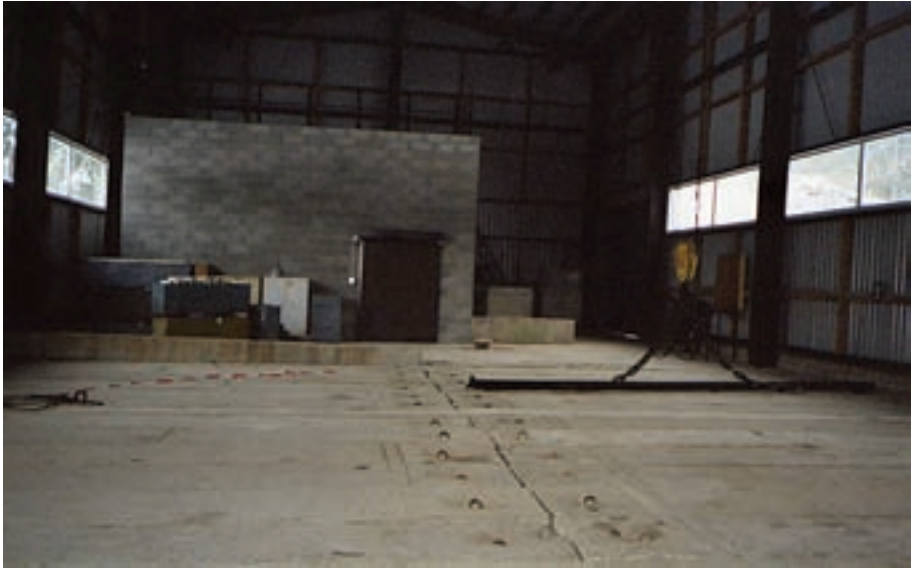
FIG. 29. The Baldone disposal facility, Latvia.
