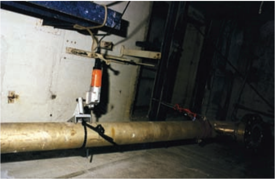
FIG. 18. Pipe sawing at the HDR project, Germany.
