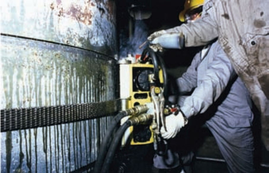
FIG. 19. Orbital sawing at the HDR project, Germany.
