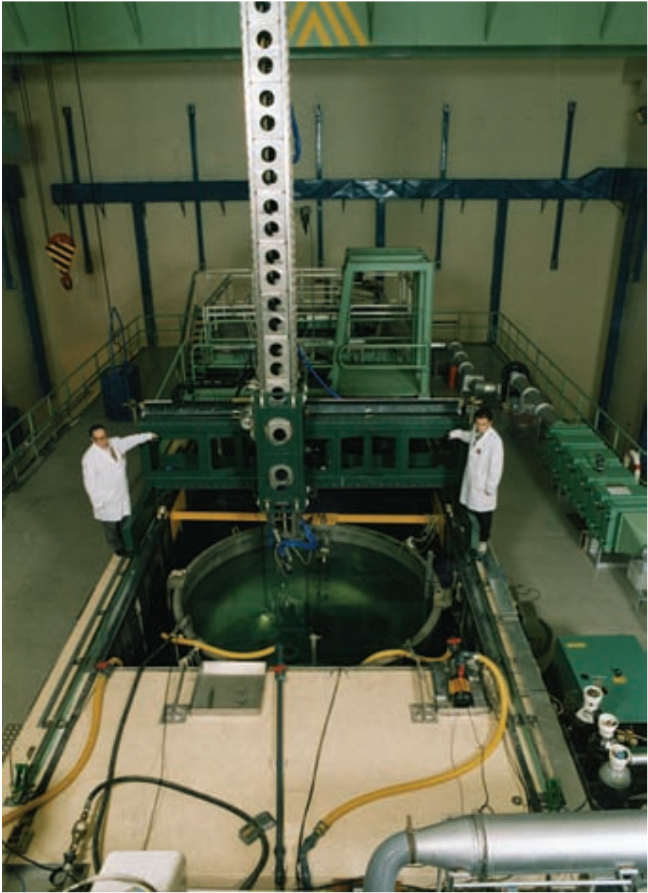
FIG. 9. JEN-1 decommissioning project, CIEMAT, Madrid, Spain: underwater cutting machine.
