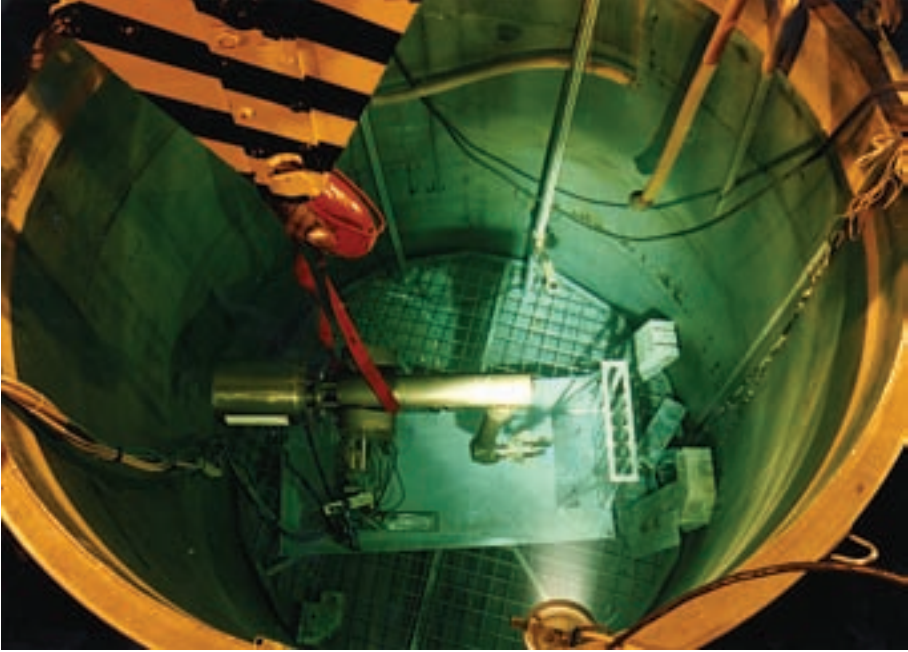
FIG. 22. JEN-1 decommissioning project, Spain: robotic manipulator.
