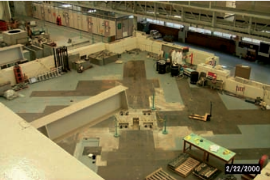
FIG. 1. The NESTOR reactor, Winfrith, UK (a) before and (b) after decommissioning.
