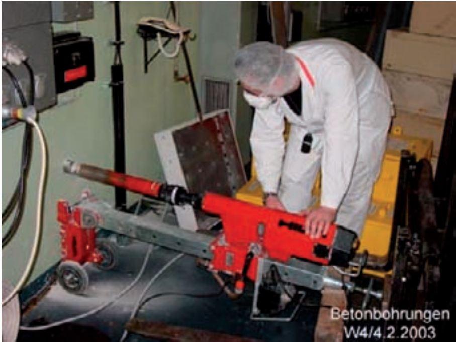
FIG. 28. Concrete core drilling device, ASTRA reactor, Austria.
