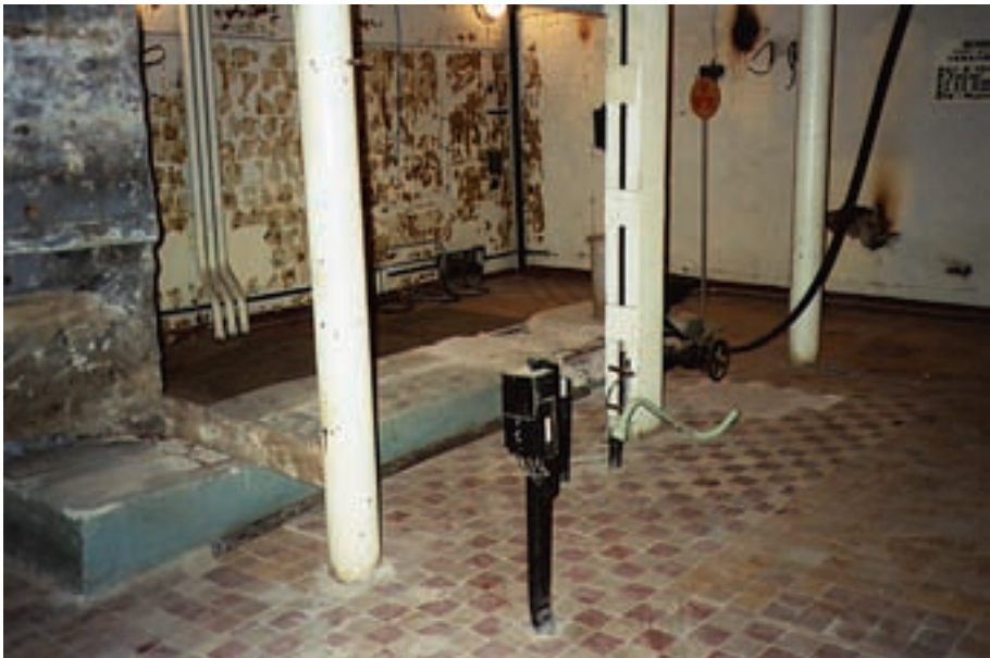
FIG. 3. The TVR reactor, Moscow: basement after dismantling of the cooling circuit.
