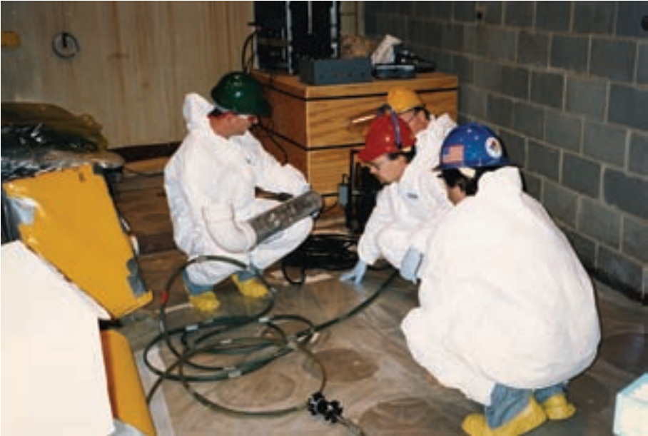
FIG. 27. Pipe crawler characterization technology being 'checked out' prior to demonstration at the CP-5 facility (source: Argonne National Laboratory, USA, contract no. W-31-109-ENG-38).
