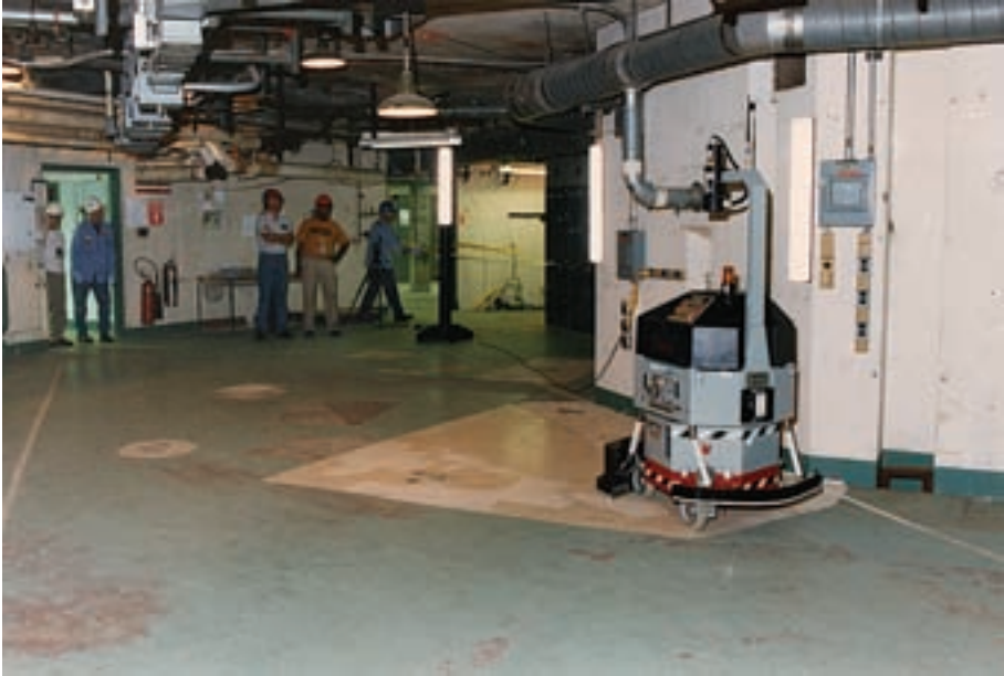
FIG. 26. The MACS being used at CP-5 for radiological characterization (source: Argonne National Laboratory, USA, contract no. W-31 109 ENG 38).
