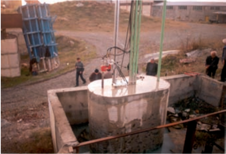
FIG. 15. Mock-up facility to test the IRT-M reactor grouting, Georgia.
