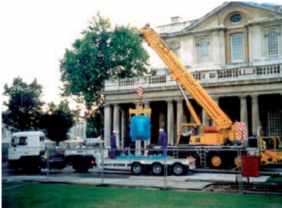
FIG. 4. Spent fuel removal from the JASON reactor, UK.
