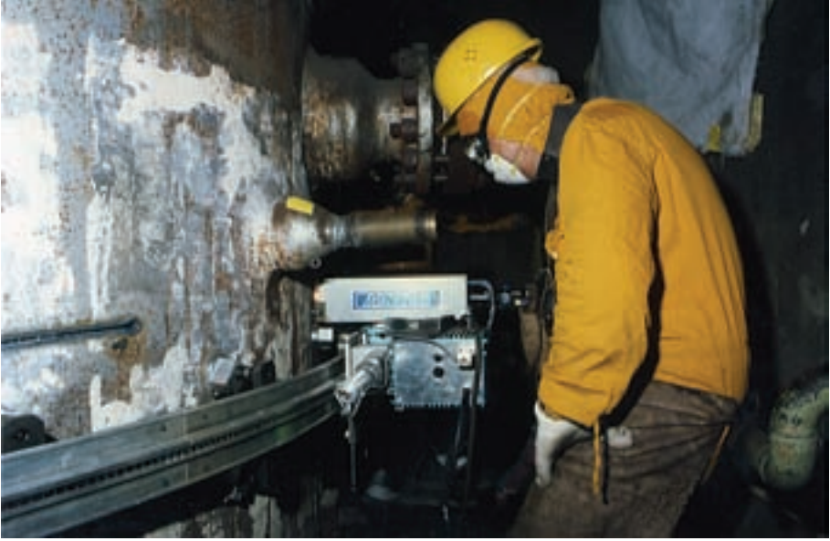
FIG. 17. Thermal dismantling at the HDR project, Germany.
