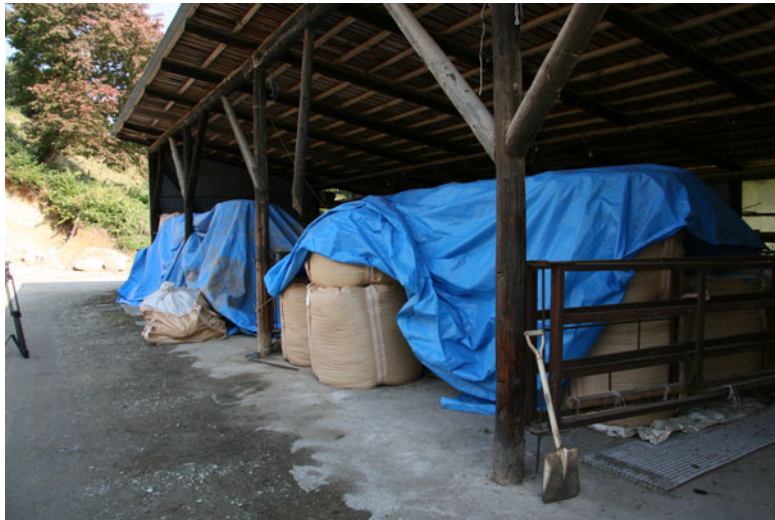
Fig. F.8. Temporary storage for removed topsoil from a paddy field at a demonstration site in Iitate Village (IAEA, 2011b).
