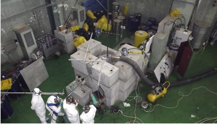
Fig. 11.8 Plasma cutting of reactor core in a shielded cell. Courtesy of C. Dragolici.
