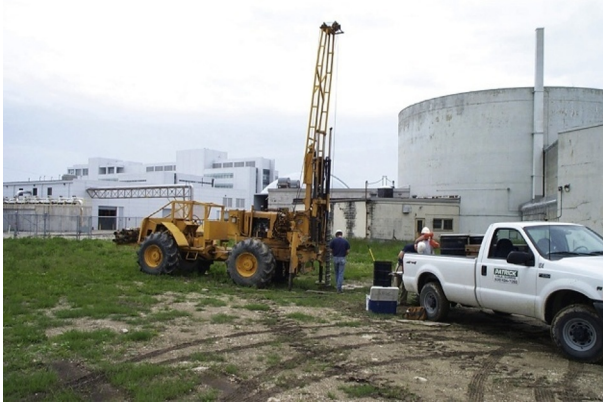
Fig. 13.4 Site characterization around B330 at ANL's Chicago site. From Larry Moos, Argonne National Laboratory.
