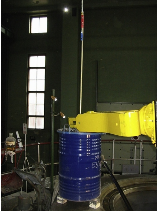
Fig. 11.9 Cutting the automatic regulation rod. Courtesy of C. Dragolici.
