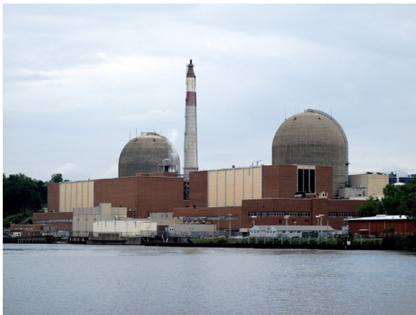
Fig. 12.3 Indian Point Unit 2 & 3 (Unit 1 invisible in this photo).
