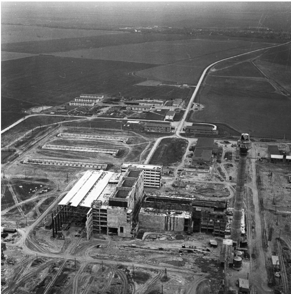
Fig. 9.10 The A1 NPP during the construction.
