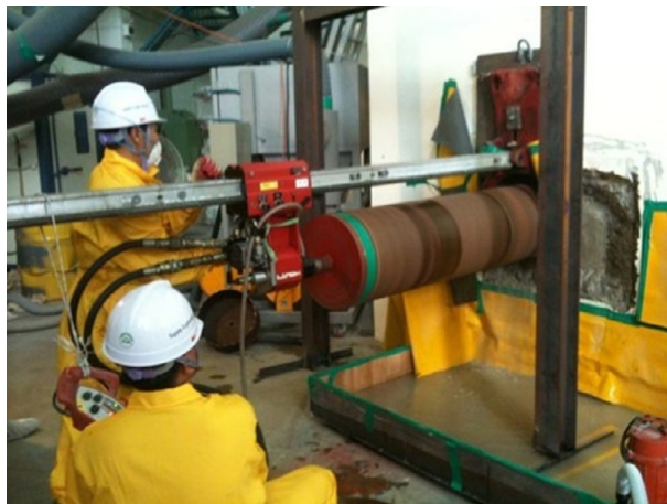
Fig. 11.6 Core drilling. Courtesy of S.-K. Park.
