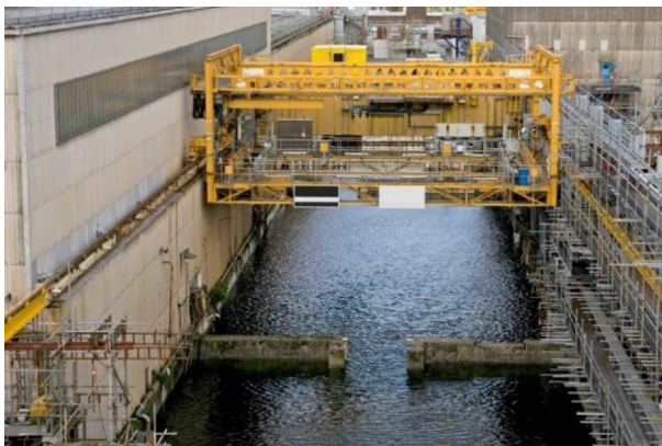
First generation Magnox fuel storage pond.
