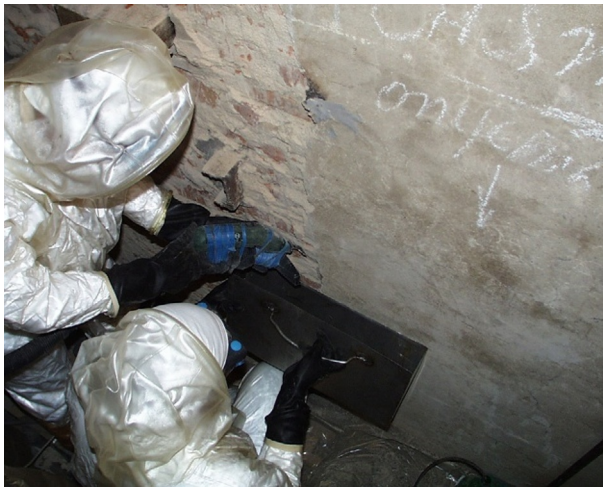
Fig. 6.4 Demolition of contaminated plaster.
