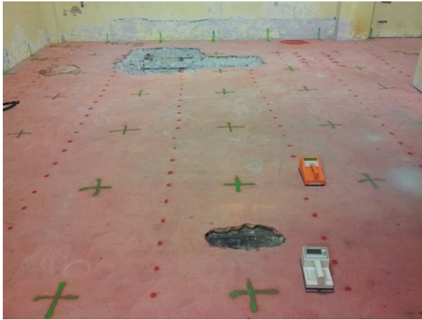
Fig. 10.2 Development of a measurement mesh for the purpose of building a final radiological survey.
