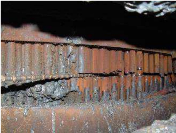
Fig. 8.31 Rancho Seco Steam Generator Diamond Wire Cut [154].
