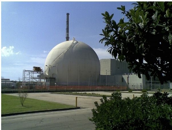
Fig. 1.2 Garigliano NPP: the spherical reactor building with the stack in the background. Photo by M. Lاراia, 1980s.
