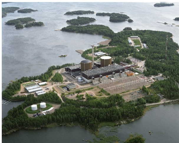
Fig. 12.6 Bird's-eye view of Loviisa NPP's two reactors.
