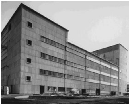
3.17 The MAGNOX reprocessing plant at Sellafield, UK. Source: Nuclear Decommissioning Authority (“NDA”), copyright: Nuclear Decommissioning Authority (“NDA”).
