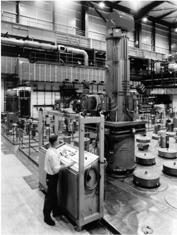
3.7 Remote replacement of an EARP ultrafilter module. Source: Nuclear Decommissioning Authority (“NDA”), copyright: Nuclear Decommissioning Authority (“NDA”).
