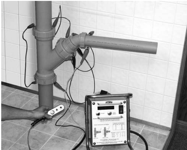
Figure 2-13 Fusion Lock Process in Operation
