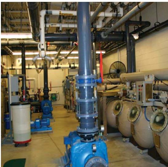
Figure 6-7 Horizontal High-rate Sand Filtration System, Multi-tank
