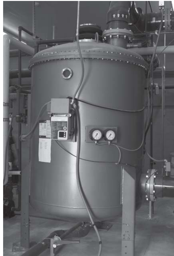
Figure 6-9 Regenerative DE Filter
