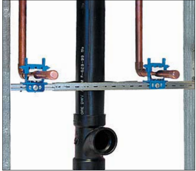
Figure 12-12 Appropriate Dissimilar Metal Isolation
