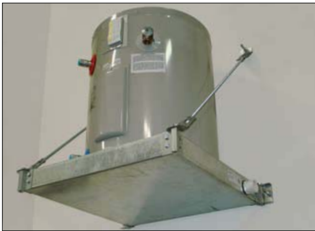
Figure 12-17 Engineered Wall-hung Equipment Platform
