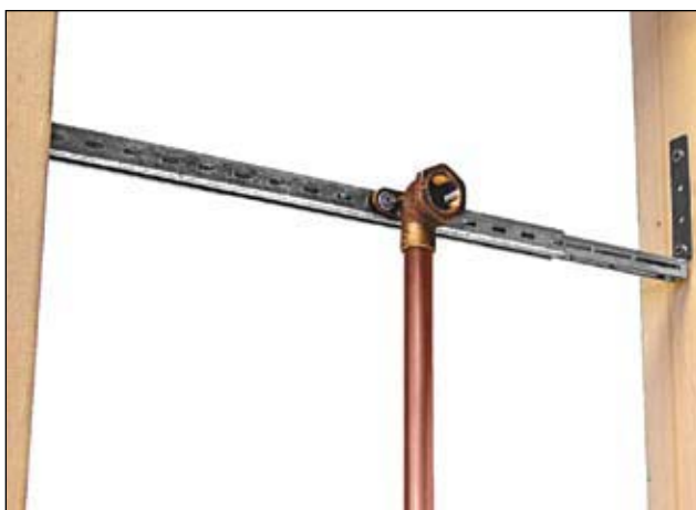
Figure 12-10 Shower Head Rough-in (Engineered)
