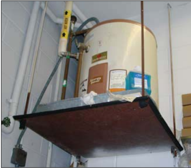
Figure 12-15 Makeshift Suspended Equipment Platform
