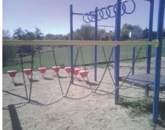
Figure 9.7 Playground equipment with potential for straddle injury (chain-link tight-rope).
