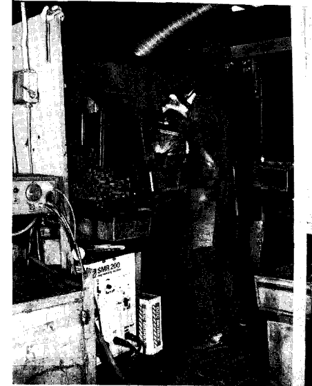
M.I.G. welding of small components in jigs. Note protective clothing - leather apron, gauntlets, strong boots - and safety aids such as fume extraction.
