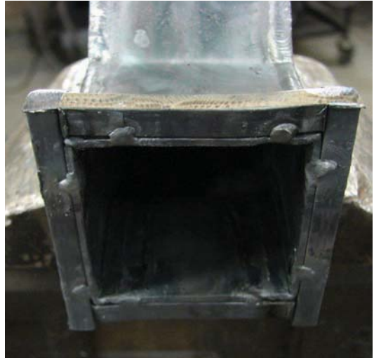
Figure 7-37. Grind the ends flush.
