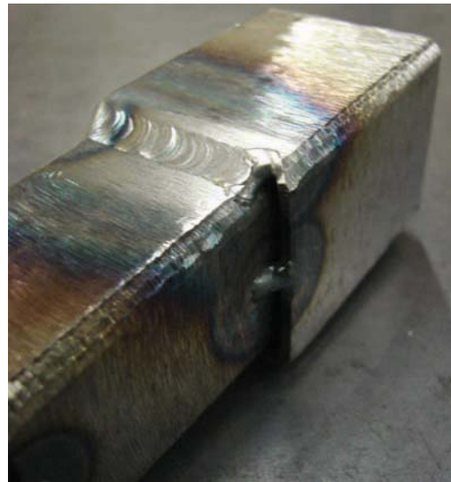
Figure 8-12. Lap welds completed on one side of the top and center tube. Make sure to end the weld by lapping around the corner, which will make it easier to proceed to the next weld.
