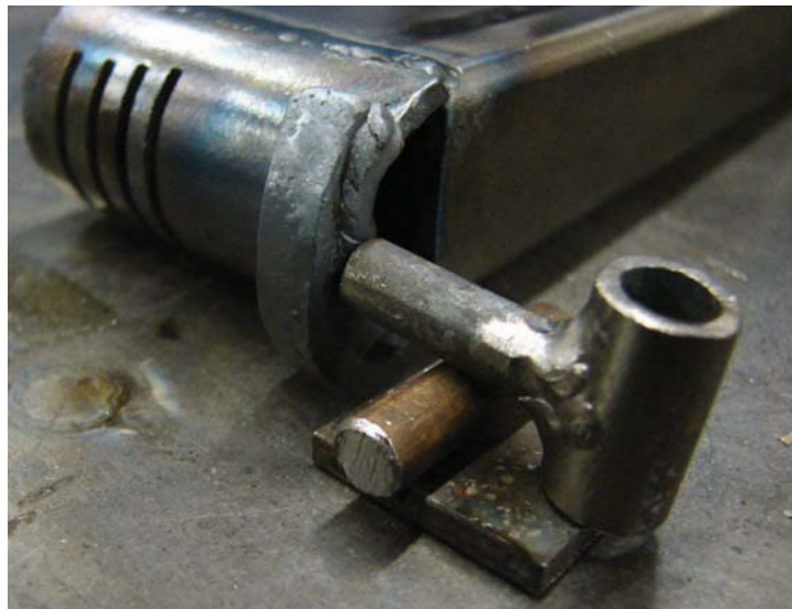
Figure 9-40. The axle parts supported and ready to be welded to the bumper. Observe that the main body of the tractor is laying flush on the table without any supports. This is achieved by hanging the seat base off the edge of the work table.
