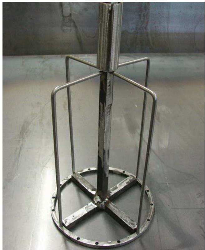
Figure 12-23. Preparing to weld the spokes to the spout and bottom outside ring.
