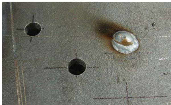
Figure 11-9. Completed plug weld.
