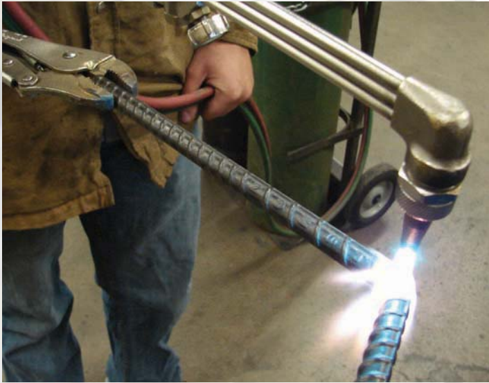
Figure 10-4. Bending the rebar base using a cutting torch.
