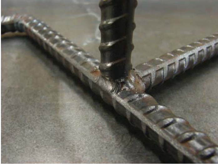
Figure 10-9. Completed welds around pole and base.
