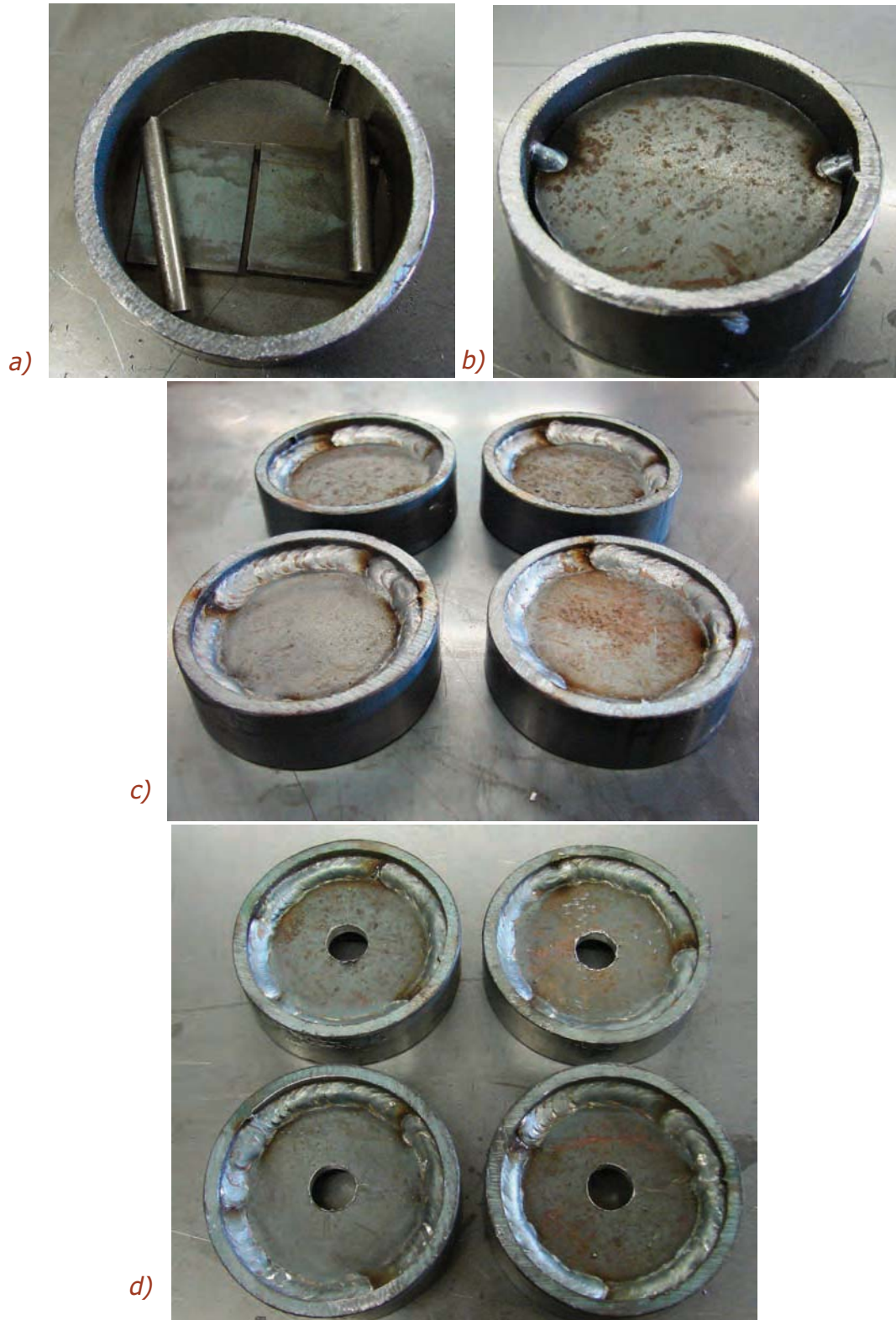
Figure 1-34. a) Use 1/8" flat bar and 3/16" rod for shims to place the wheel center in the right location. b) Tack the wheel center to the outside wheel. c) Completed fillet welds around wheels. d) Completed wheels with holes for axle placement.
