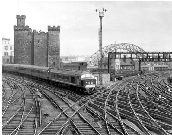
Figure 0.4 Railway crossing fabricated from manganese steel cast sections (courtesy of British Rail and Osborn-Hadfield Steel Founders Ltd.)
