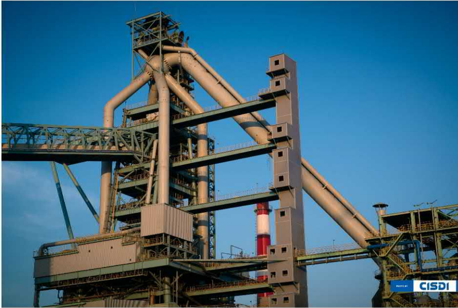
Blast Furnace in Baosteel Zhanjiang, China, Supplied by CISDI
