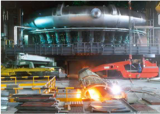
FIGURE 57.6 Typical flat casthouse floor. Note the hood manipulator on the right side of the photo and taphole drill and mud gun on the left side. Source: Photo courtesy of TMT—Tapping Measuring Technology S.à r. l & G.m.b.H.
