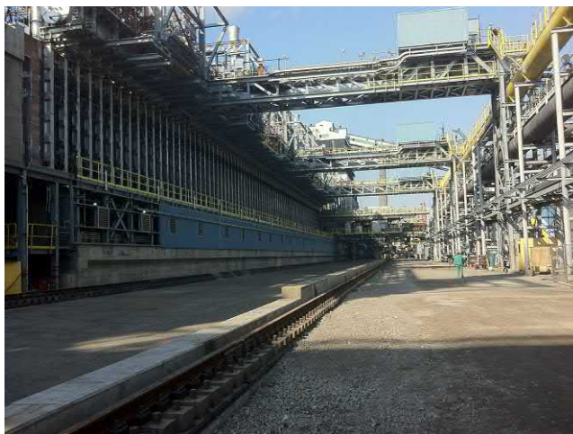
FIGURE 55.6 View of the pusher side of a typical 6-m by-product coke oven battery. Note that the coal storage bunker is in the background at the top of the inclined conveyor. Source: Photograph courtesy of thyssenkrupp Industrial Solutions AG.
