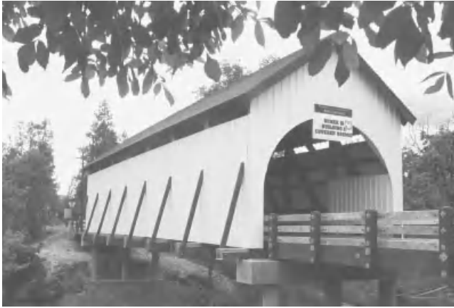
Figure 17.2.5-2 88-ft covered vehicular bridge. (Photo courtesy of Western Wood Structures, Inc., Tualatin, Oregon)
