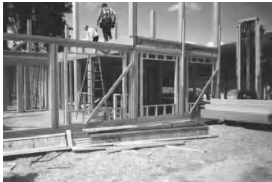
Figure 1.3.1-1 Post and beam construction.
