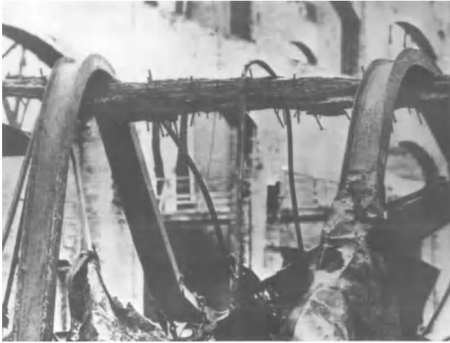
Figure 20.5-3 Nail-laminated 12" × 16" timber beam maintained integrity while steel girders collapsed.
