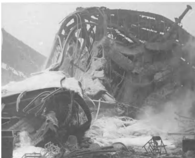
Figure 20.3.1-1 Noncombustible structure collapsed after 30 to 45 minutes of fire exposure at McCormick Place.
