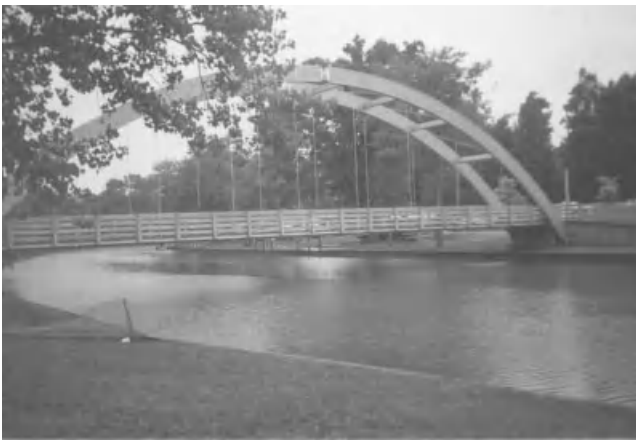
Figure 17.2.6-2 Glulam through-arch bridge.
