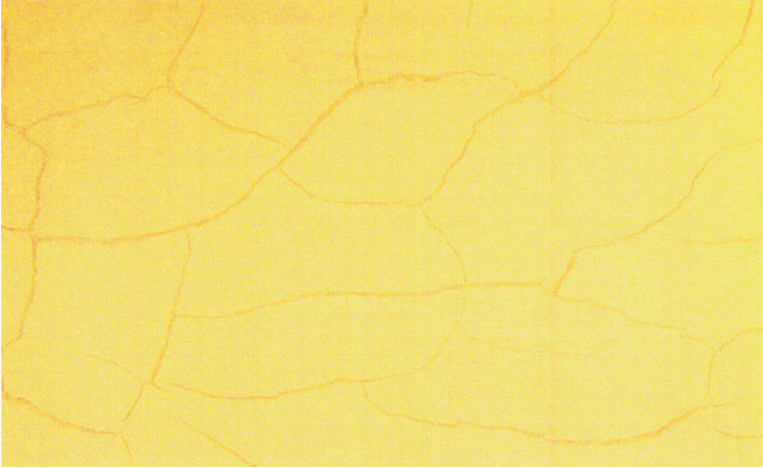
Fig. 4.72 Earth plaster with cracks after application [100]
