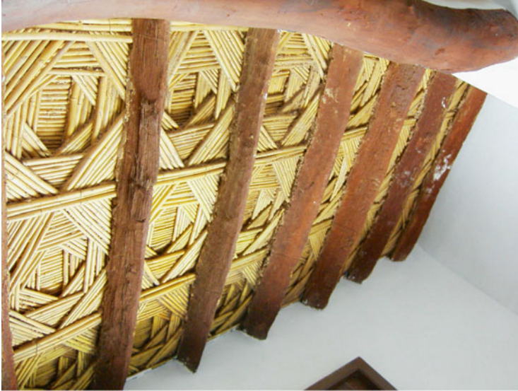
continuous bamboo sheathing to support puddled earth
