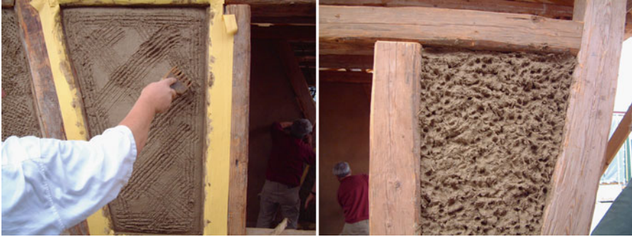
Fig. 4.69 Earth plaster, scratch and puncture patterns to roughen the substrate [51]
