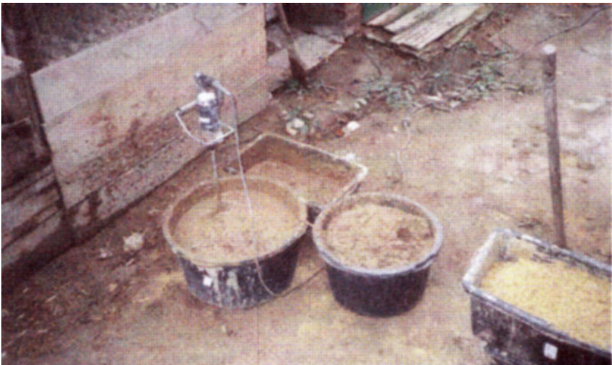
Fig. 6.2 Reuse of salvaged soil: soaking and adding sand [14]
