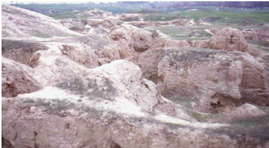
Fig. 1.12 Earth block walls in the city of Afrasiab, present-day Samarkand, Uzbekistan
