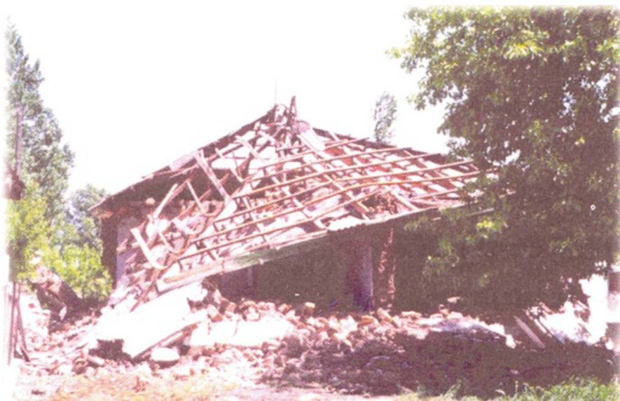
Fig. 5.38 Damage patterns after earthquake impact: destroyed building made of earth block masonry (Lugovaya, Kazakhstan, 2003) [45]
