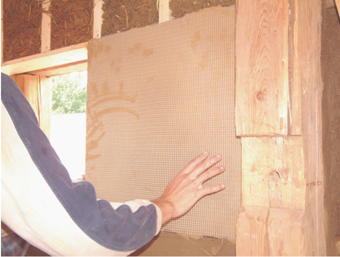
Fig. 4.71 Earth plaster, embedding reinforcement mesh into the wet base coat [51]
