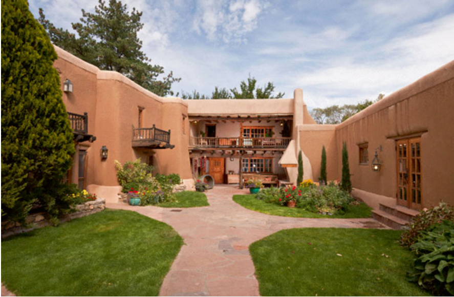
Fig. 4.9 Applegate Estate, residential adobe building in Santa Fe, NM, USA
