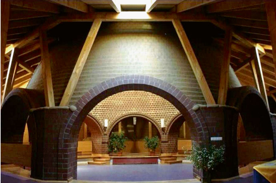
Fig. 4.10 Daycare facility Sorsum, Germany, earth block dome [1]
