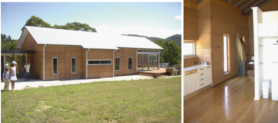
Fig. 4.4 Load-bearing rammed earth walls stabilized with cement
