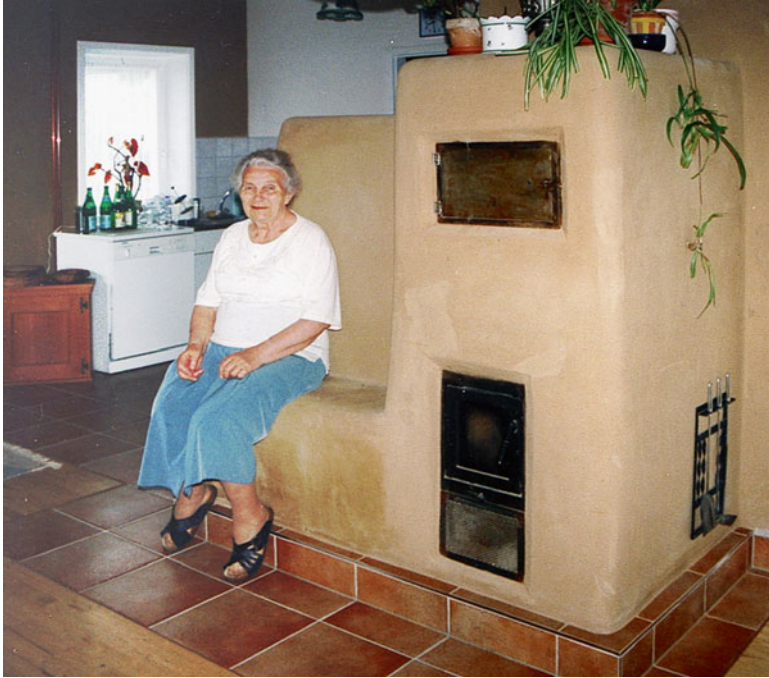
Fig. 4.80 Technical installations, earth masonry heater in the form of a standard wood-burning stove wrapped with a coat of high-mass earth [87]
