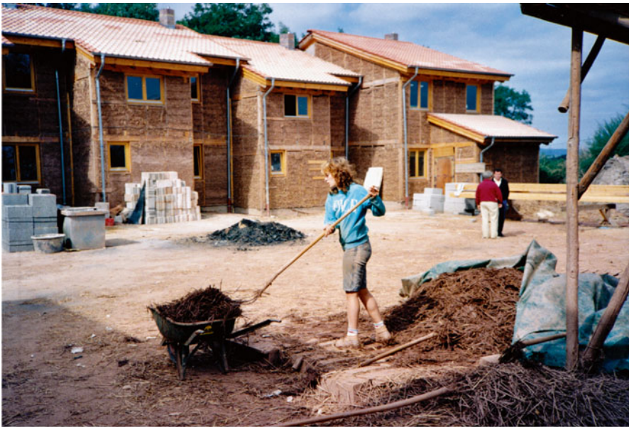
new residential construction in Saarbrücken-Bous/Germany, 1990
