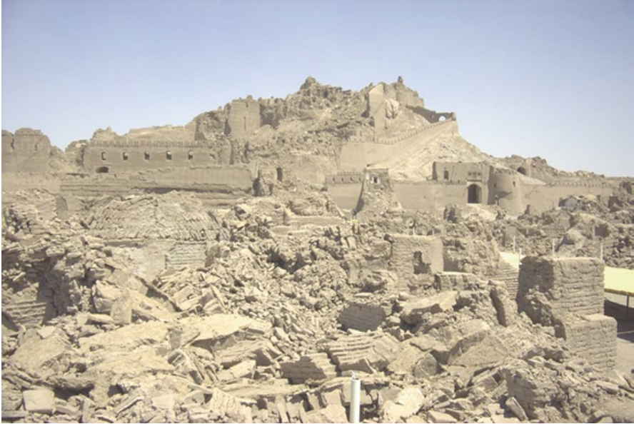
Fig. 5.41 Damage patterns after earthquake impact: destroyed structures employing traditional earth block and cob techniques (tschineh), Bam, Iran, 2003
