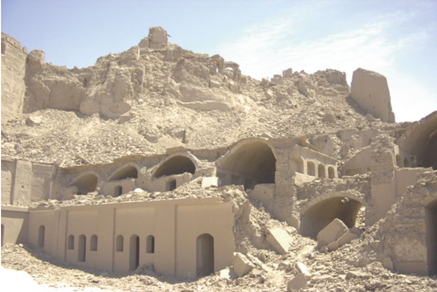
Fig. 5.33 Damage patterns after earthquake impacts: intact earth block vault structures, Bam, Iran, 2003
