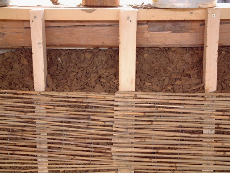
Fig. 3.20 Shaping of walls made of wood-chip light clay using permanent formwork [9]
