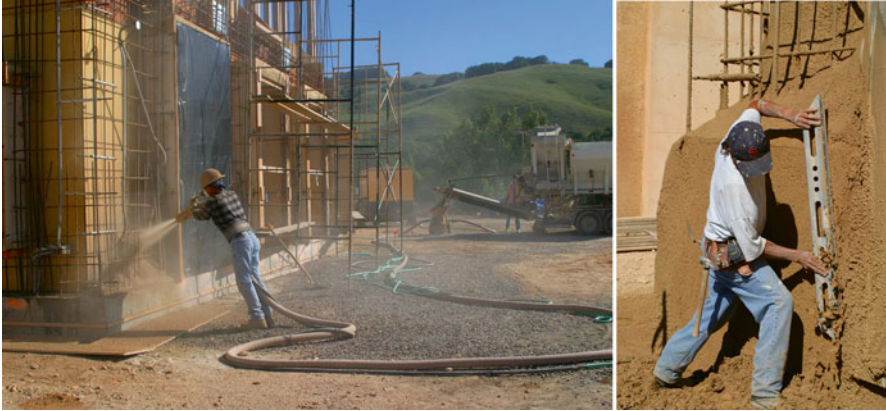
Fig. 4.32 Load-bearing walls made of sprayed earth with steel reinforcement [69]
