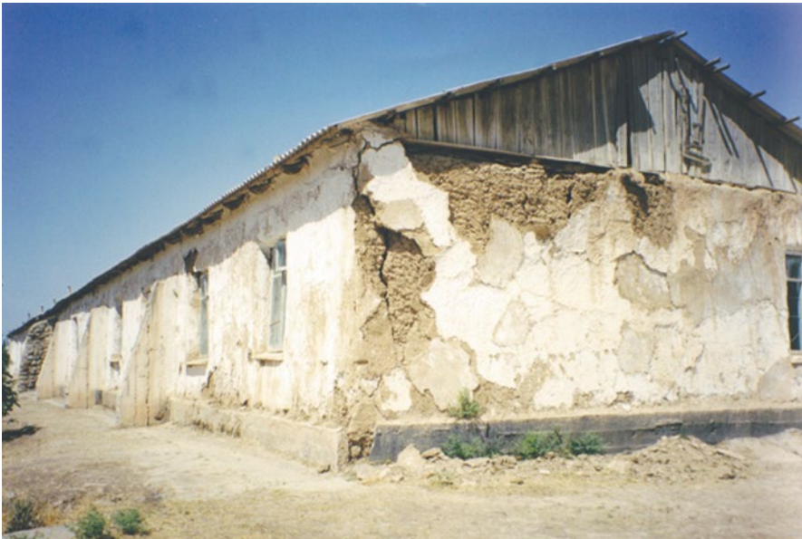
Fig. 5.69 Seismic retrofitting of earth buildings, reinforcement using buttresses: school building constructed in “pachsah” method in the Kamashi Region, Uzbekistan, after earthquake in the year 2000 [45]
