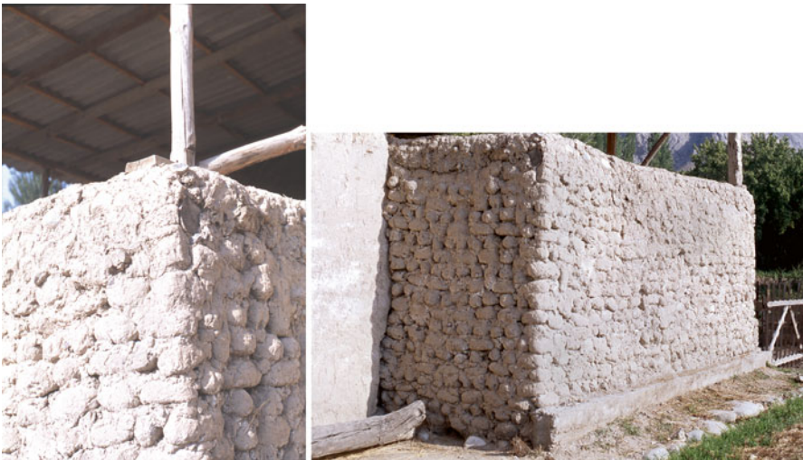
Fig. 4.37 Load-bearing wall construction using the guvalja technique
