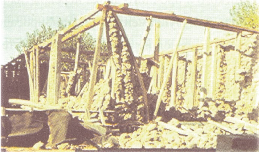
Fig. 5.39 Damage patterns after earthquake impact: destroyed residential building using half-timber construction with earth clump infill (sintsch) (Kairakkum, Tajikistan, 1985) [45]
