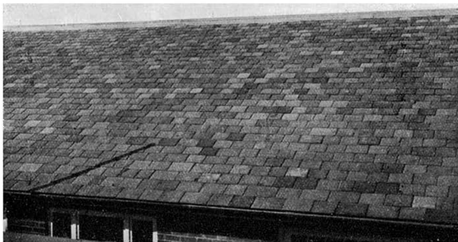
Fig. 3.—OLD DELABOLE SLATING—RANDOM SLATES LAID IN DIMINISHING COURSES
