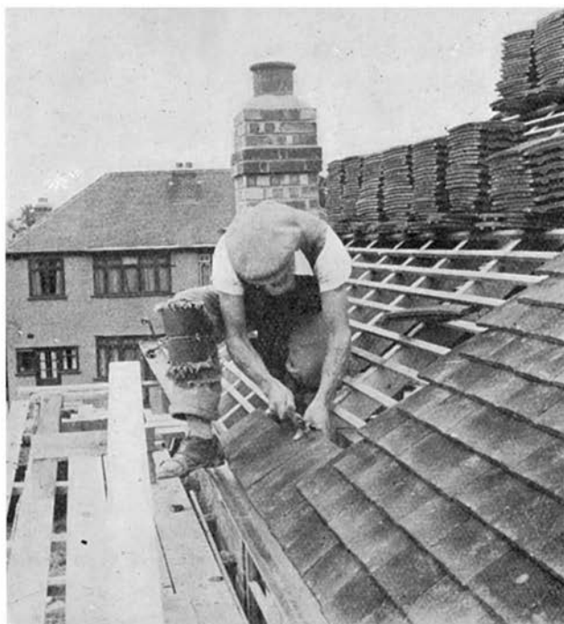
Fig. 13.—CONSTRUCTION AT EAVES IN PLAIN TILING
