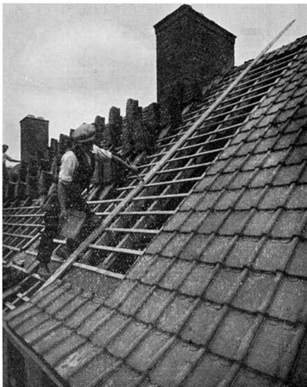
Fig. 24. —COURTRAI-DU-NORD TILING ON OPEN BATTENING
