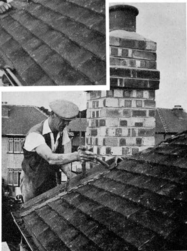
Figs. 15 and 16. —HIP COVERED WITH HALF-ROUND RIDGE
