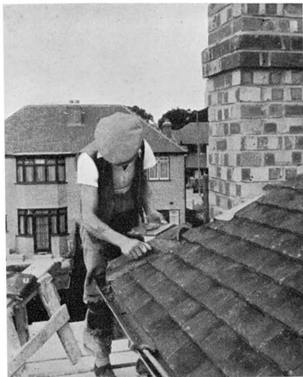
Figs. 15 and 16. —HIP COVERED WITH HALF-ROUND RIDGE
