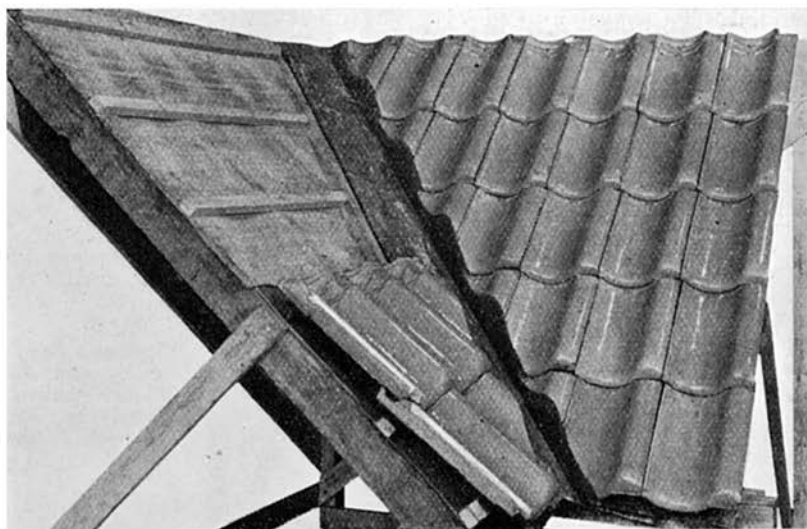
Fig. 27F.—STAGE 7—VALLEY NEARING COMPLETION—STRAIGHT-EDGE REMOVED ( Langley London Ltd. )
