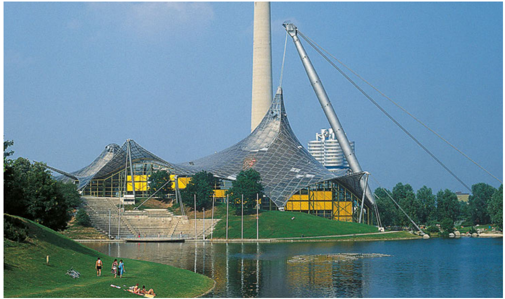
Entrance area, view from east
