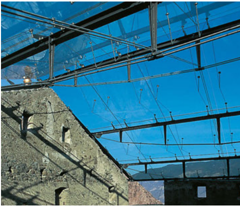
Underside of roof
