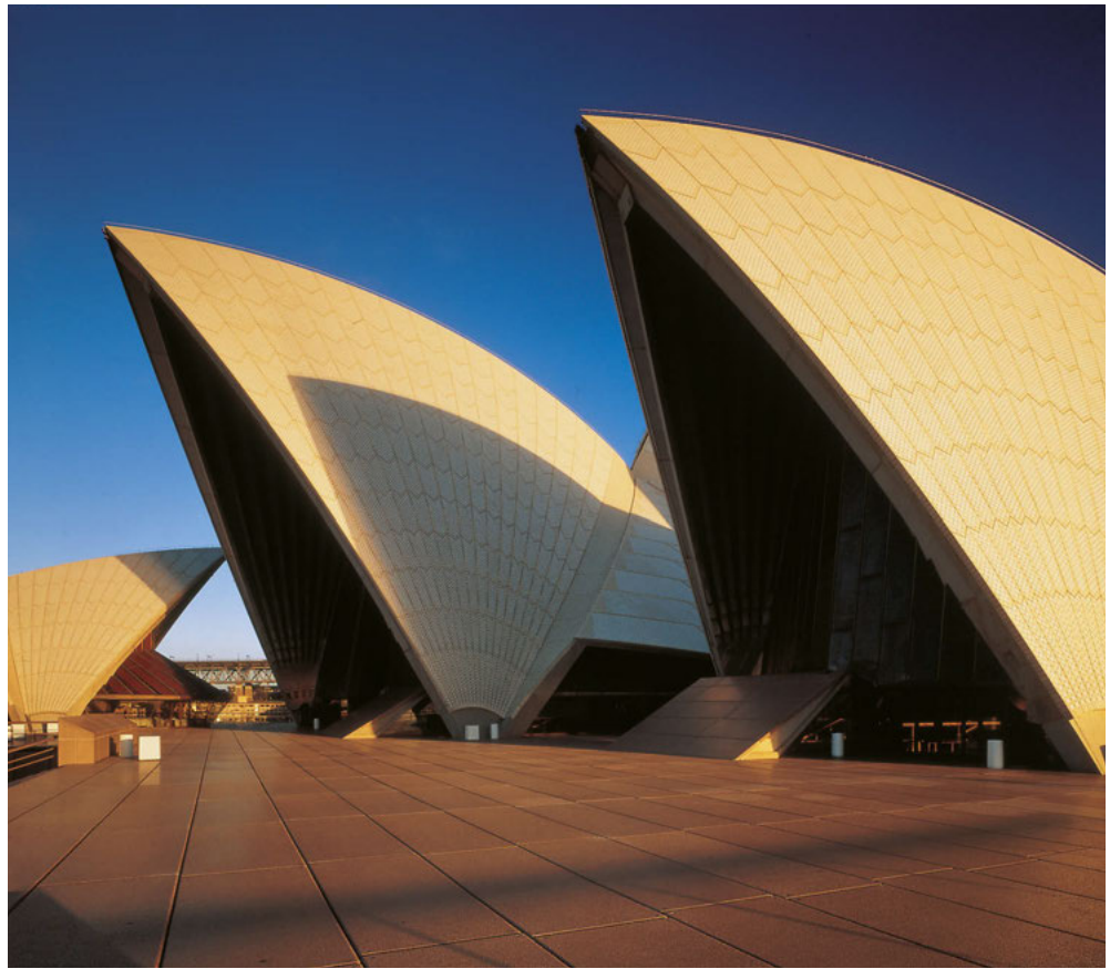
Harbour promenade, north side
