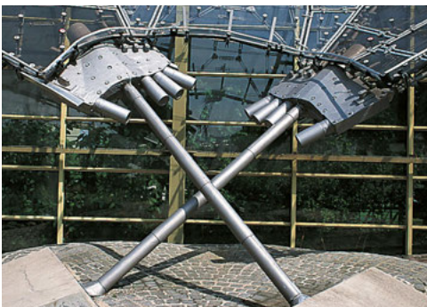
Eaves anchor point
