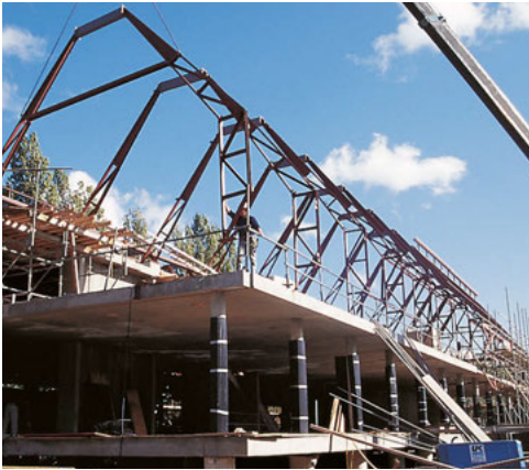
Steel truss roof frame
