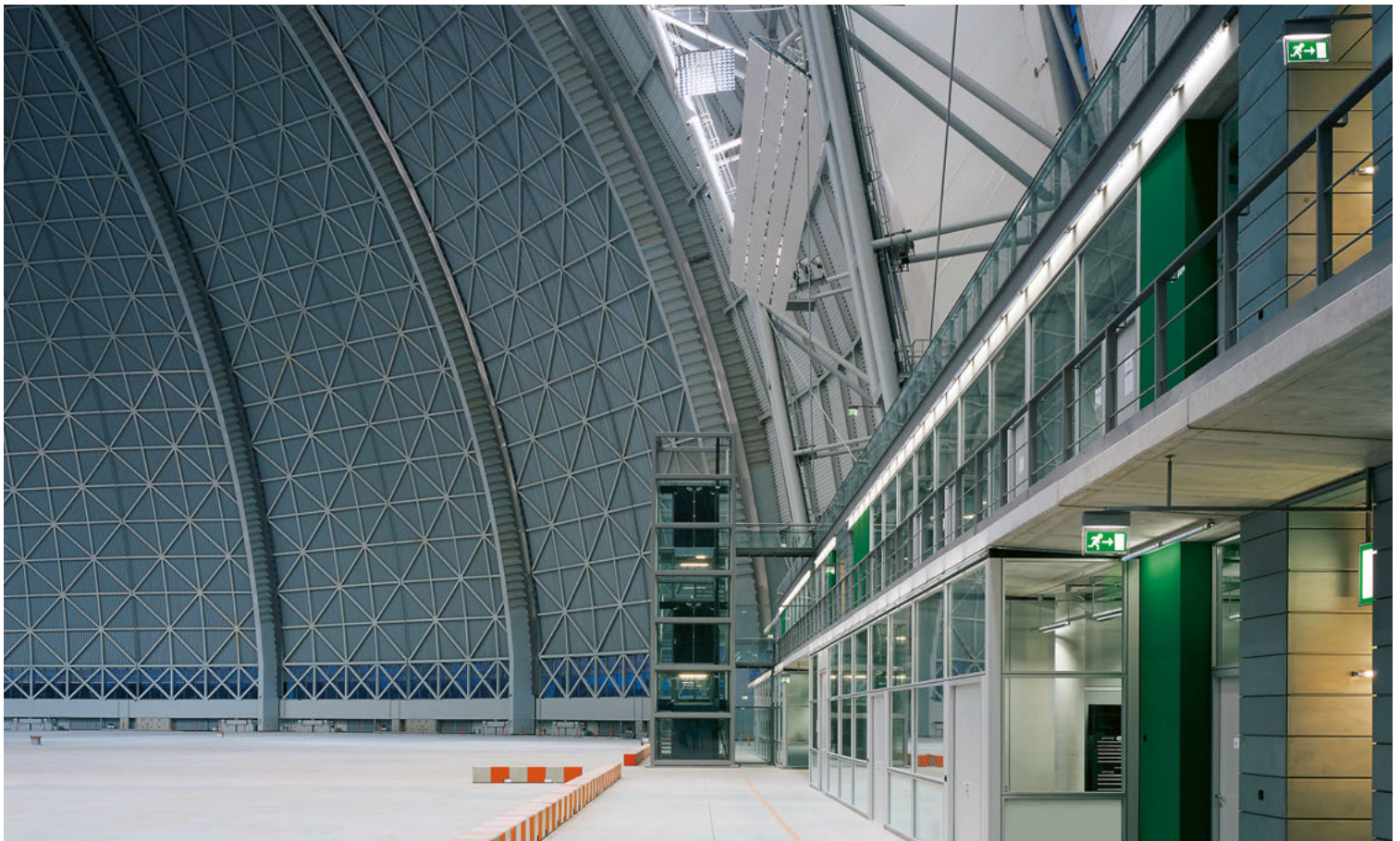
Glazed offices and rest areas in front of the opening gate
