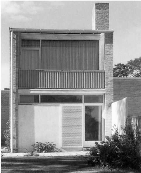
Balcony, projecting roof
