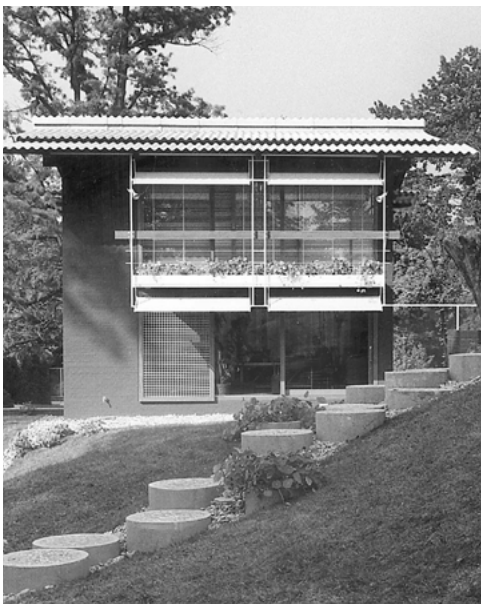
Projecting roofs of both houses
