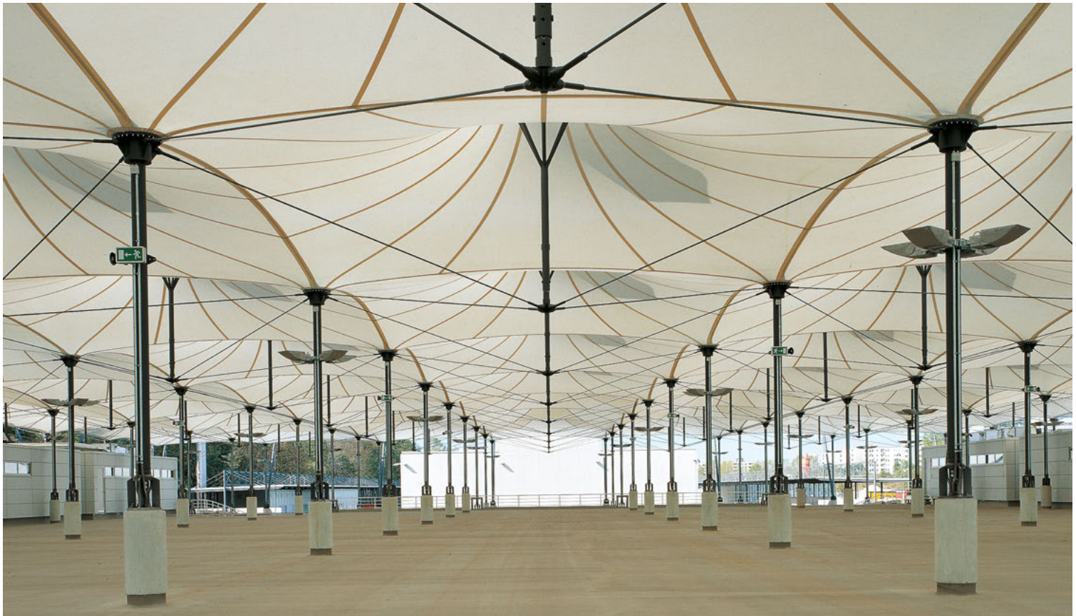
Underside of roof
