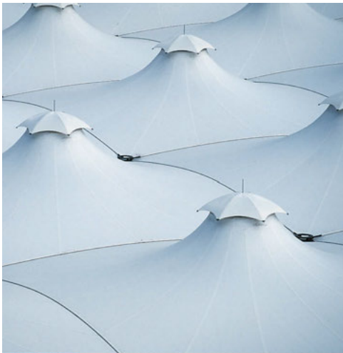
Top view of roof
