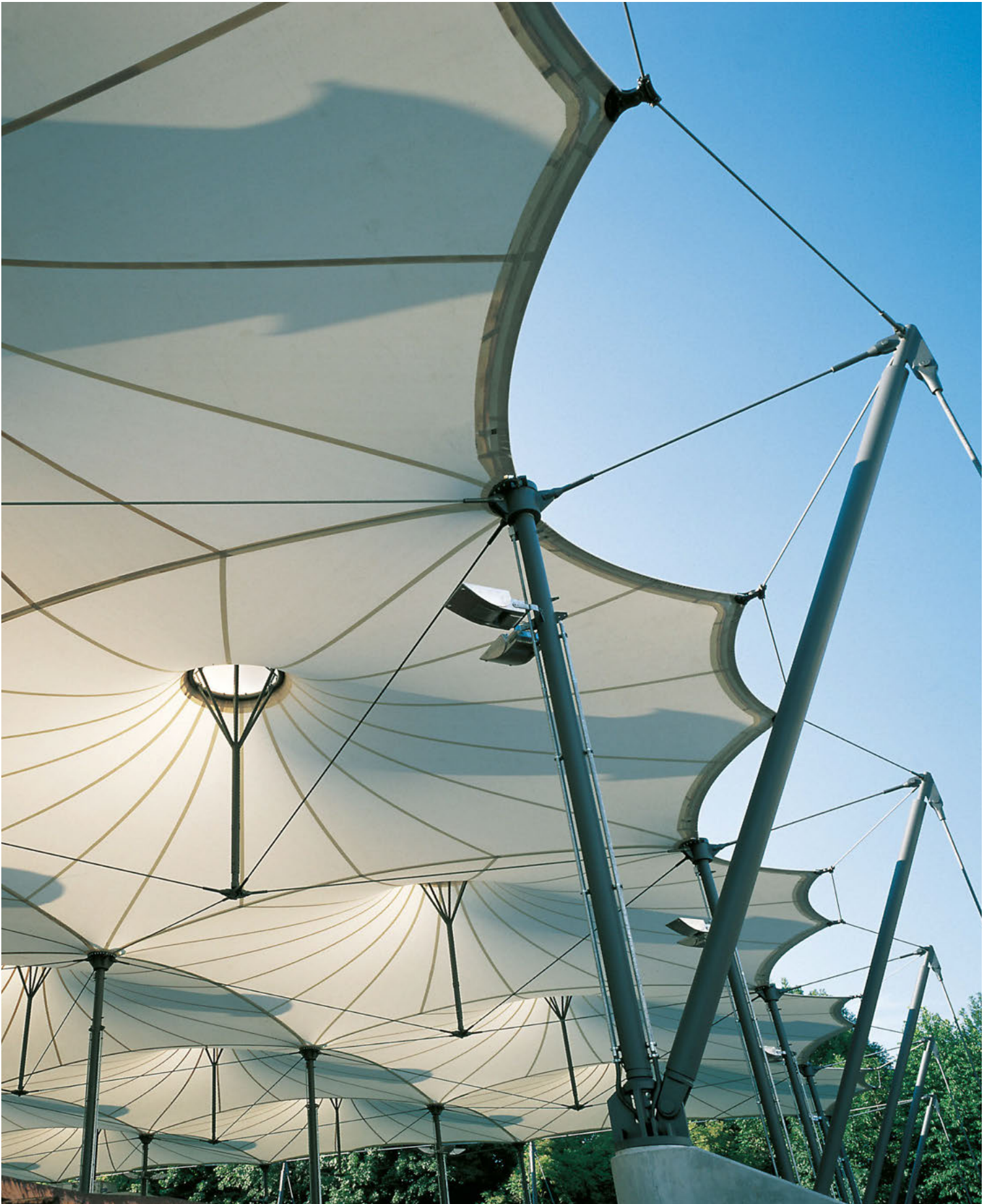
Edge column and underside of roof
