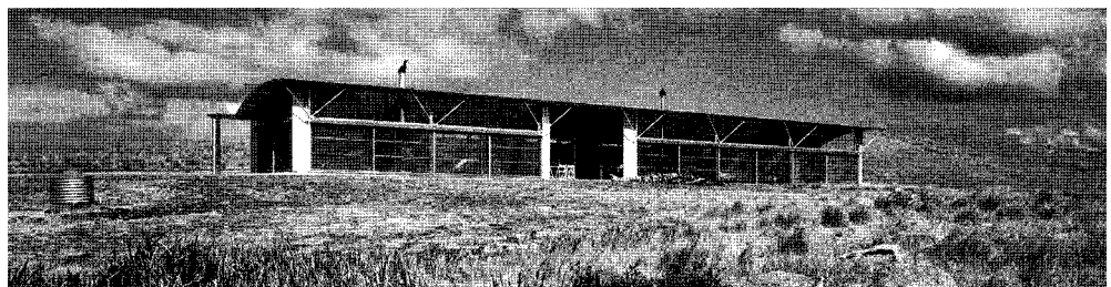
North side, terrace
