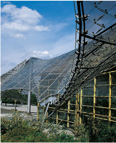
Swimming pool, view from south
