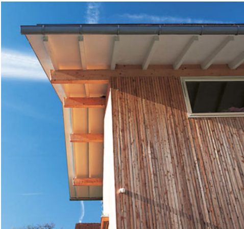
Gable overhang, south
