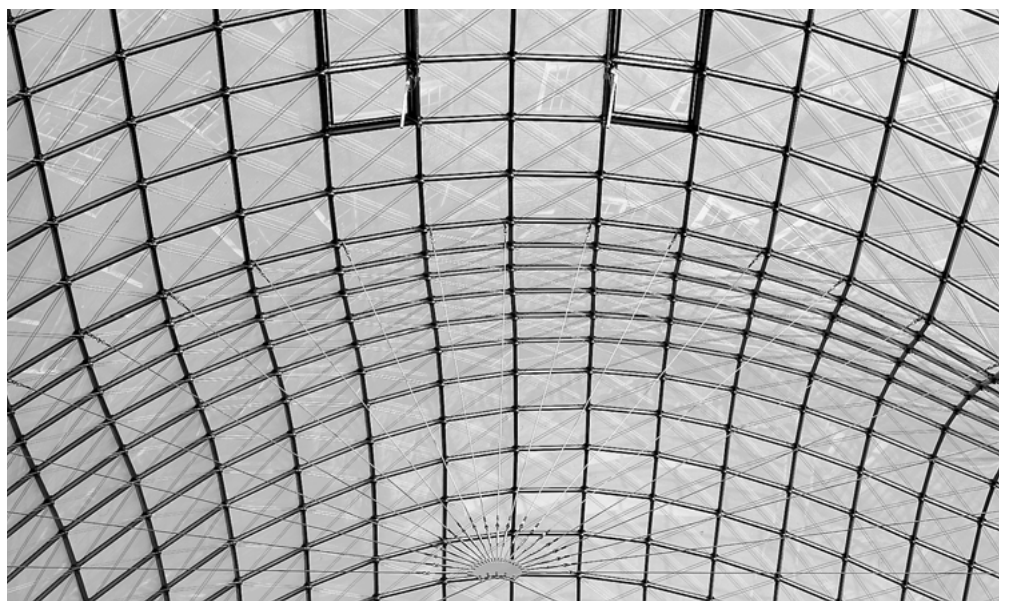
Underside of roof
