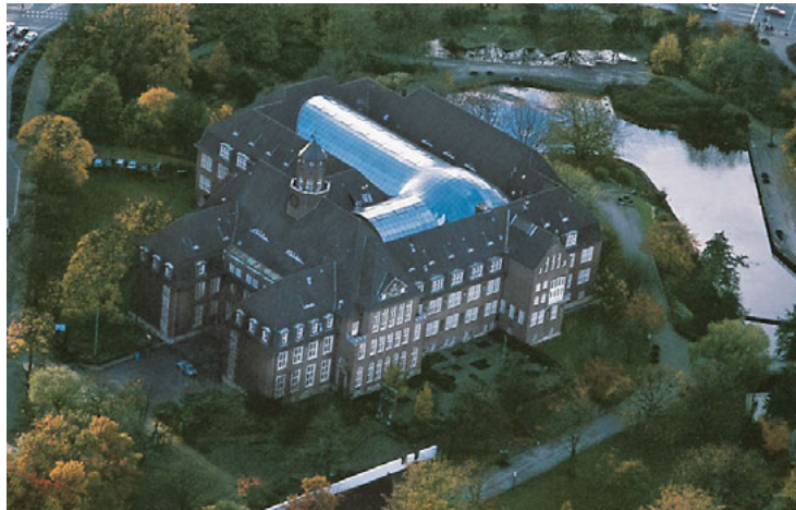
View of roof
