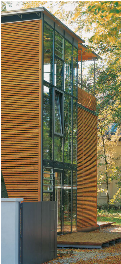
West-facing gable facade
