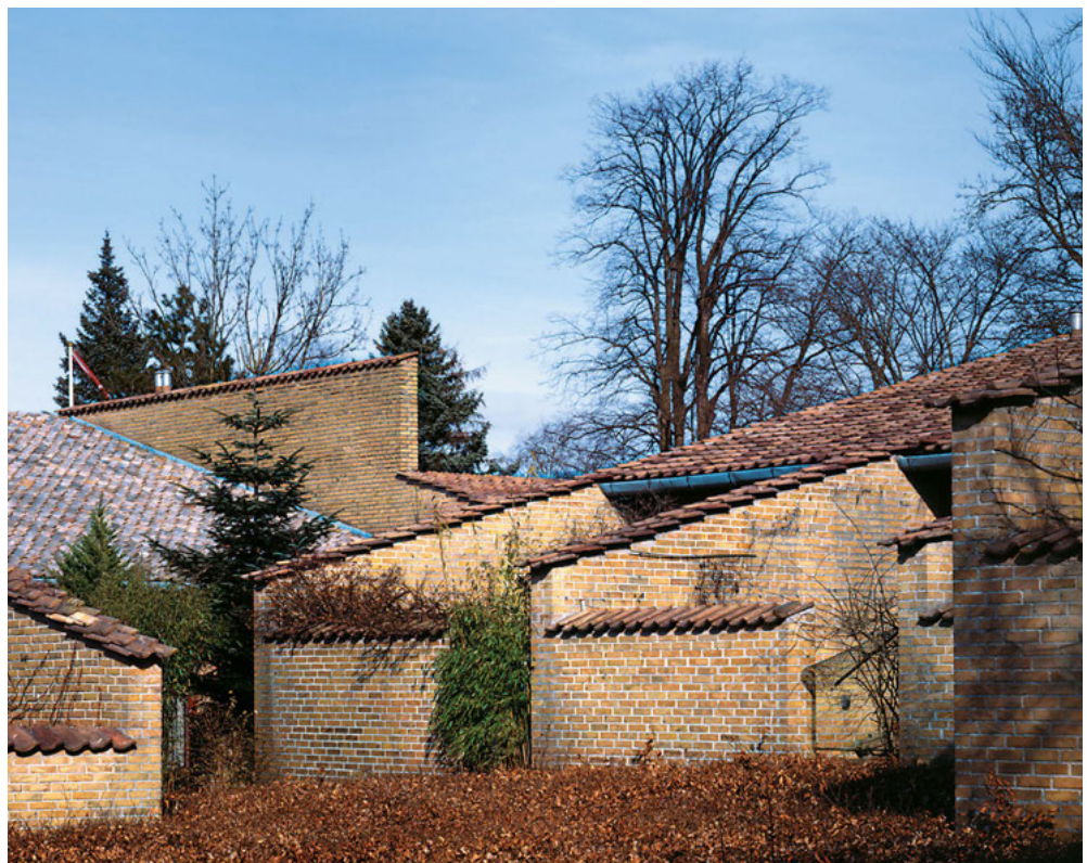
View of roofs
