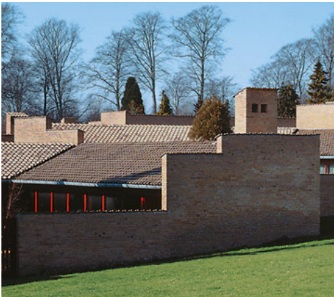
View of roofs
