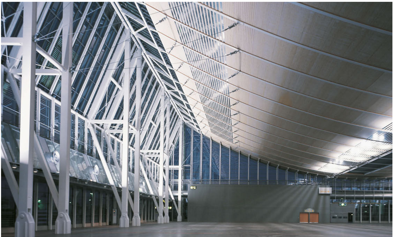
Interior/underside of roof
