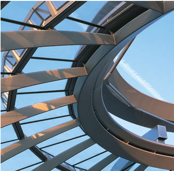
Apex of dome with ring girder and wind-deflecting profile
