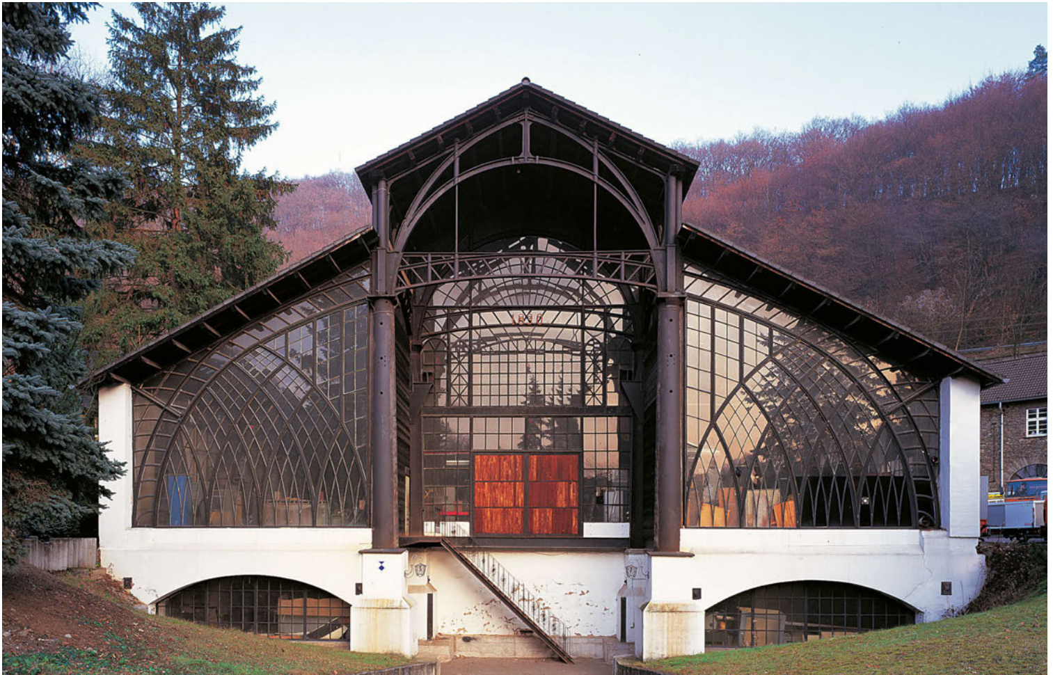
1.1 Foundry building, Sayner Works, Bendorf, 1828-30, Carl Ludwig Althans
