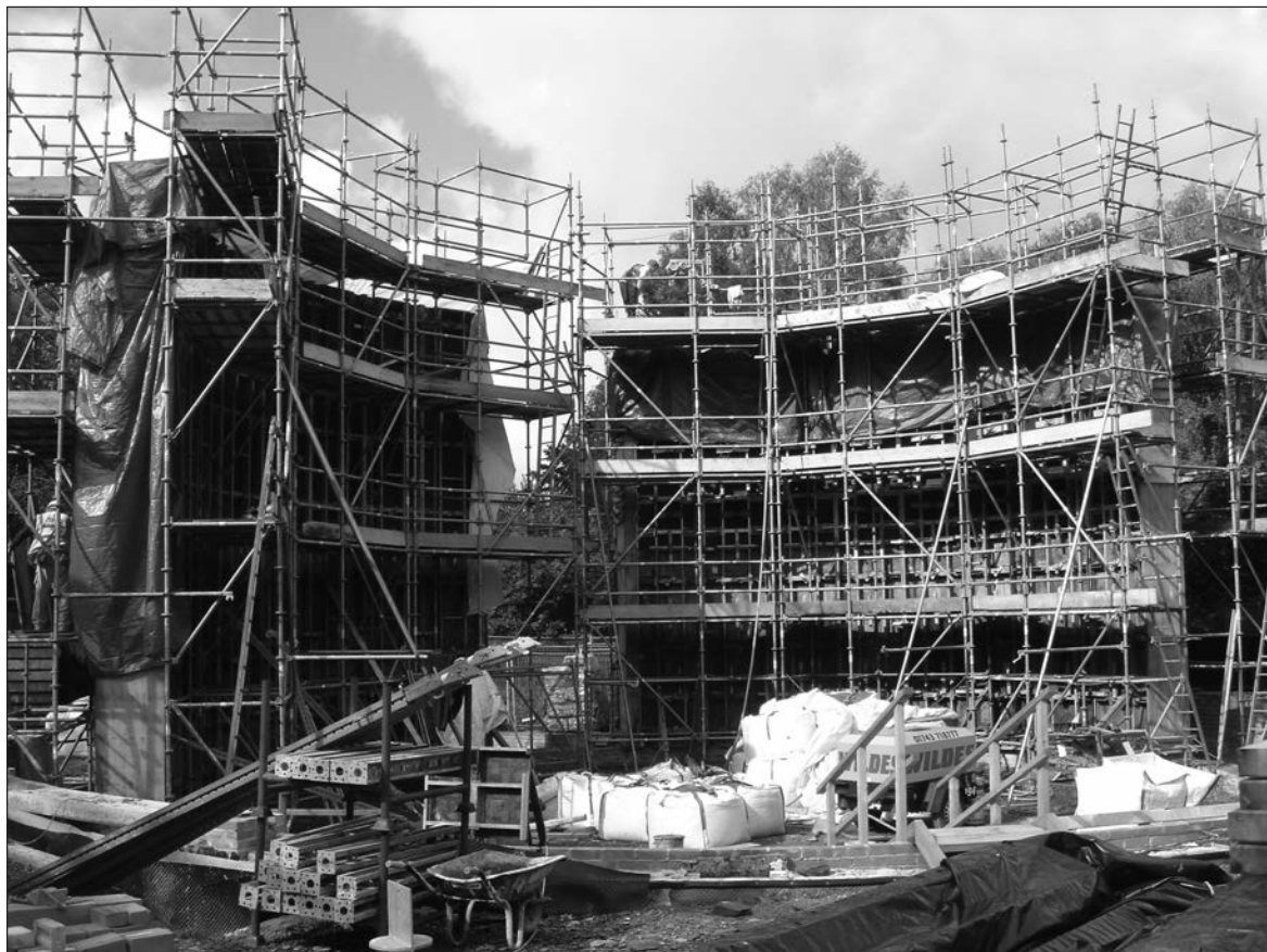
WISE building under construction
