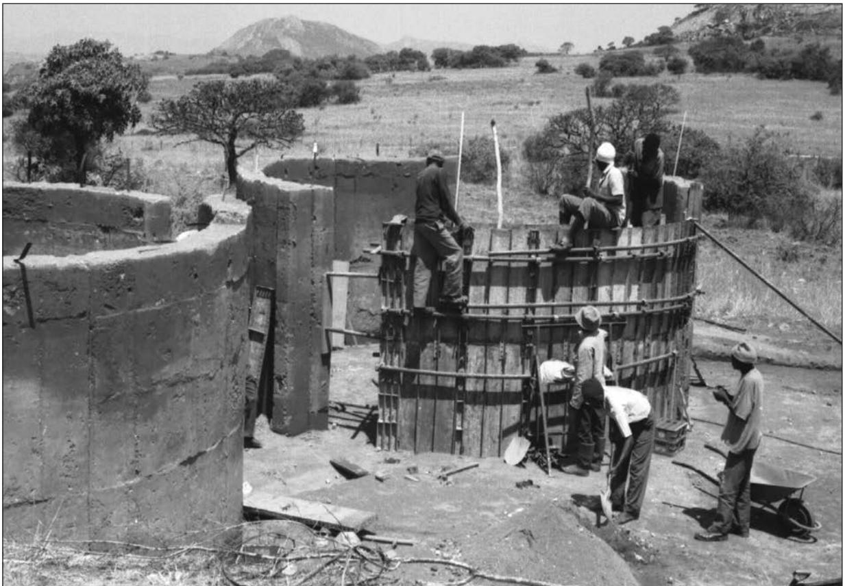
Bonda house under construction
