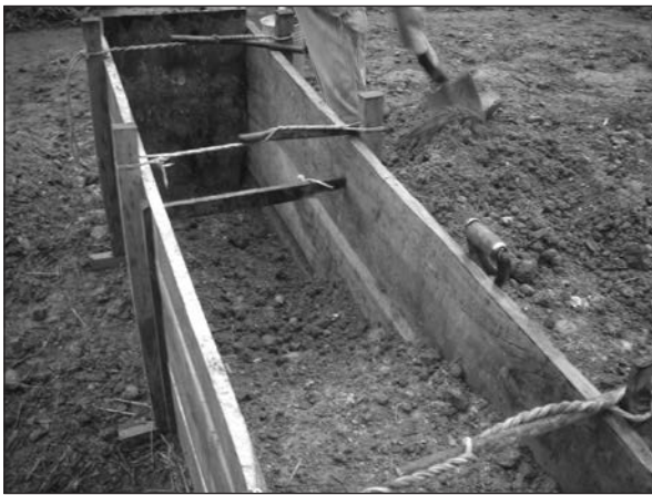
(8) Second fill jointing on to sloping face
