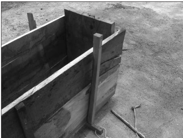
(2) Placing vertical ribs into bottom blot slots
