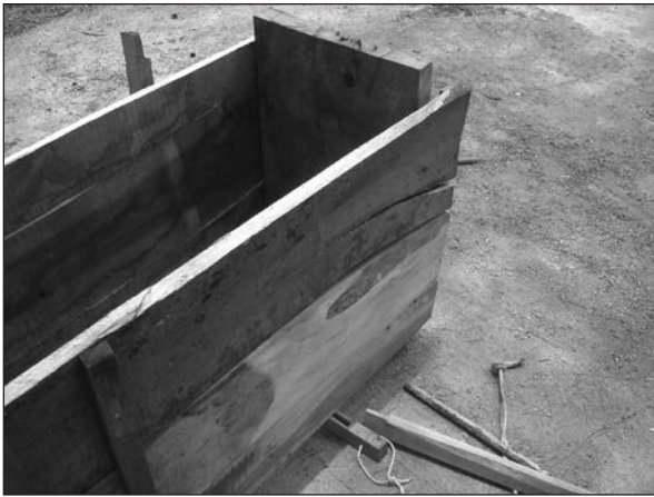
(1) Bottom bolts showing slots for vertical ribs
